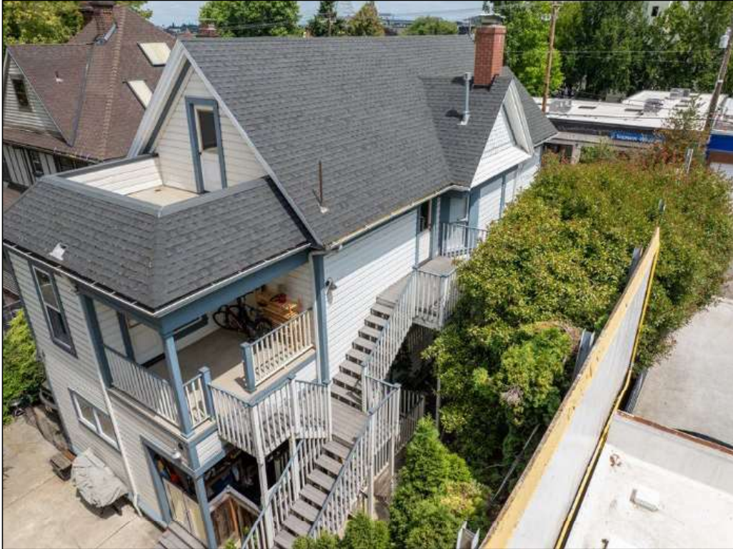
Photograph 5 of 16: OR_MultnomahCounty_DeversArthurHHouse_0005 Looking northeast at southwest corner from back yard.
