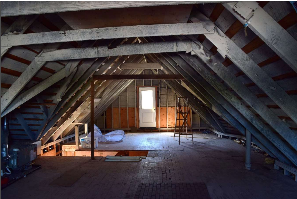
Photograph 16 of 16: OR_MultnomahCounty_DeversArthurHHouse_0016 Interior, looking west at the attic level.
