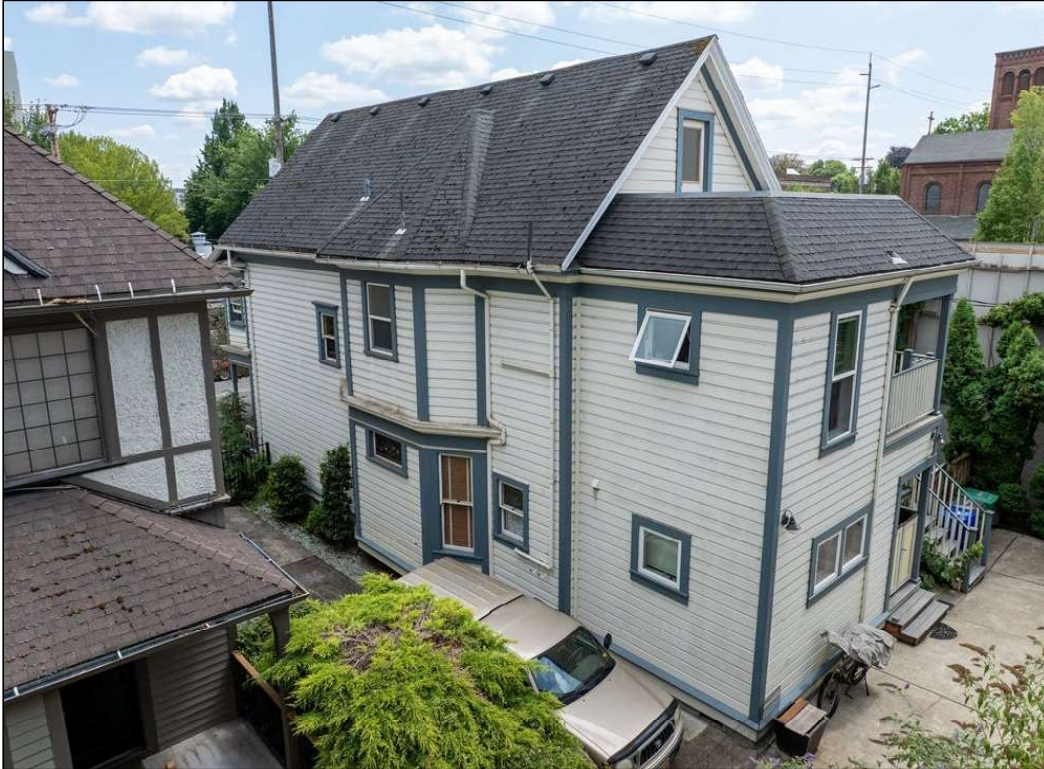
Photograph 3 of 16: OR_MultnomahCounty_DeversArthurHHouse_0003 Looking southeast at the north and west façades.
