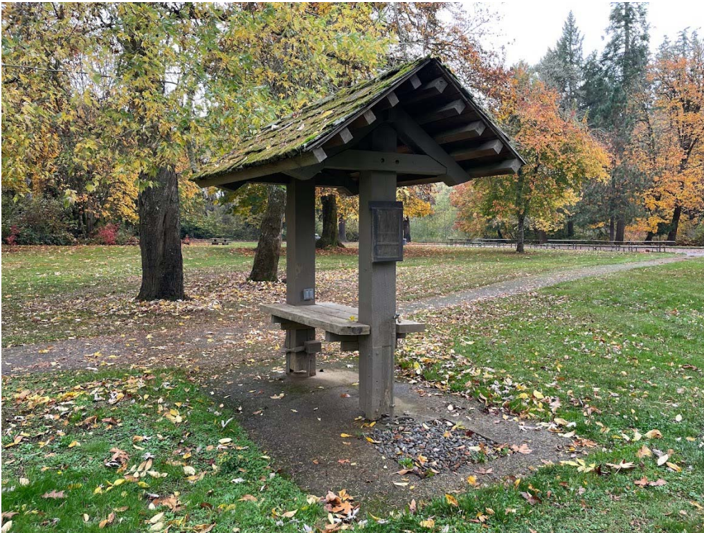
Photo 13 of 19: Stove shelter (1 of 2). Looking west/northwest.
