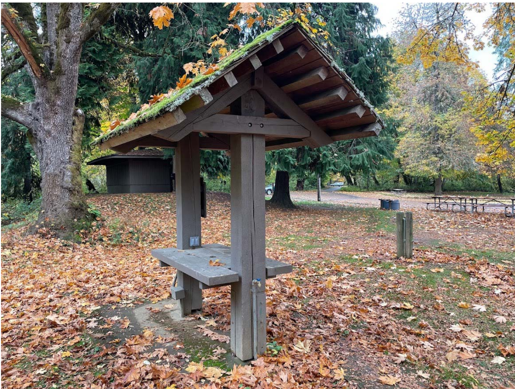
Photo 14 of 19: Stove shelter (2 of 2). Looking north/northeast.
