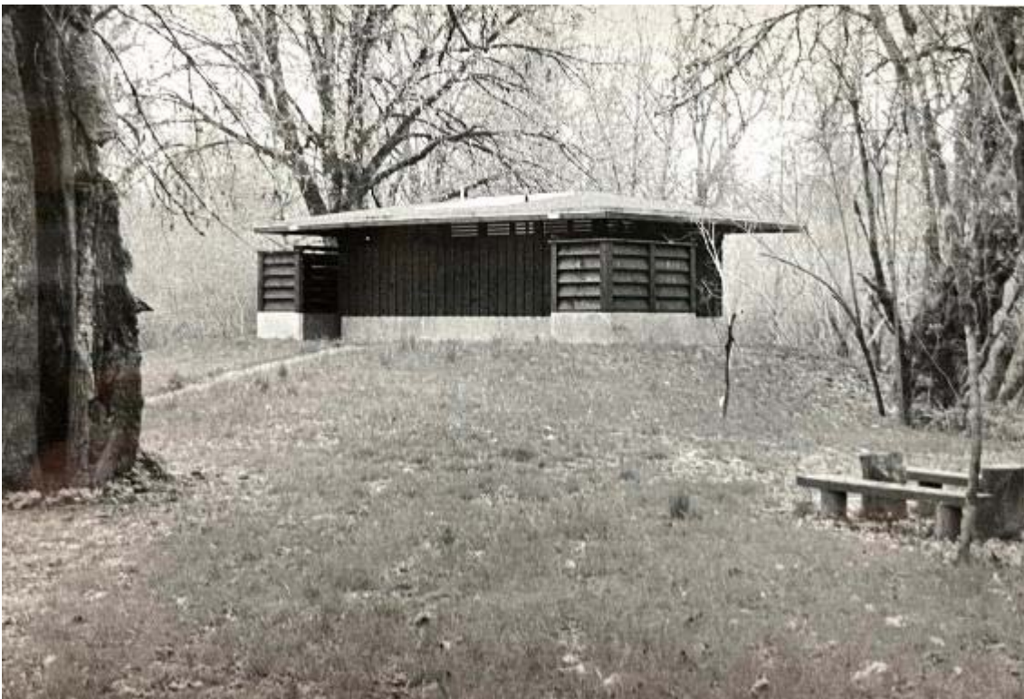
Figure 17: HISTORIC PHOTO West latrine, March 1957. Oregon Parks and Recreation Department Archives. Sarah Helmick State Park Folder.
