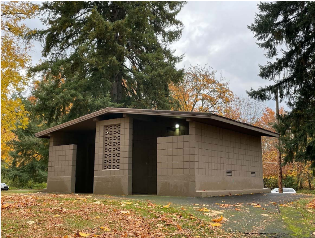
Photo 17 of 19: East latrine. Looking northeast.
