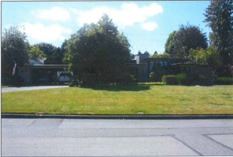
Photo 1 of 18: OR_MultnomahCounty_AmundsenHouse_0001 East façade (primary) camera facing west.
