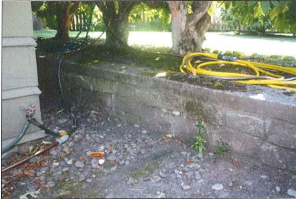
Photo 8 of 18: OR_MultnomahCounty_AmundsenHouse_0008 Detail: Stone wall west of house. North façade (left). Camera facing southwest.
