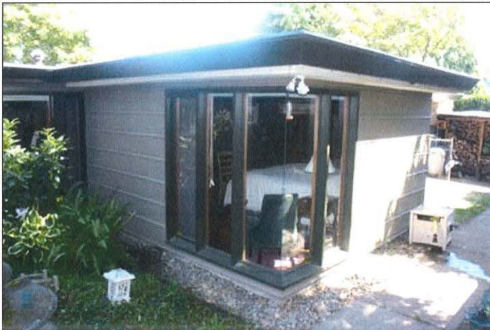
Photo 7 of 18: OR_MultnomahCounty_AmundsenHouse_0007 Southwest projection windows of Bedroom 3. West façade (right) north façade (left). Camera facing southeast.
