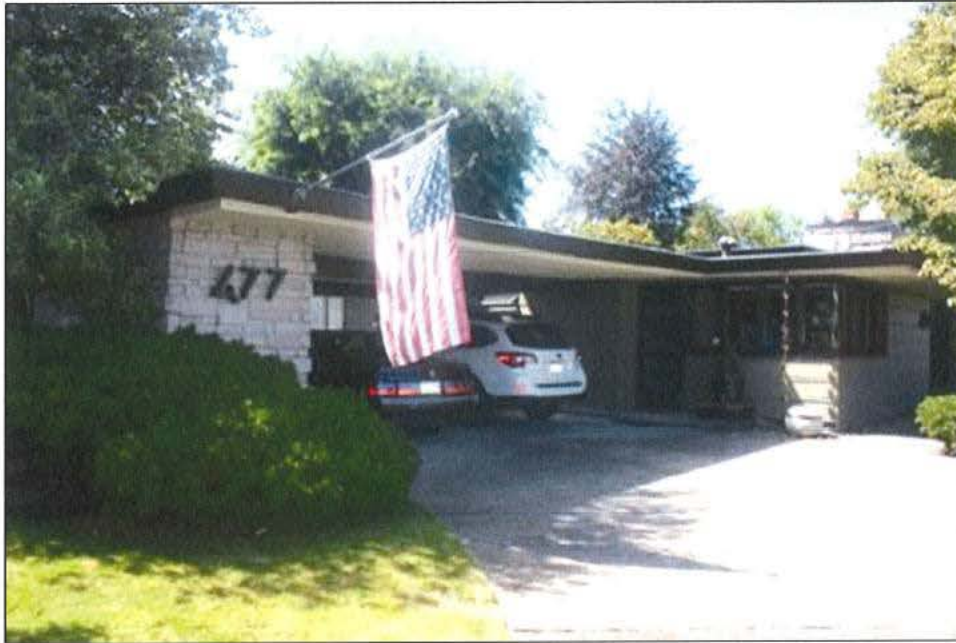
Photo 3 of 18: OR_MultnomahCounty_AmundsenHouse_0003 South façade (right) and carport (left), camera facing northwest.
