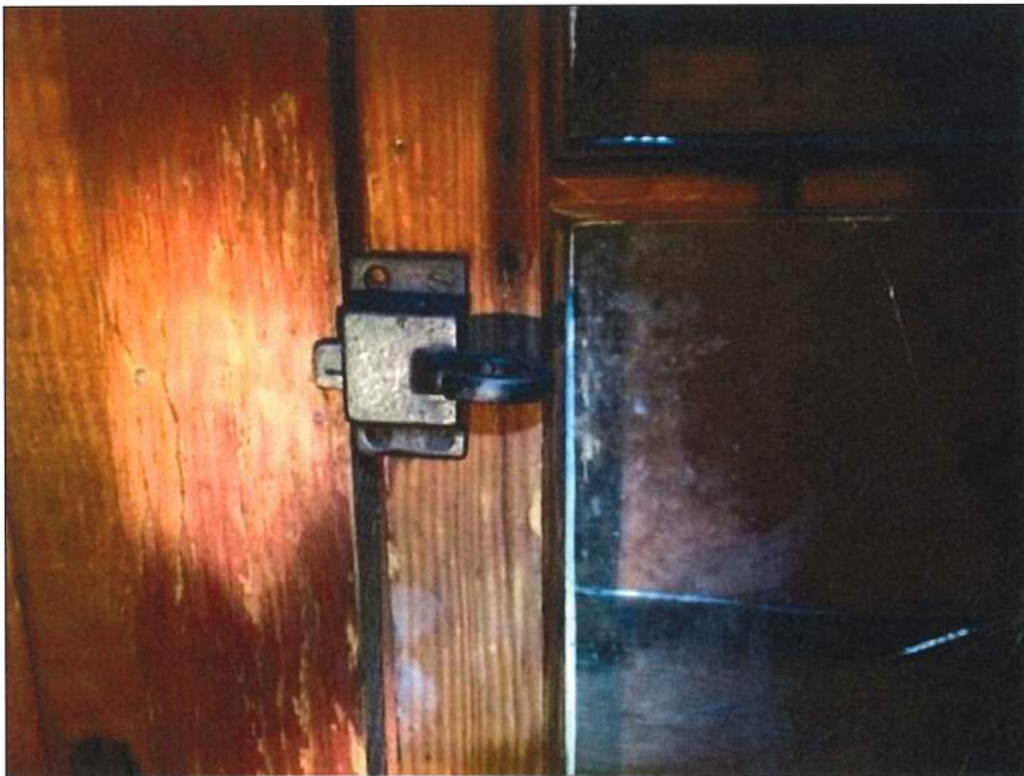
Photo 6 of 10: Main Lodge window hardware, example of type on all windows
