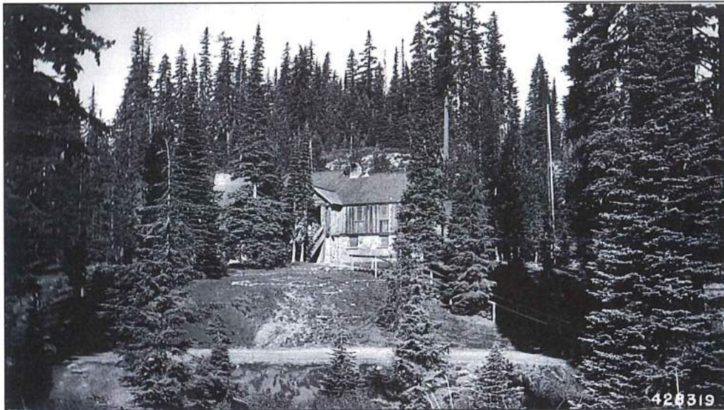
Figure 10: Santiam Pass Ski Lodge c.1940 Same film as Figure 11 but different exposure.
