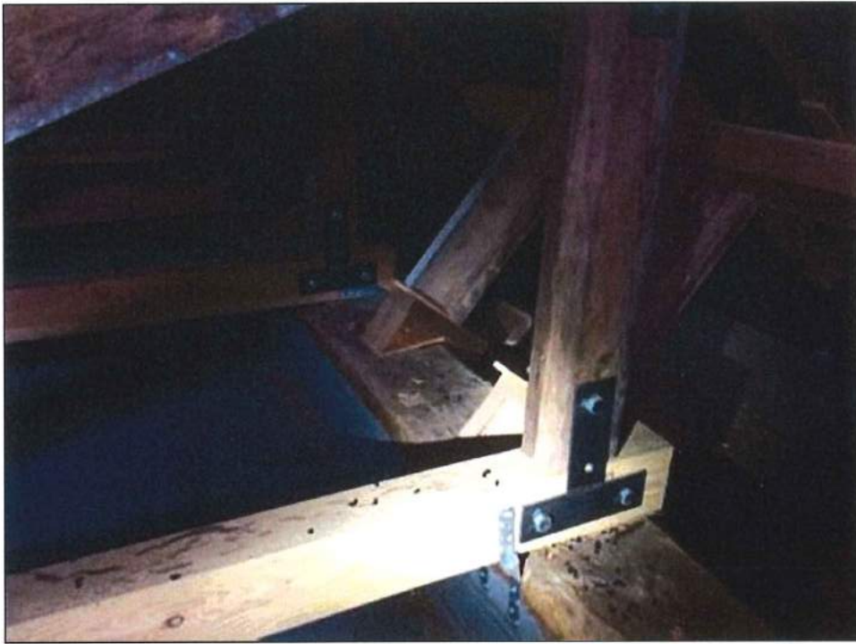
Photo 5 of 10: Main Lodge interior attic story 2003 structural reinforcements
