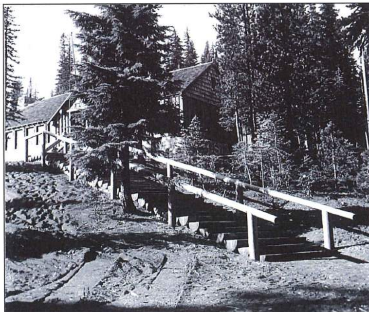
Figure 13: Santiam Ski Lodge 1941. Of half round log stairs. Southeast facing aspect of the lodge in the background.
