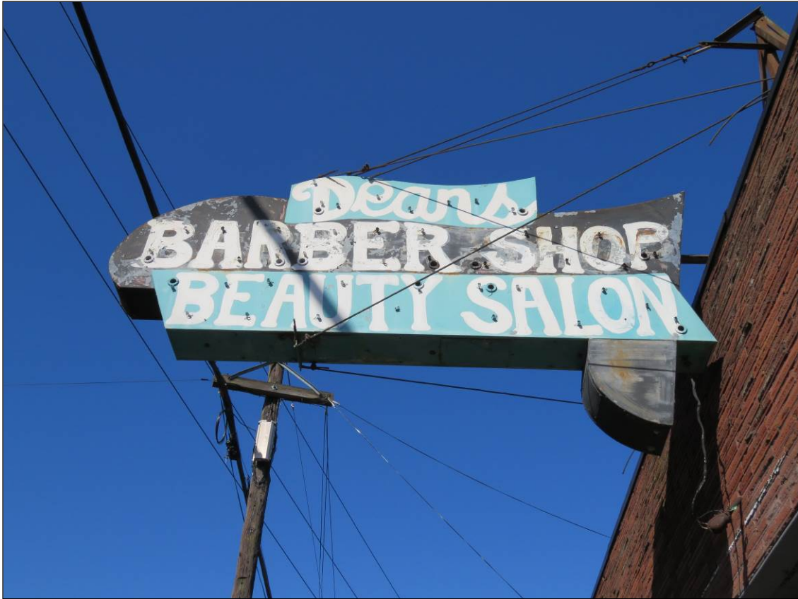
Photograph 7 of 22: OR_MultnomahCounty_DeansBeautySalonandBarberShop_0007 Detail of original blade sign extending over primary (south) façade, camera facing west.
