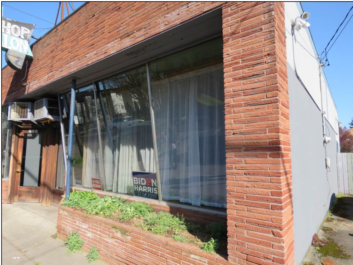
Photograph 6 of 22: OR_MultnomahCounty_DeansBeautySalonandBarberShop_0006 Detail of angled window and integral planter in primary (south) façade, camera facing north.
