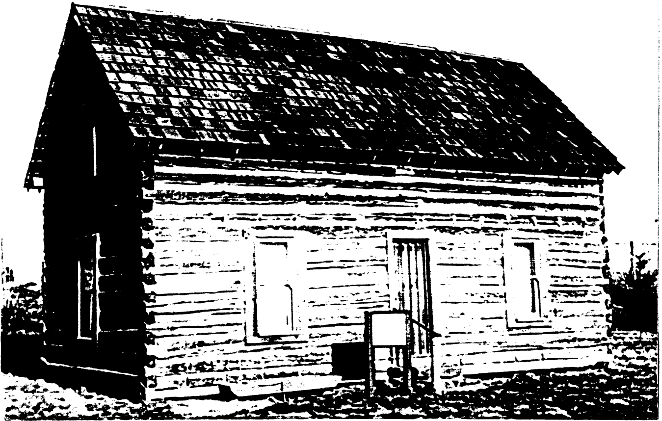
South (front) elevation as restored. Jean Gilliam photograph, February 25, 1991. Present site on Gilliam County Fairgrounds, Burns Park at Condon.
