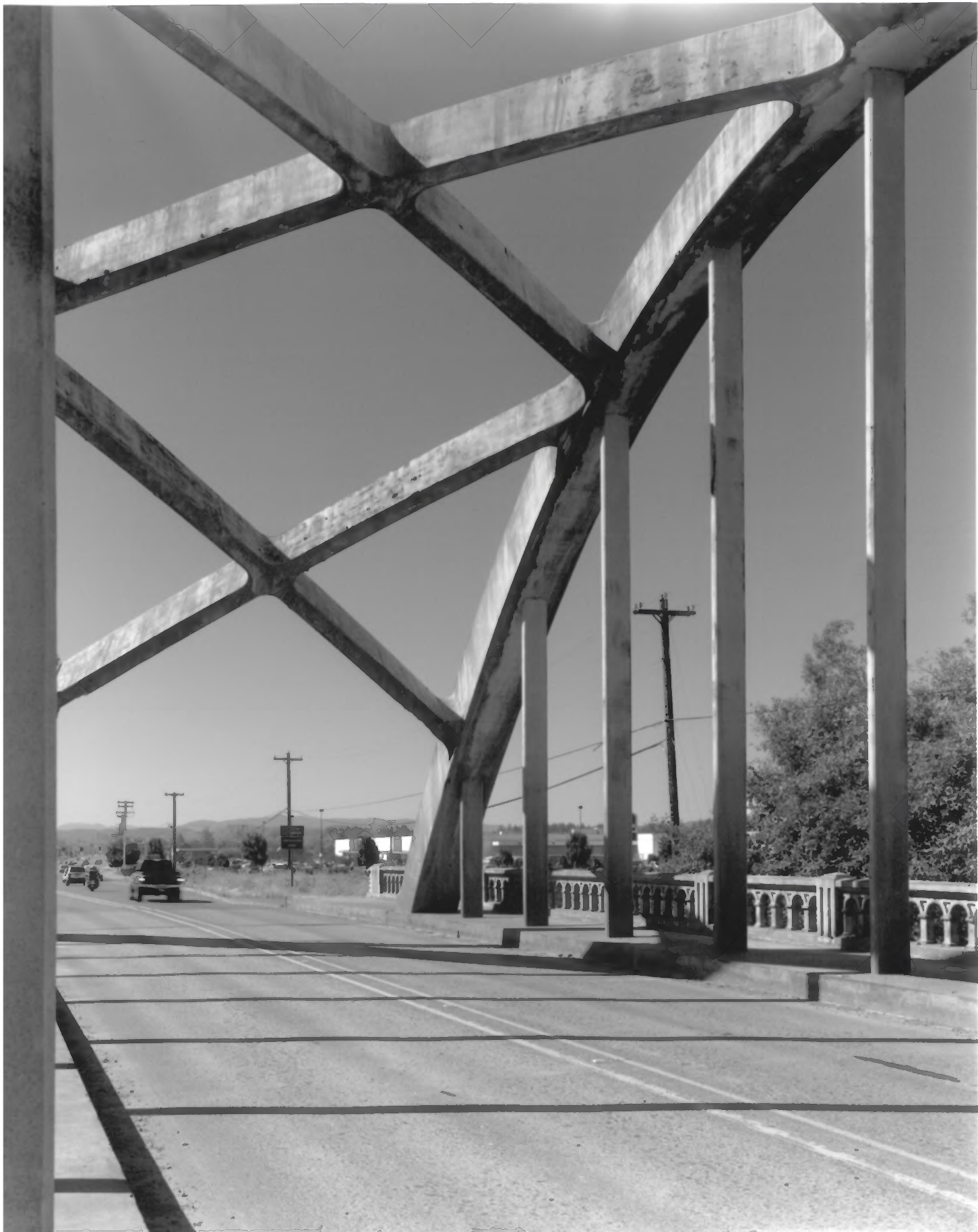
WILSON RIVER BRIDGE, TILLAMOOK, OREGON # 9
