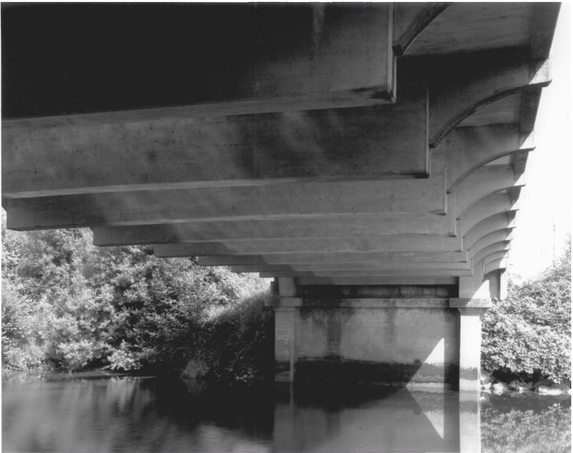
WILSON RIVER BRIDGE, TILLAMOOK, OREGON
