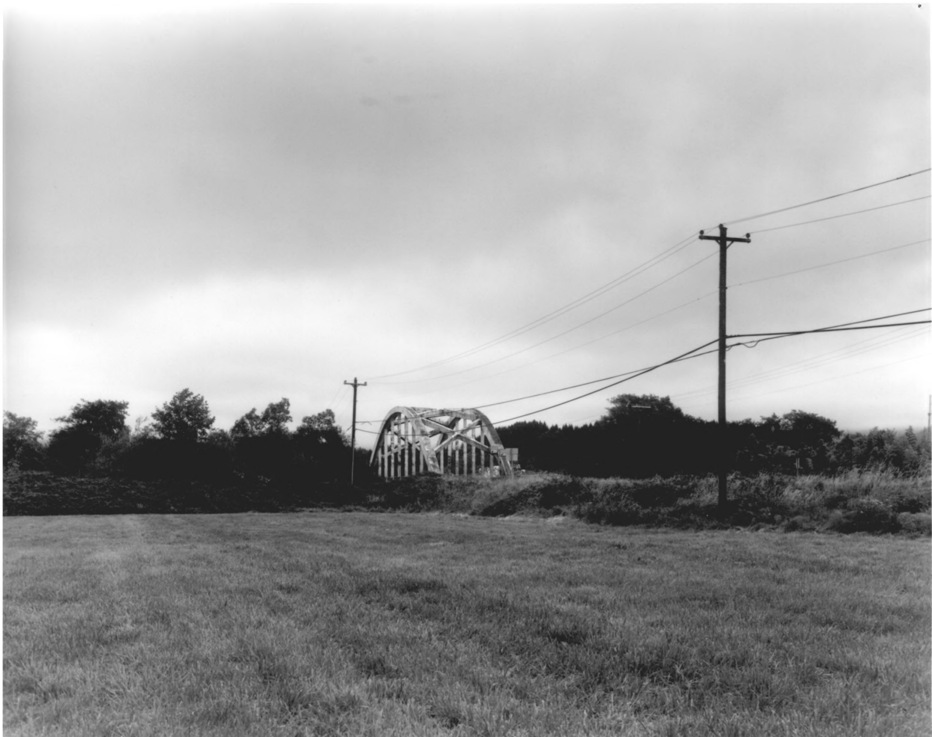
WILSON RIVER BRIDGE, TILLAMOOK, OREGON #1
