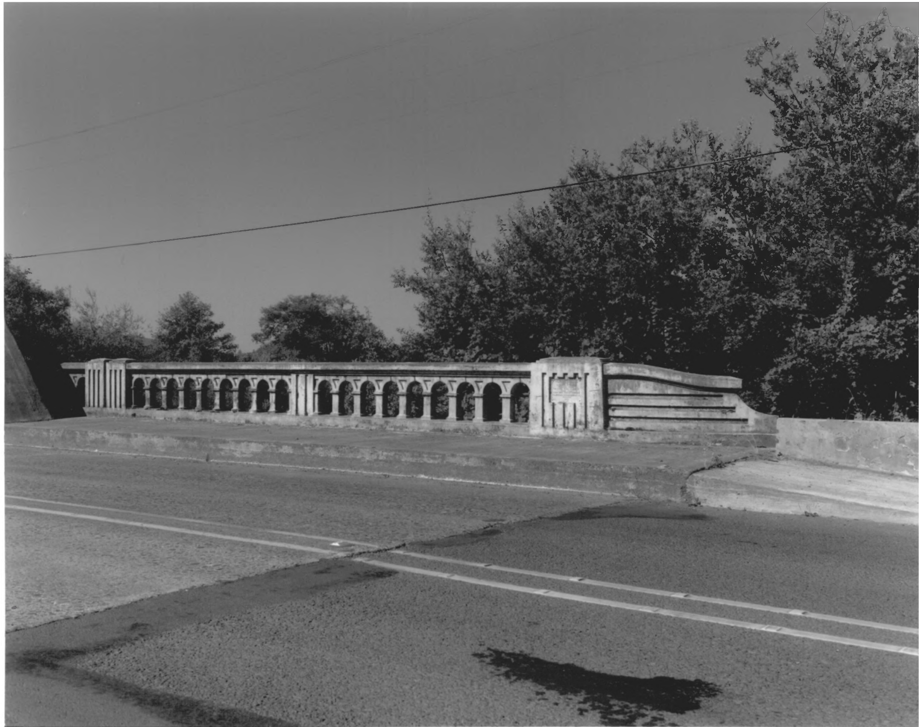
WILSON RIVER BRIDGE, TILLAMOOK, OREGON
