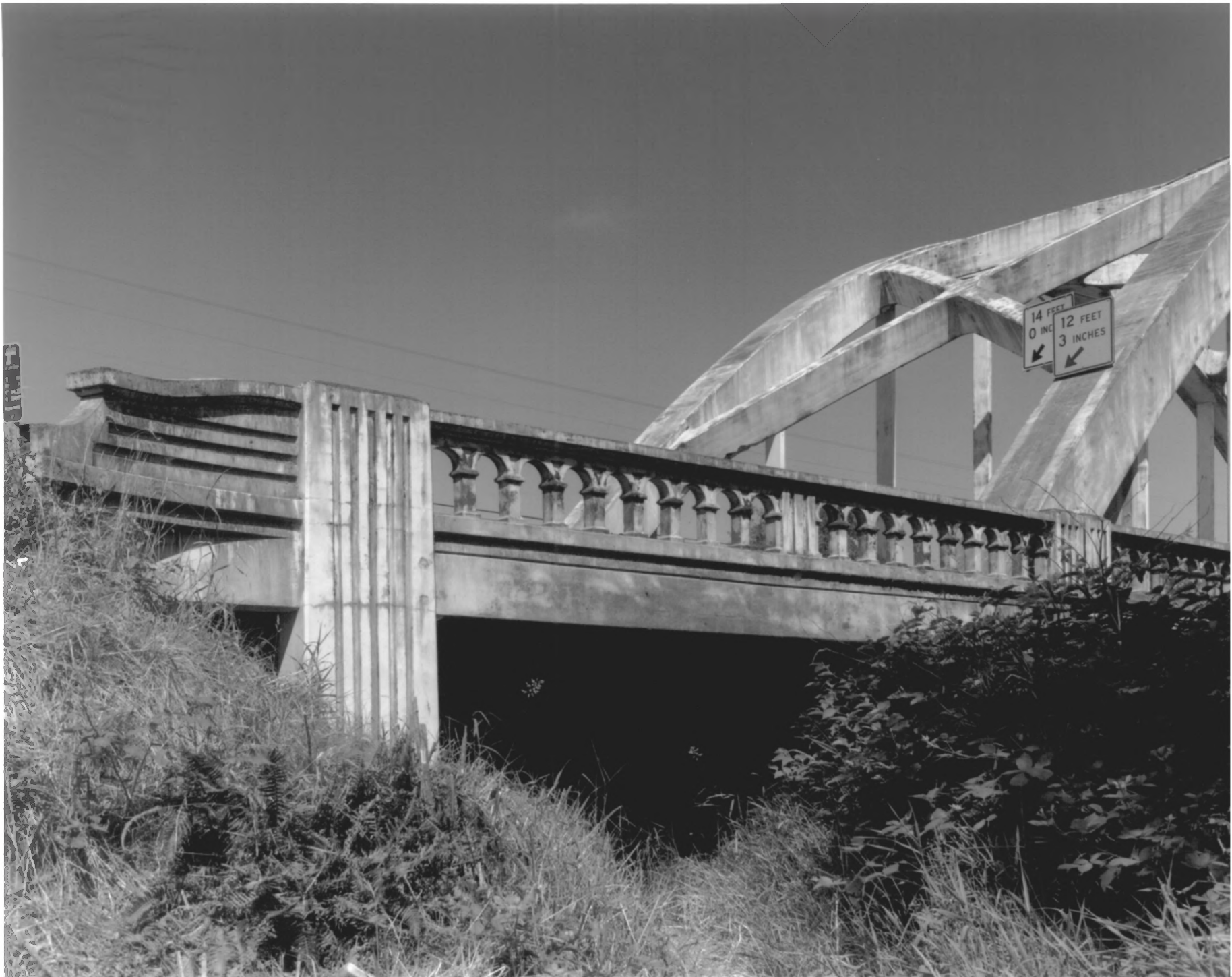
WILSON RIVER BRIDGE, TILLAMOOK, OREGON
