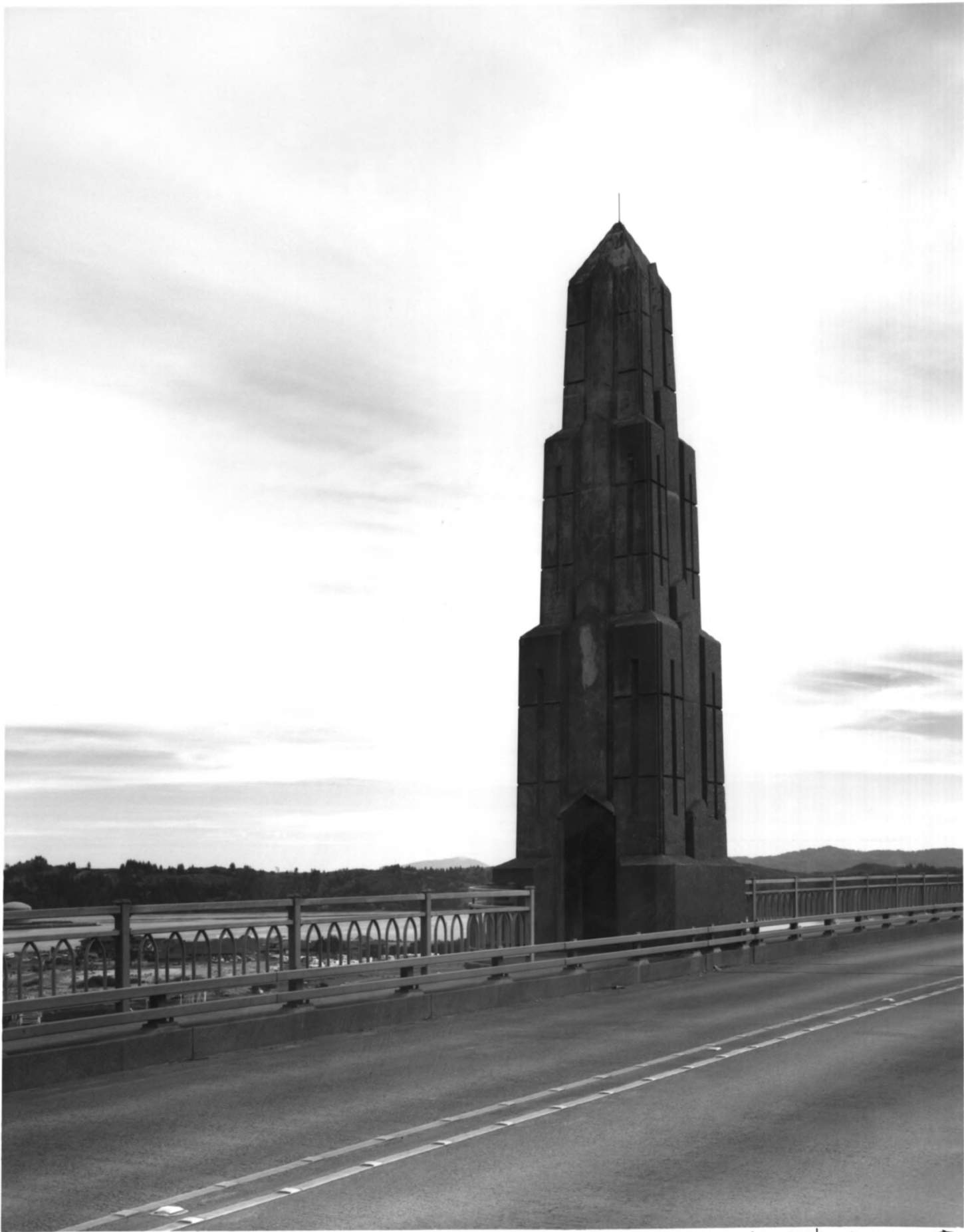
YAVINA BAY BRIDGE, NEWPORT, OREGON # 11
