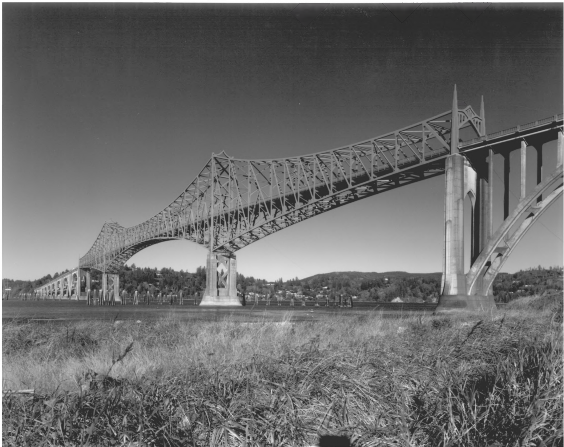
COOS BAY BRIDGE, COOS BAY, OREGON
