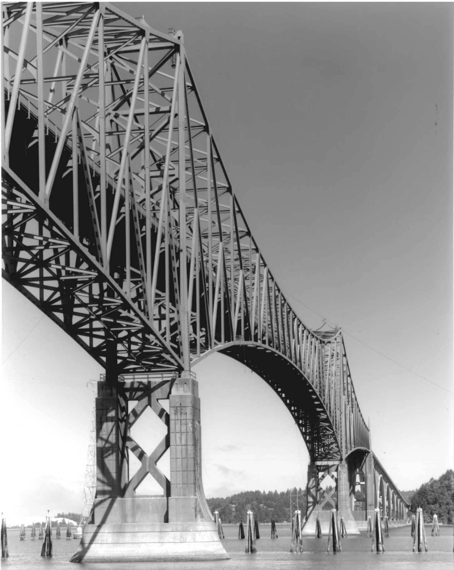
COOS BAY BRIDGE, COOS BAY, OREGON #8
