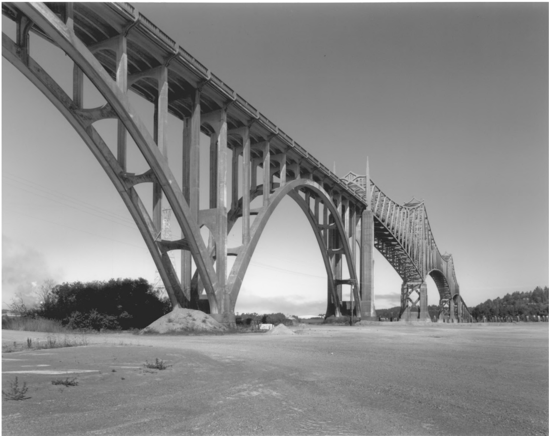
COOS BAY BRIDGE, COOS BAY, OREGON
