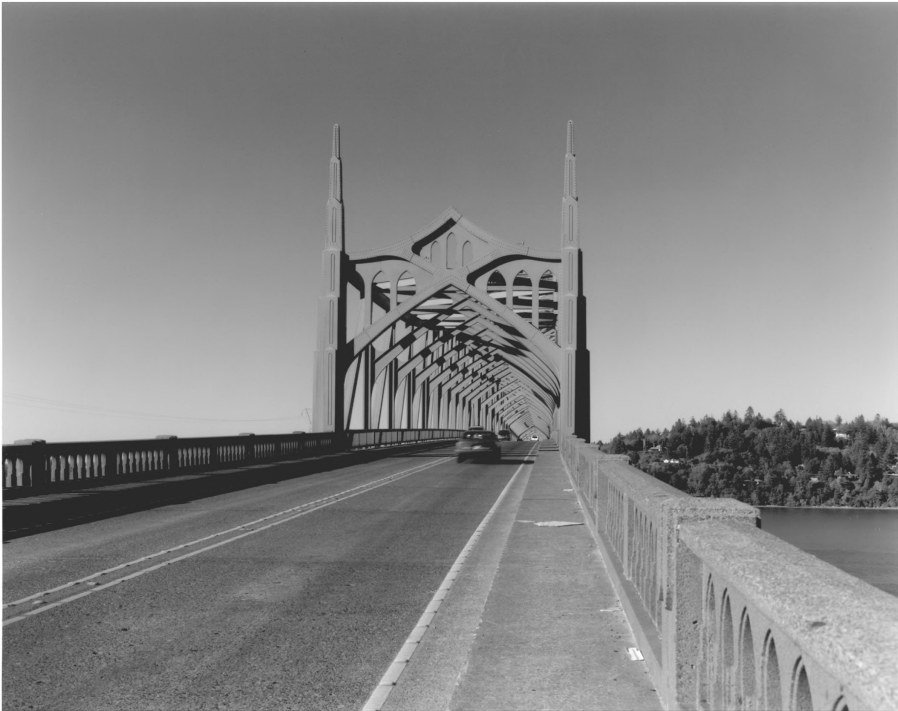
COOS BAY BRIDGE, COOS BAY, OREGON #9
