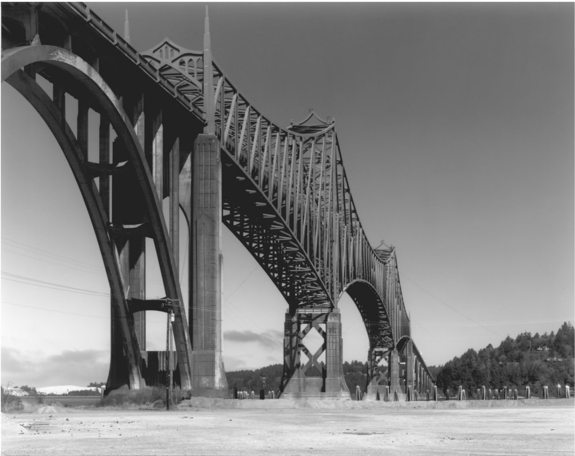
COOS BAY BRIDGE, COOS BAY, OREGON
