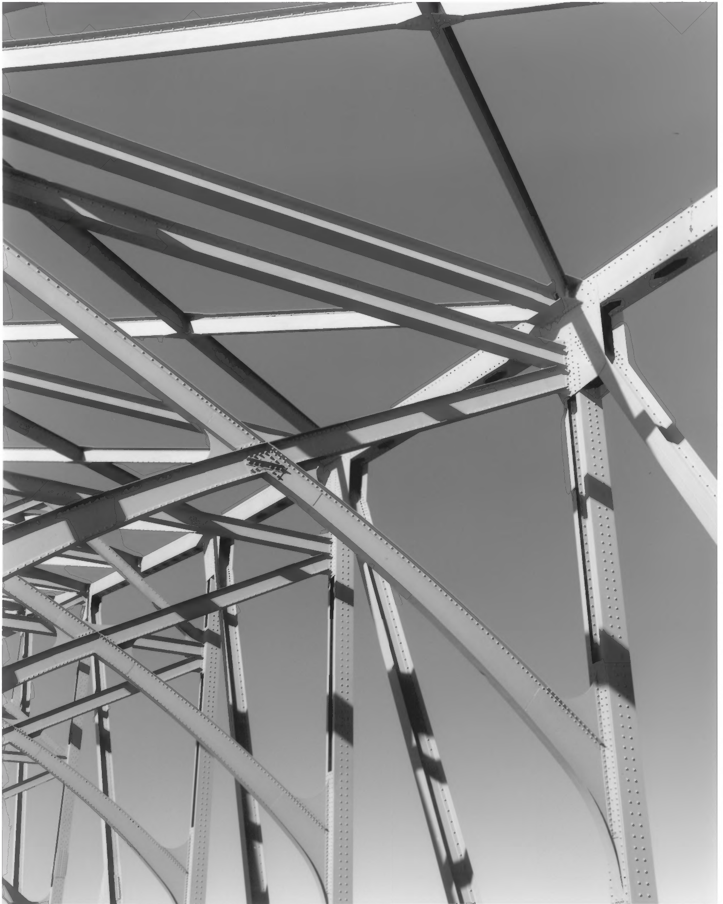
COOS BAY BRIDGE, COOS BAY, OREGON # 11
