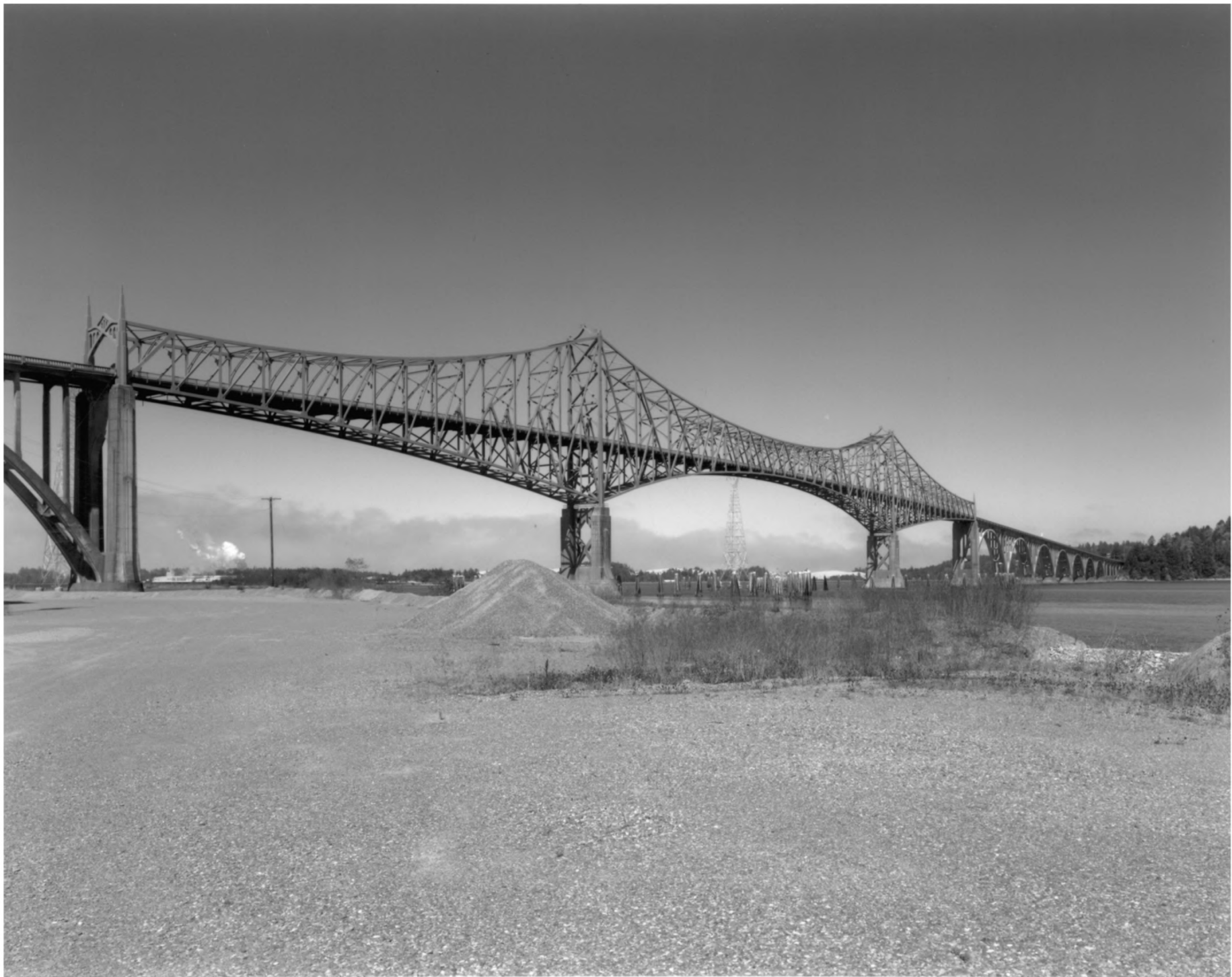
COOS BAY BRIDGE, COOS BAY, OREGON #2
