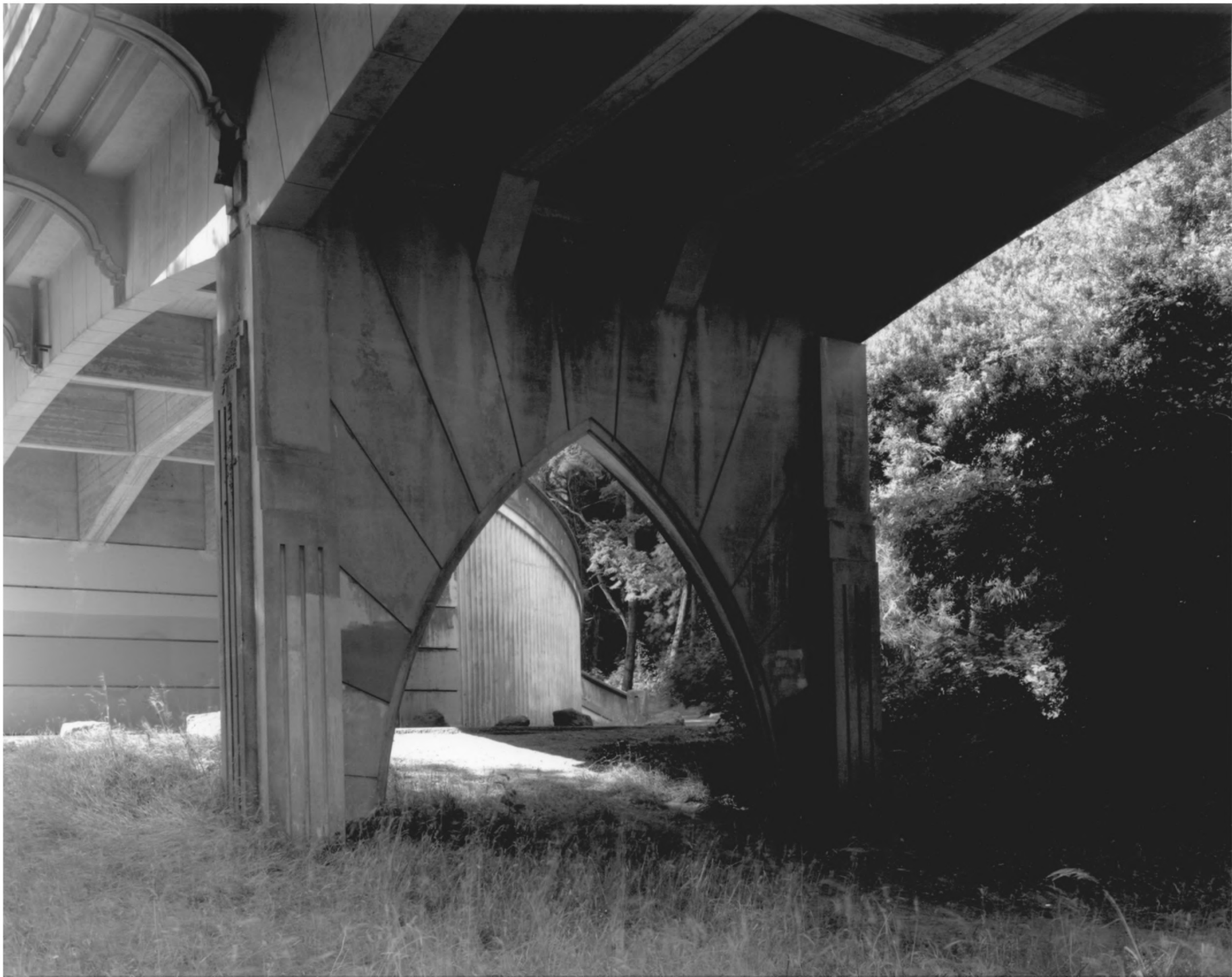
COOS BAY BRIDGE, COOS BAY, OREGON
