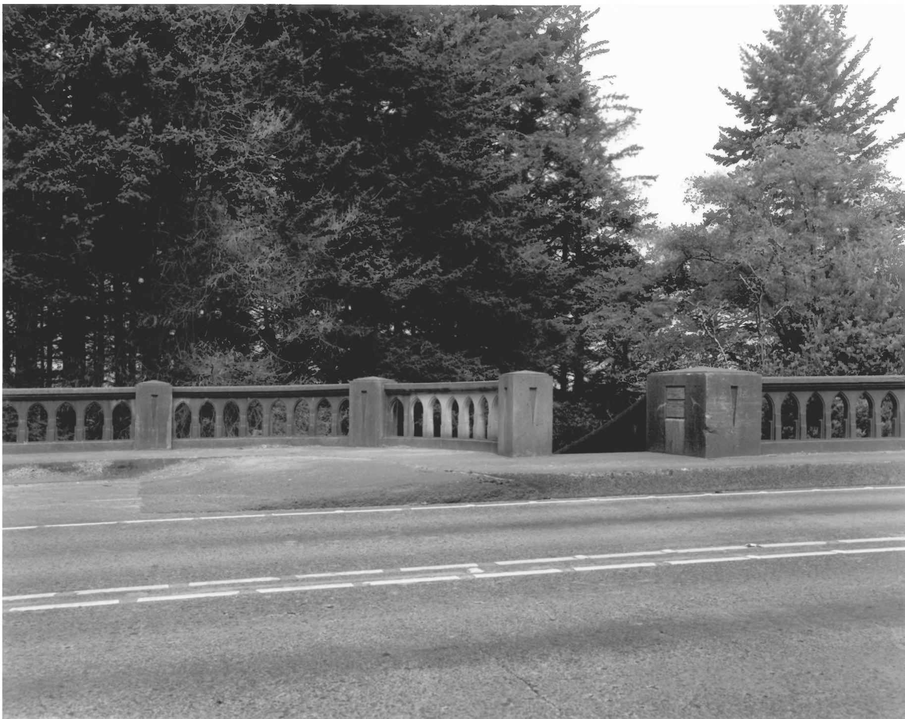
COOS BAY BRIDGE, COOS BAY, OREGON
