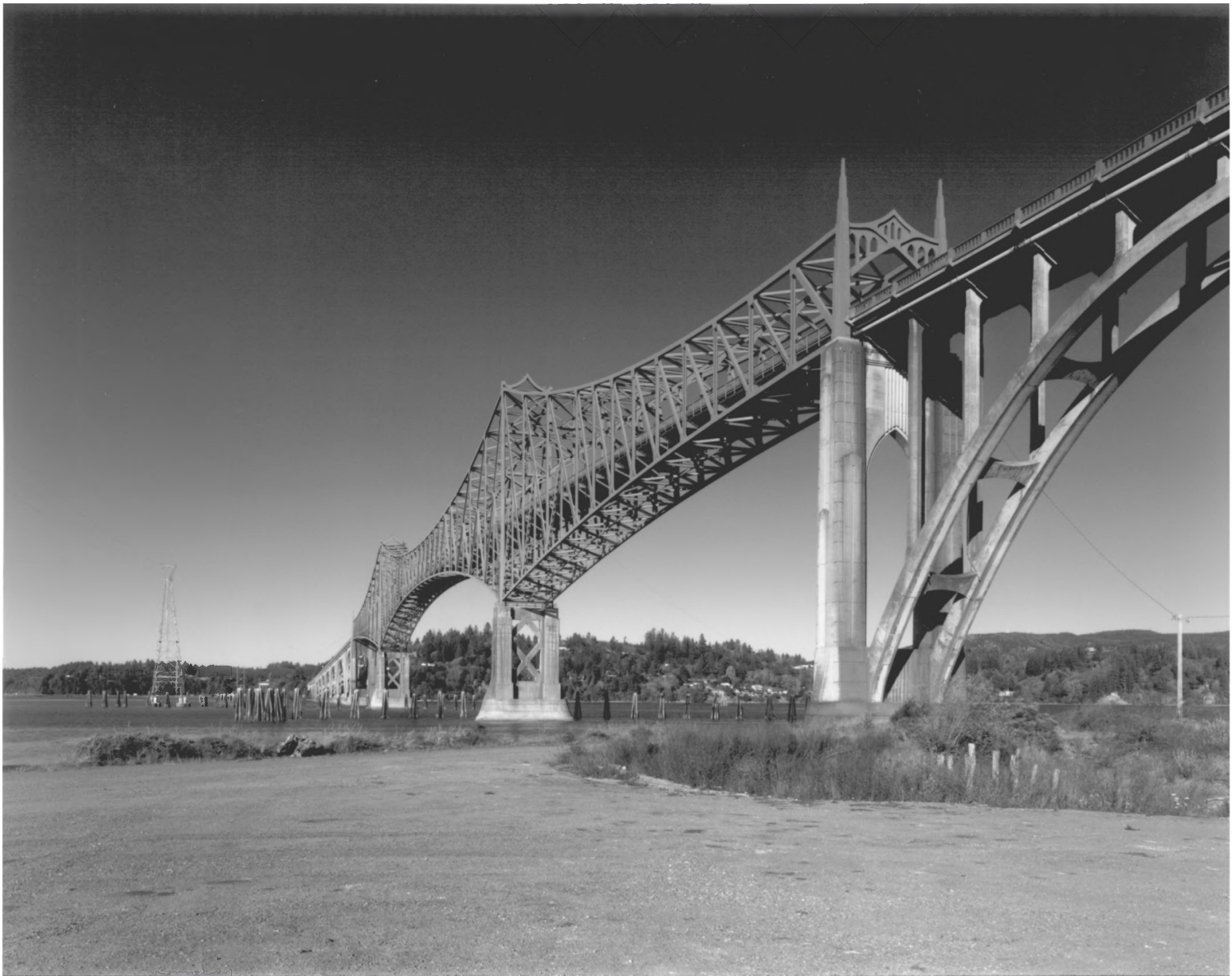
COOS BAY BRIDGE, COOS BAY, OREGON #16
