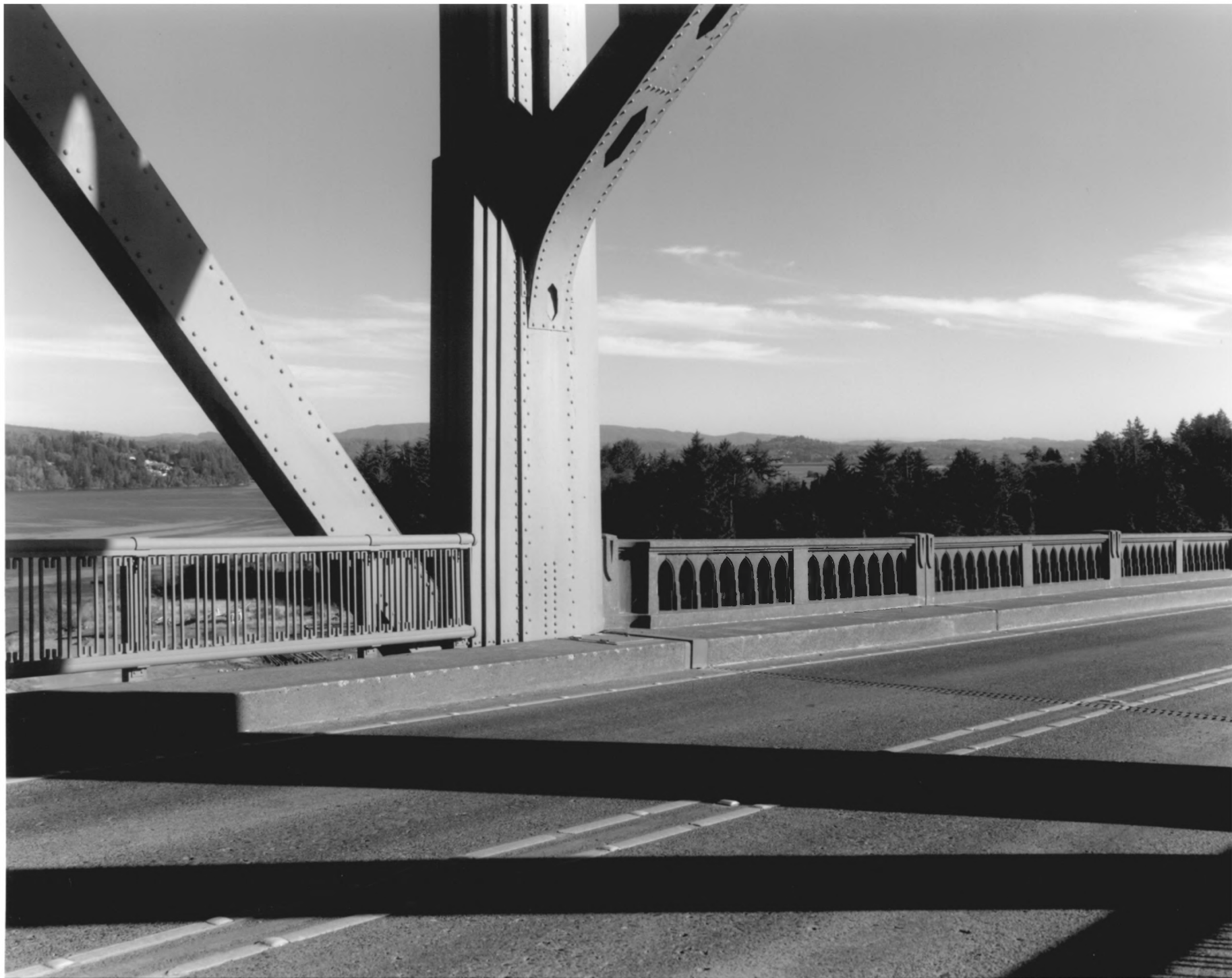
COOS BAY BRIDGE, COOS BAY, OREGON #10
