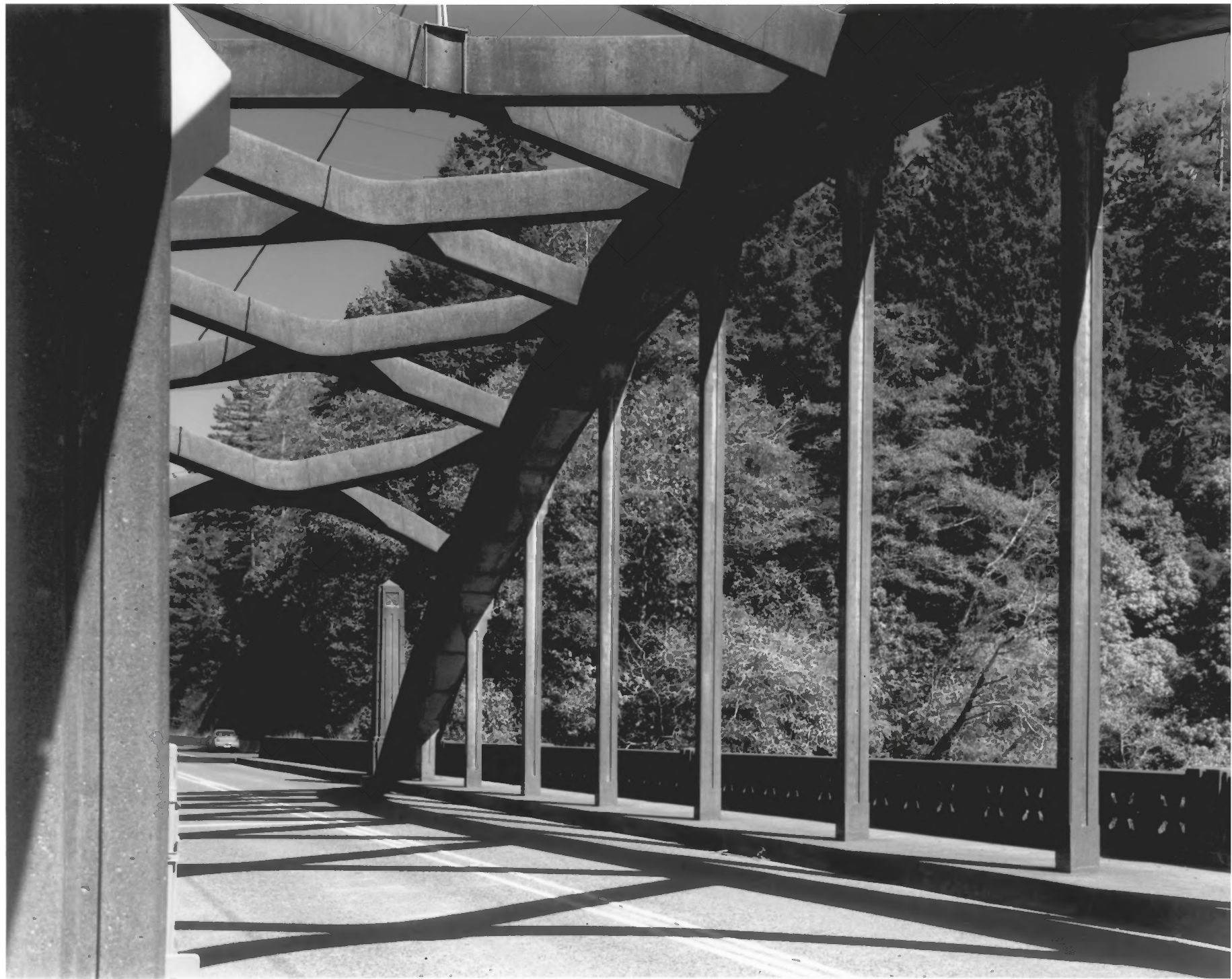
UMPUWA RIVER BRIDGE RECONSTRUCTION #9
