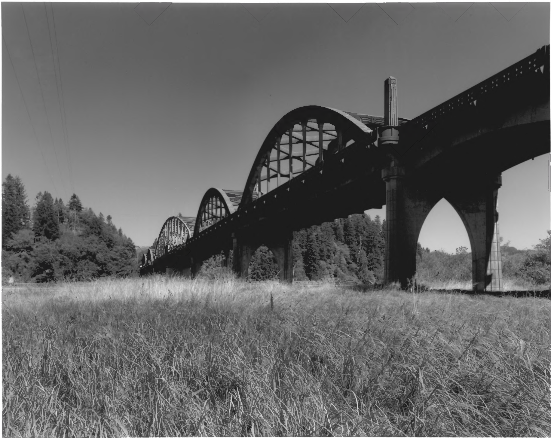
UMPUQA RIVER BRIDGE, REEDSPORT, OREGON #3
