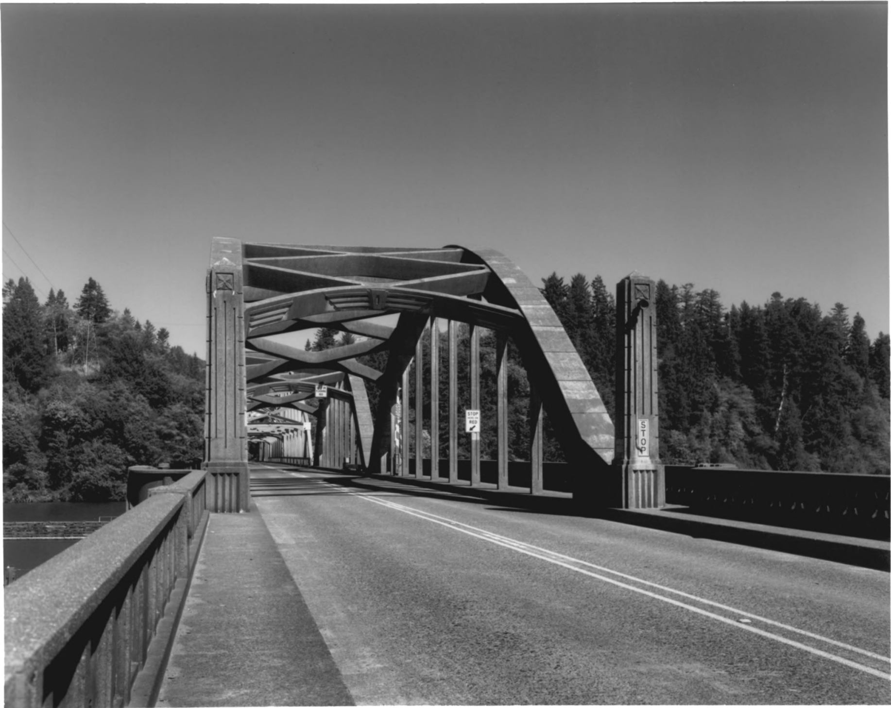
UMPUQA RIVER BRIDGE, REEDSPORT, OREGON
