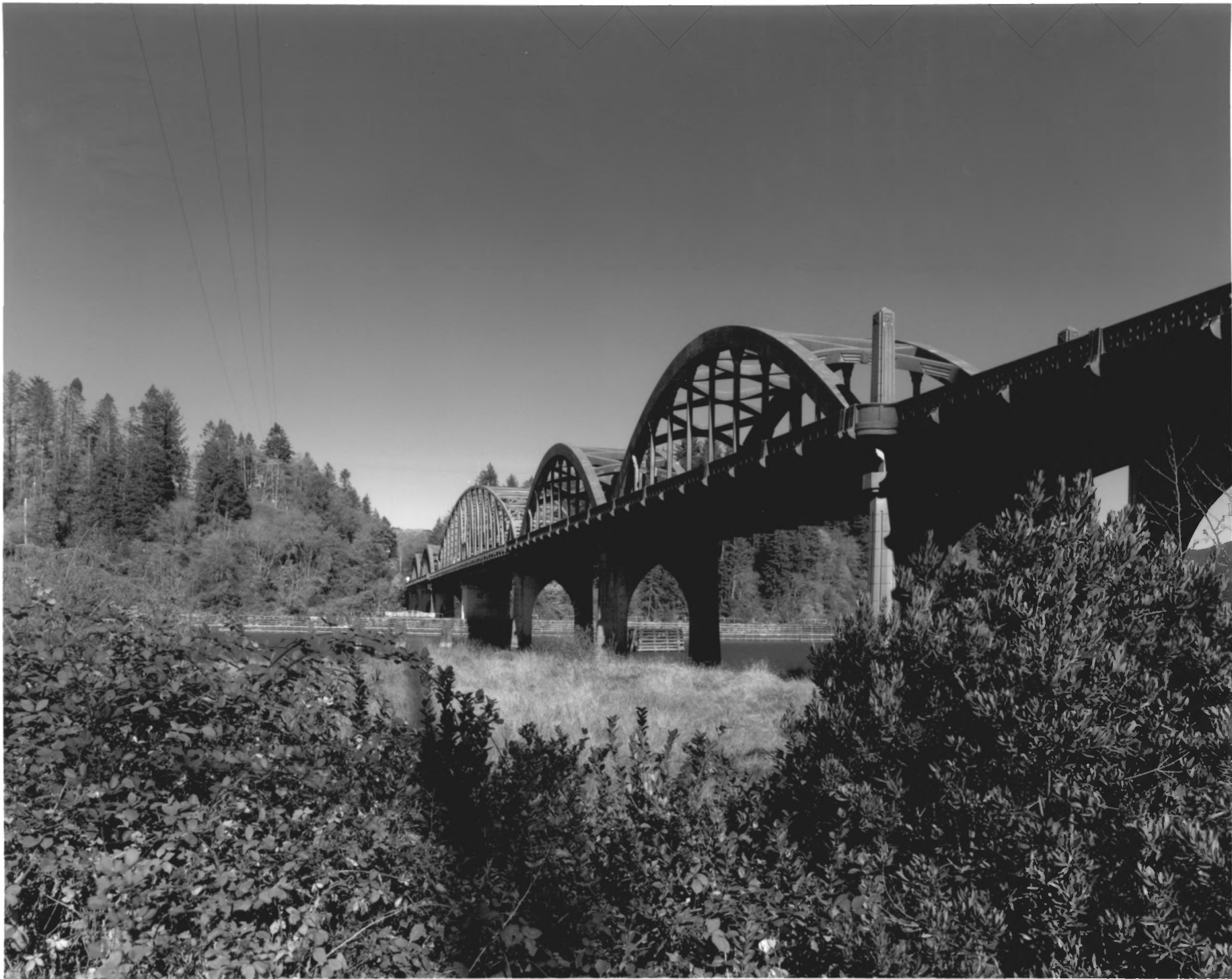
WAPOVA RIVER BRIDGE, REEDSPORT, OREGON
