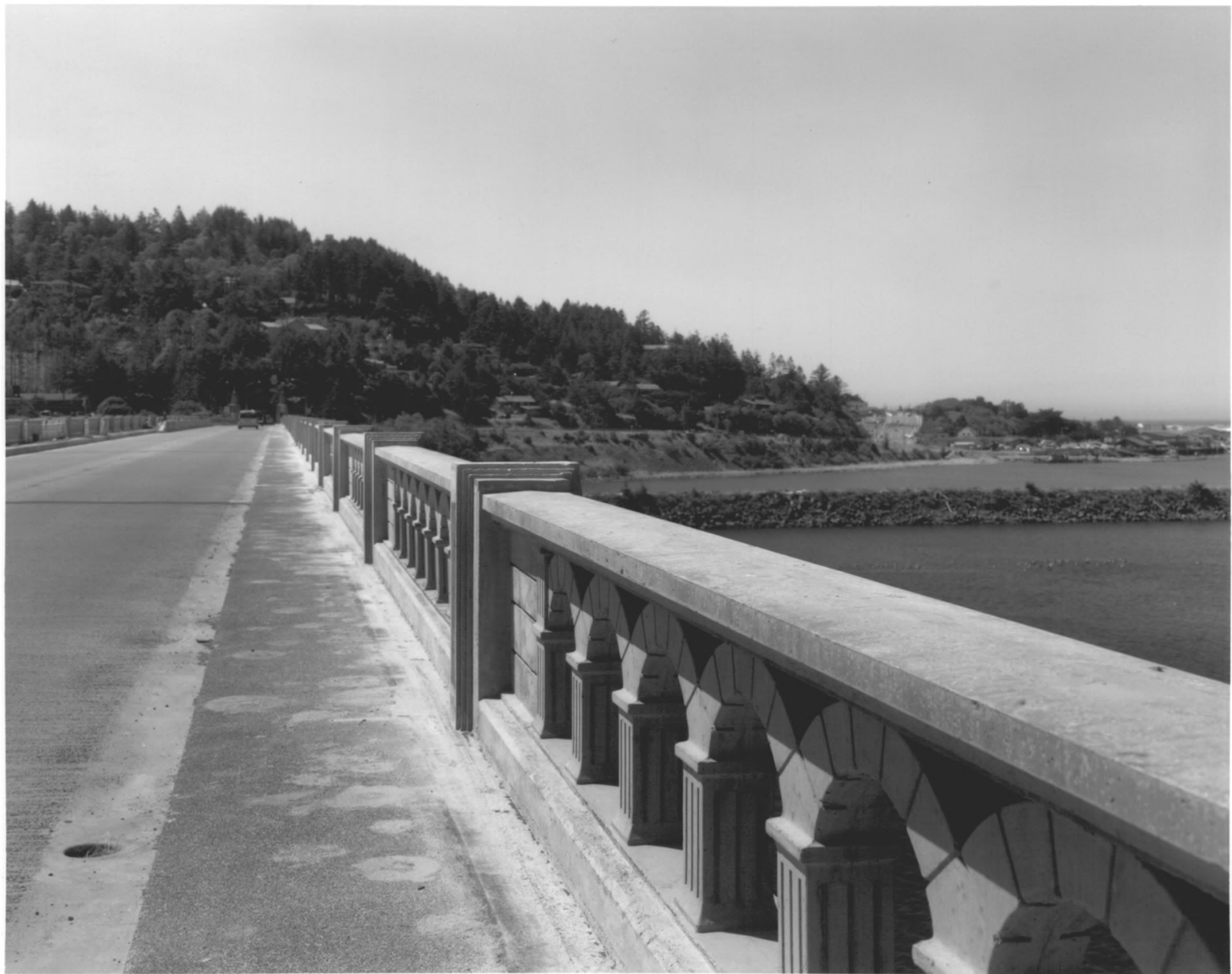
ROGUE RIVER BRIDGE, GOLD BEACH, OREGON
