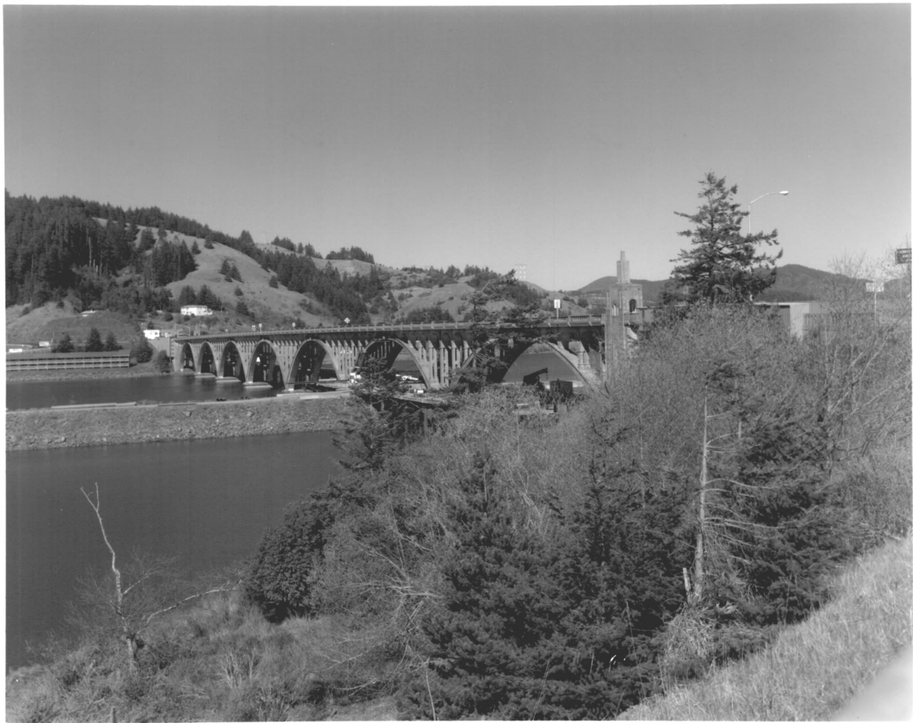
ROGUE RIVER BRIDGE, GOLD BEACH, OREGON #1
