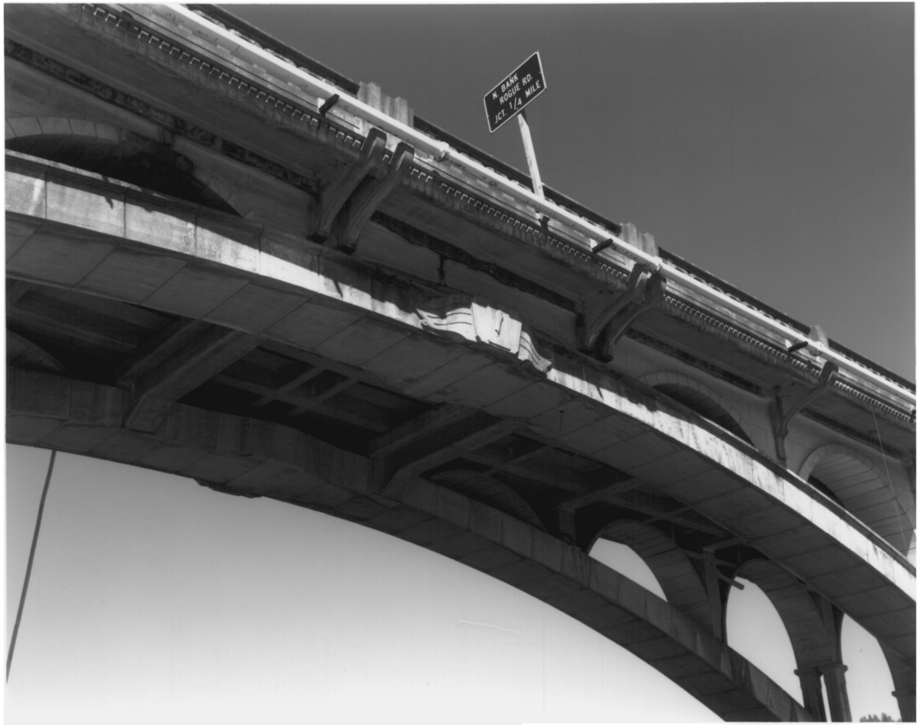
ROGUE RIVER BRIDGE, GOLD BEACH, OREGON #3
