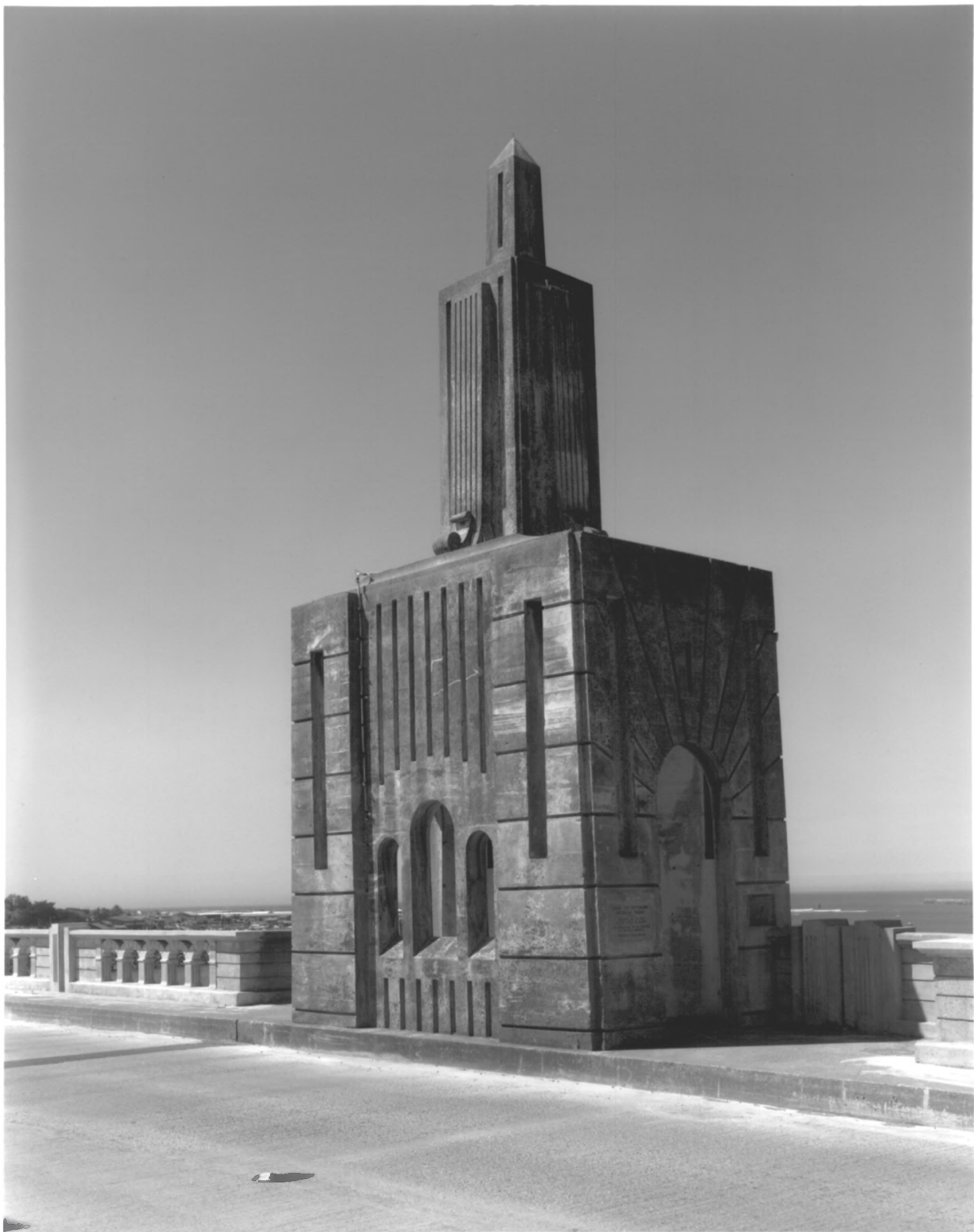
ROGUE RIVER BRIDGE, GOLD BEACH, OREGON #5
