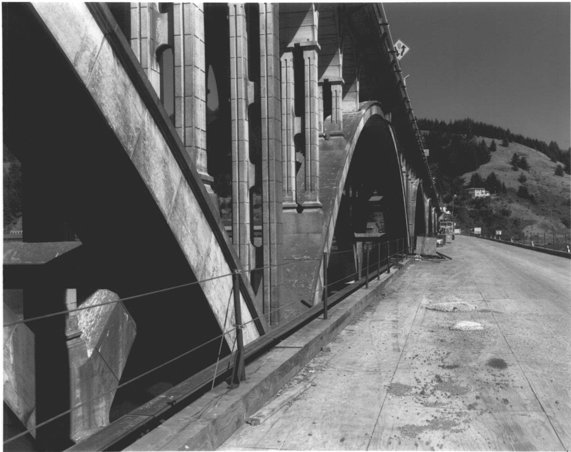
ROGUE RIVER BRIDGE, GOLD BEACH, OREGON #8
