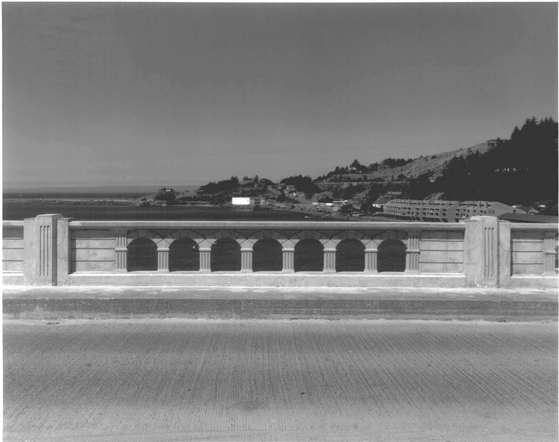
ROGUE RIVER BRIDGE, GOLD BEACH, OREGON
