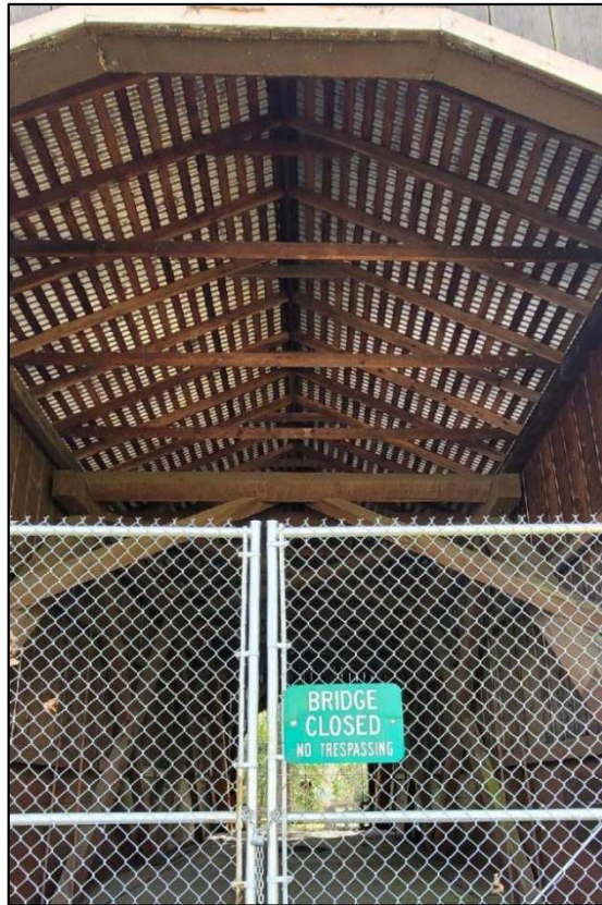
Photograph 8 of 9: OR_DouglasCounty_PassCreekCoveredBridge_0008 Top of wood Howe truss and roof framing inside Pass Creek Covered Bridge, camera facing south, the bridge's exposed interior trusswork clearly conveys its historic Howe-truss design, with diagonal timber members readily visible.
