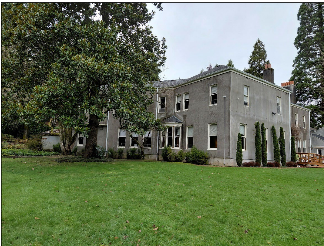
Photograph 6 of 21: OR_MultnomahCounty_KerrPeterandLaurieKingEstate_0006 South elevation of house, camera facing northwest.
