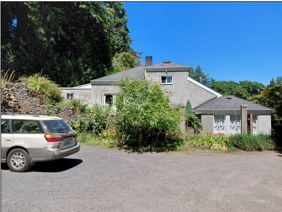
Photograph 8 of 21: OR_MultnomahCounty_KerrPeterandLaurieKingEstate_0008 South elevation of garage across visitor parking lot, camera facing north.
