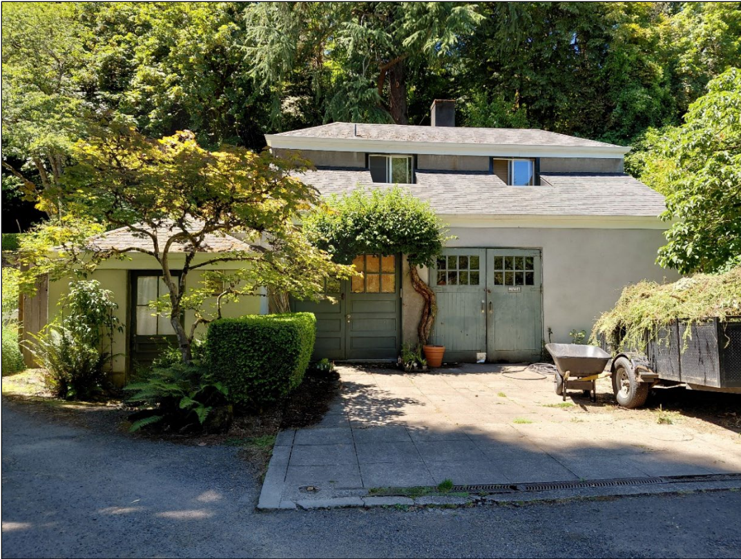
Photograph 7 of 21: OR_MultnomahCounty_KerrPeterandLaurieKingEstate_0007 East elevation of garage, camera facing west.
