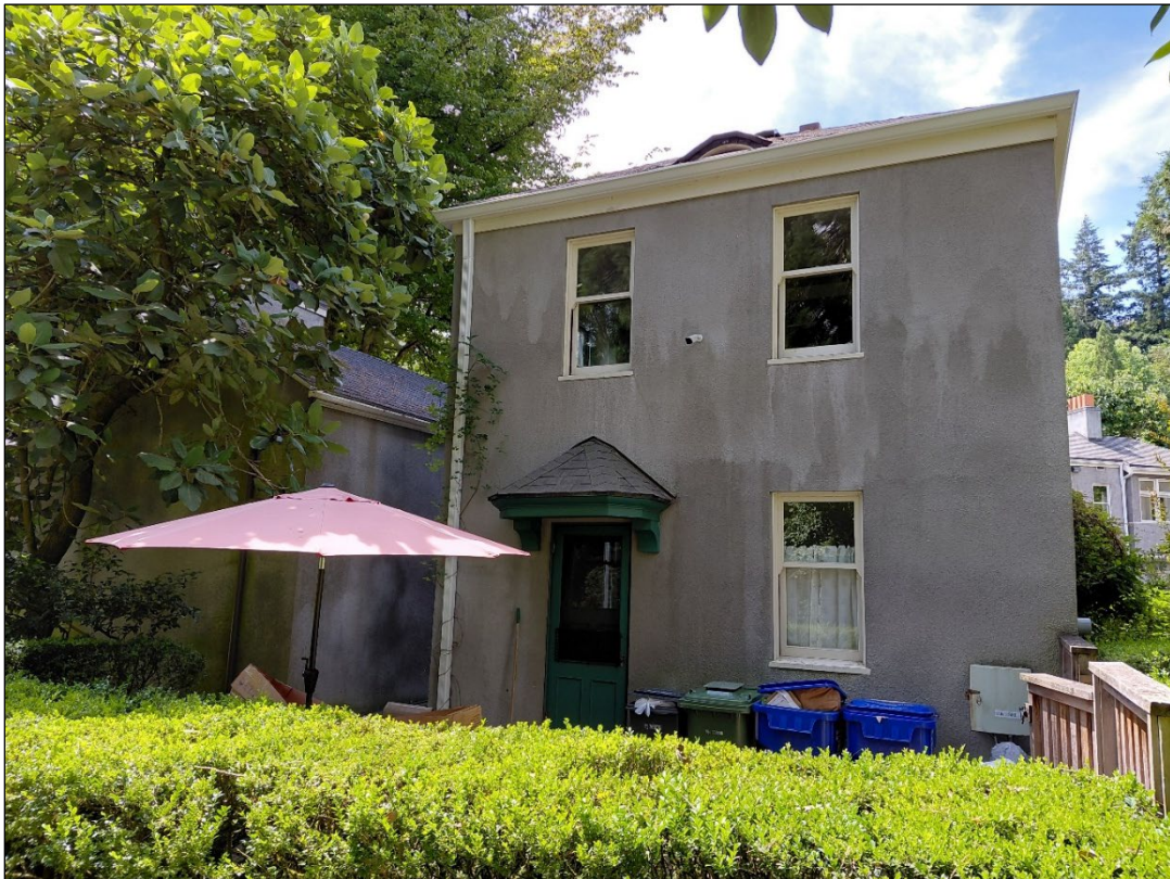
Photograph 4 of 21: OR_MultnomahCounty_KerrPeterandLaurieKingEstate_0004 North elevation of house, camera facing south.
