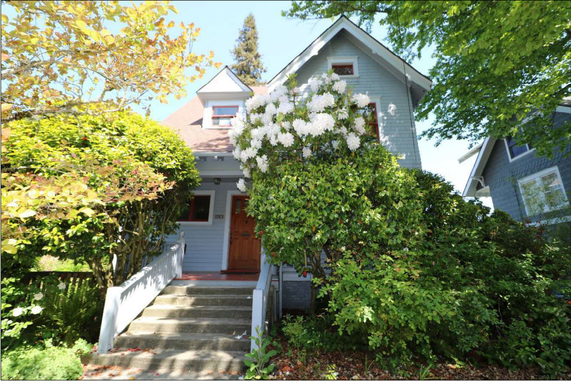
Photograph 3 of 18: OR_MultnomahCounty_LeGuinUrsulaKHouse_0003 South Elevation (Façade), view looking north.
