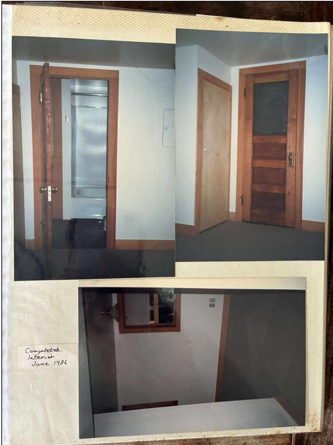
Figure 20: Basement apartment unit construction photos, 1986. View looking northeast at west elevation. Source: Le Guin Family Collection.
