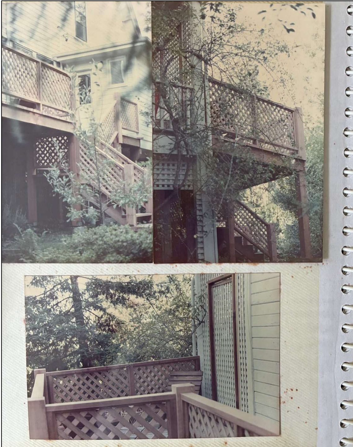
Figure 15: Construction photos showing new Laundry Room Addition and deck, 1984. Views looking at west elevation. Source: Le Guin Family Collection.
