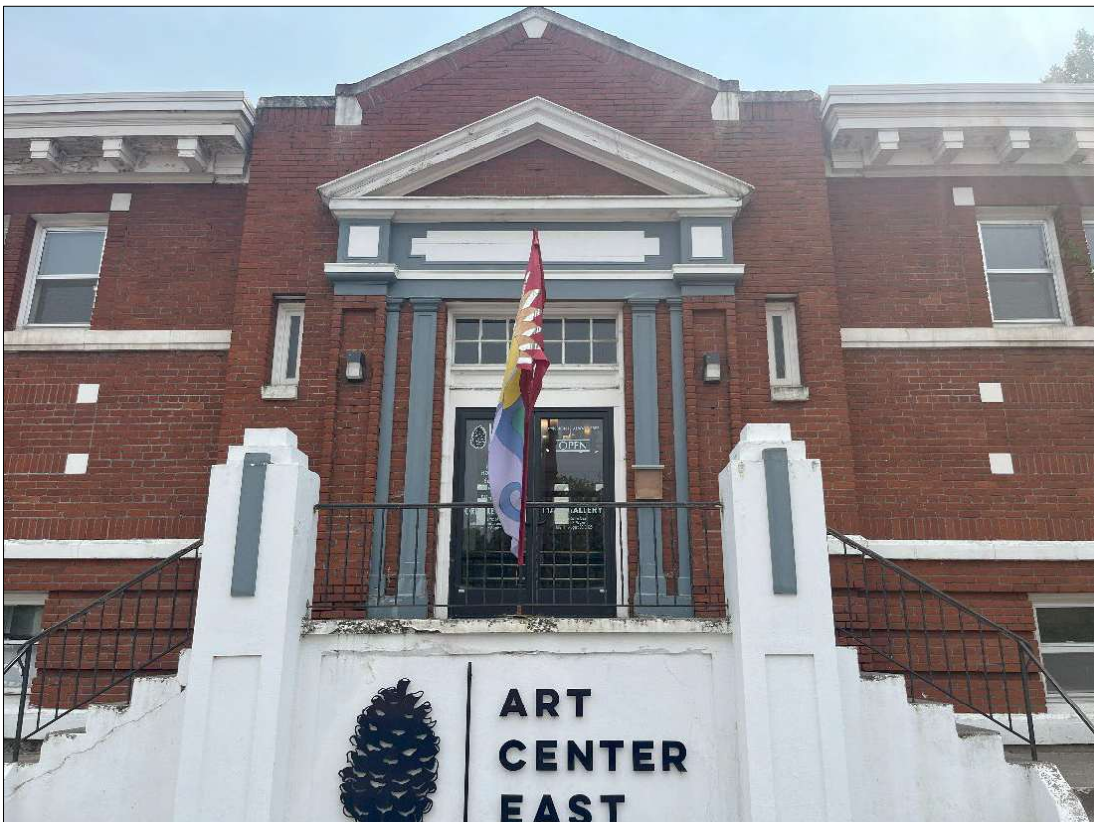
Photograph 2 of 10: OR_UnionCounty_LaGrandeCarnegieLibrary_0002 View of north façade entrance detail, looking south, September 4, 2025.
