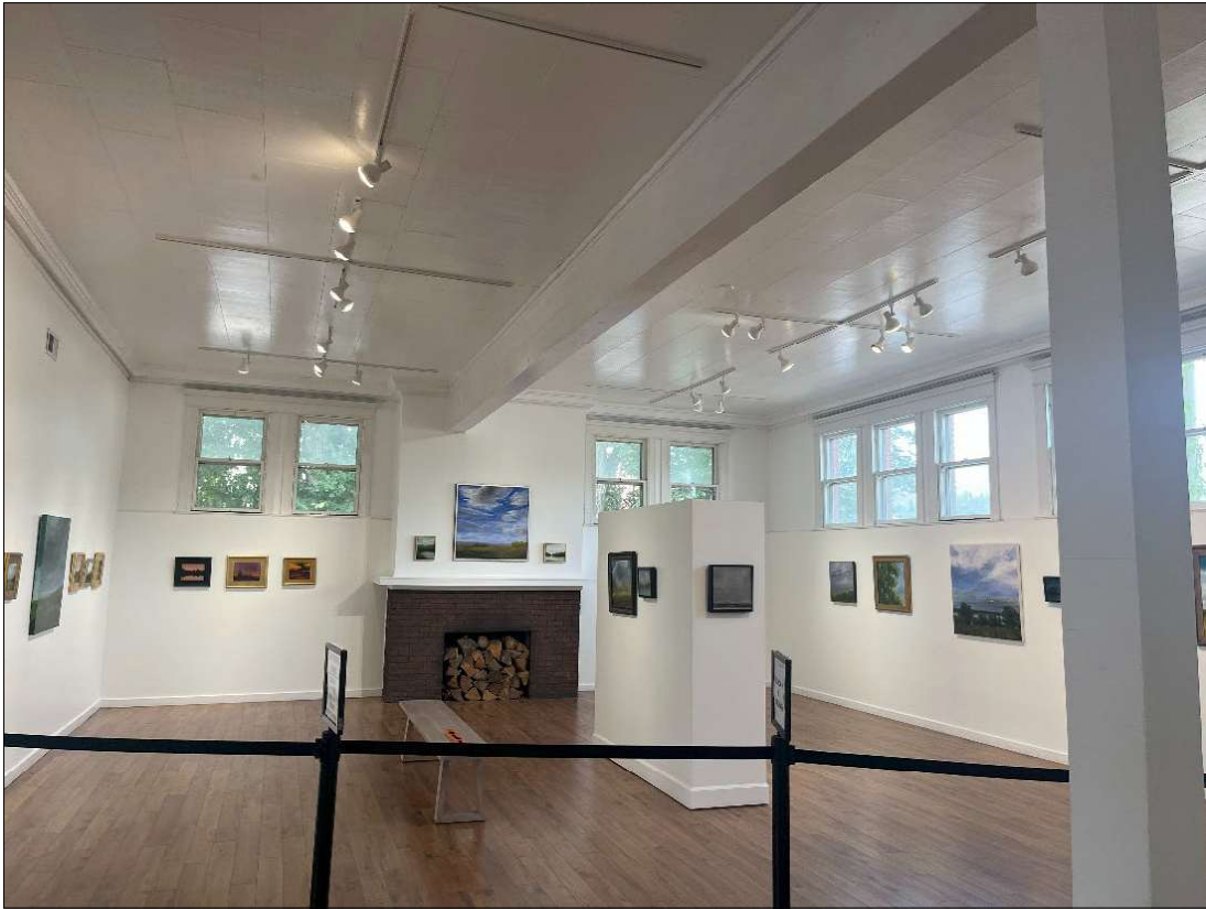
Photograph 7 of 10: OR_UnionCounty_LaGrandeCarnegieLibrary_0007 View of interior main level, looking west, September 5, 2025.
