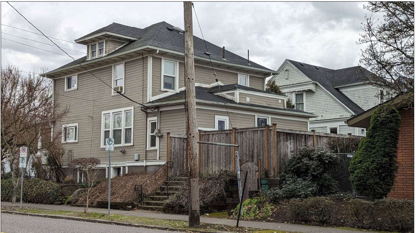
Photograph 4 of 15: OR_MultnomahCounty_JuniperHouse_0004 Side (west) and rear (south) facades. Camera facing northeast from SE 20 th Avenue.
