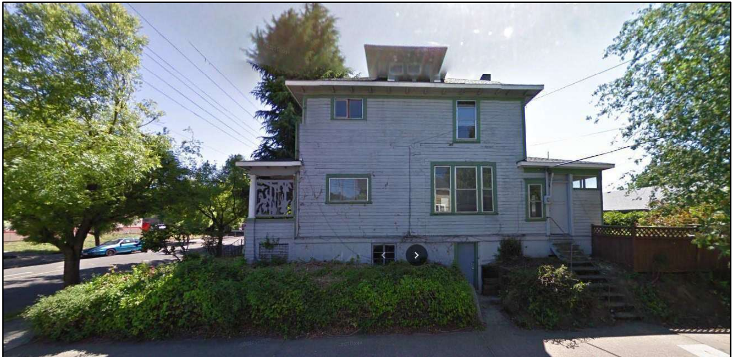
Figure 18. 2009 photograph of Juniper House, prior to 2010 renovations. Photo from SE 20 th Ave facing east, view of the west façade. Note the ghost shadows around the three-windows showing the original location of the oriel window. Note the rear porch door location and fixed windows on the corner that were removed in 2010. Source: Google Streetview.
