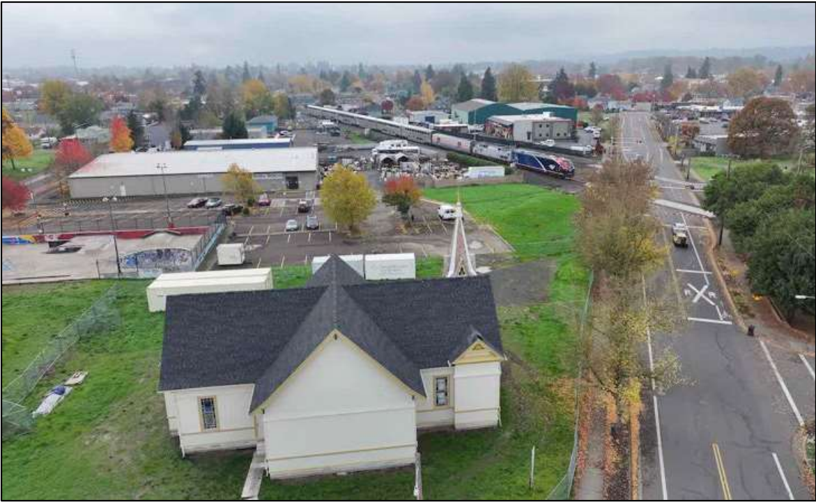
Photo 10 of 18: Aerial building and church setting, neighborhood view, camera facing west
