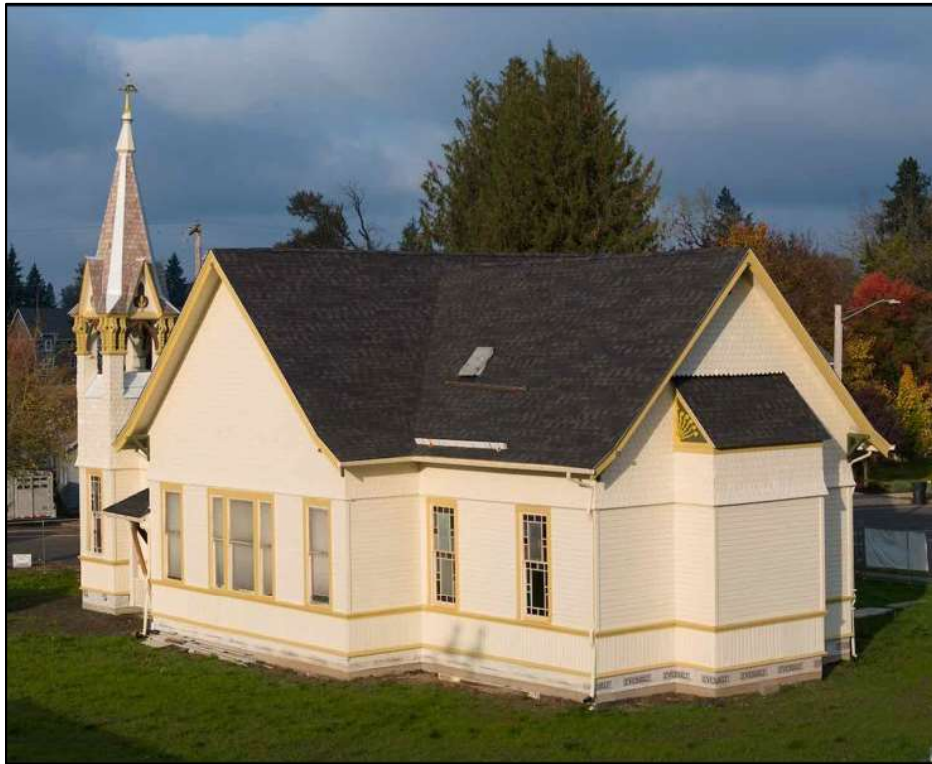
Photo 3 of 18: West elevation (left) and south elevation (right), camera facing northeast
