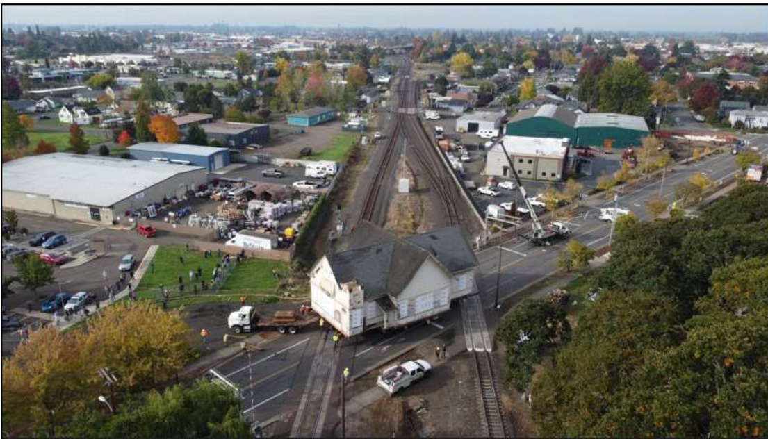
Figure 21: Image of Cumberland Presbyterian Church being moved across Union Pacific and Albany and Eastern railroad tracks
