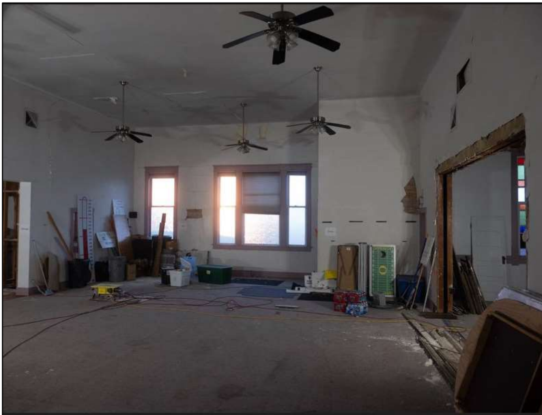
Photo 14 of 18: Interior of 1917 nave and entry (right), camera facing west
