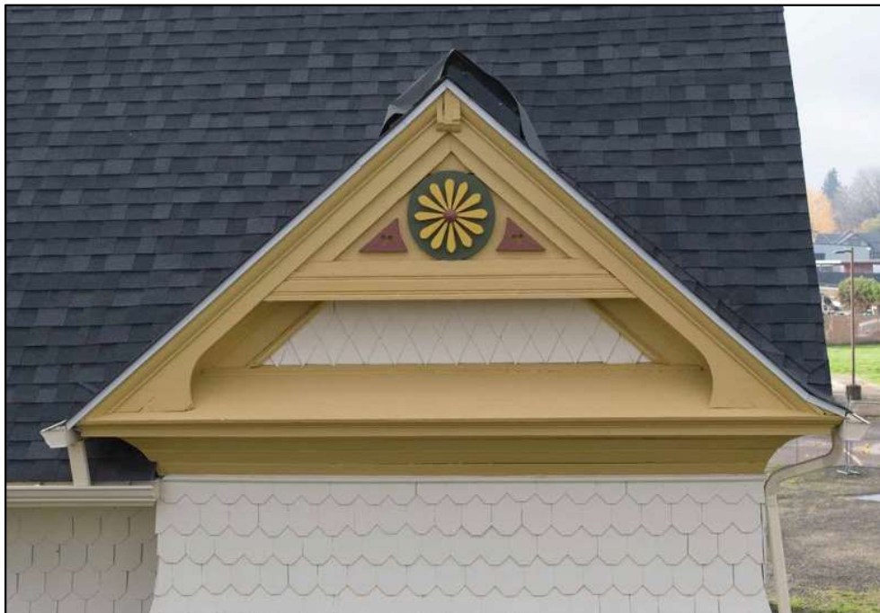
Photo 6 of 18: East chimney gable end, camera facing west
