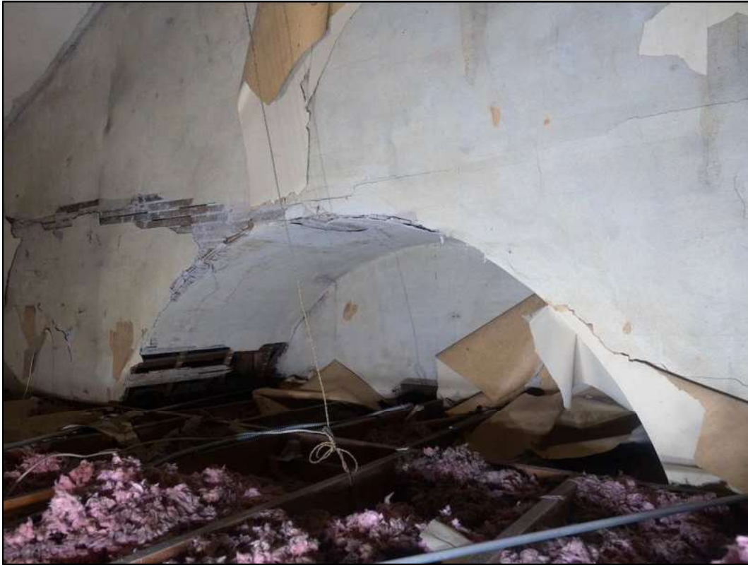
Photo 15 of 18: Interior 1892 apse sounding board above drop ceiling, camera facing southeast
