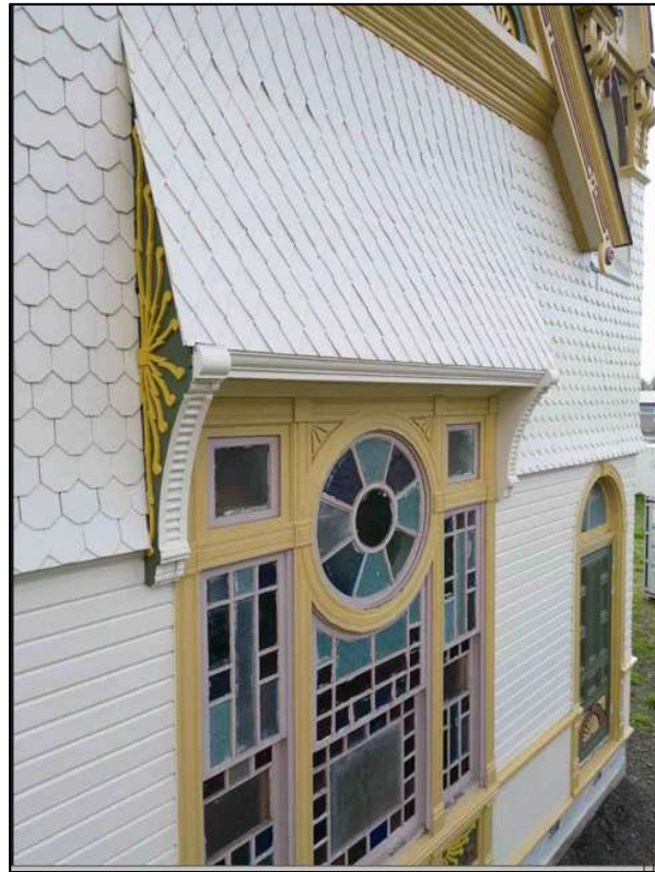
Photo 7 of 18: North façade ganged window unit, window hood, rose window, shingle patterns, camera facing southwest
