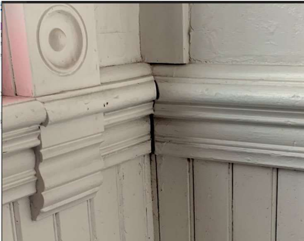
Photo 16 of 18: Interior 1892 moulding detail
