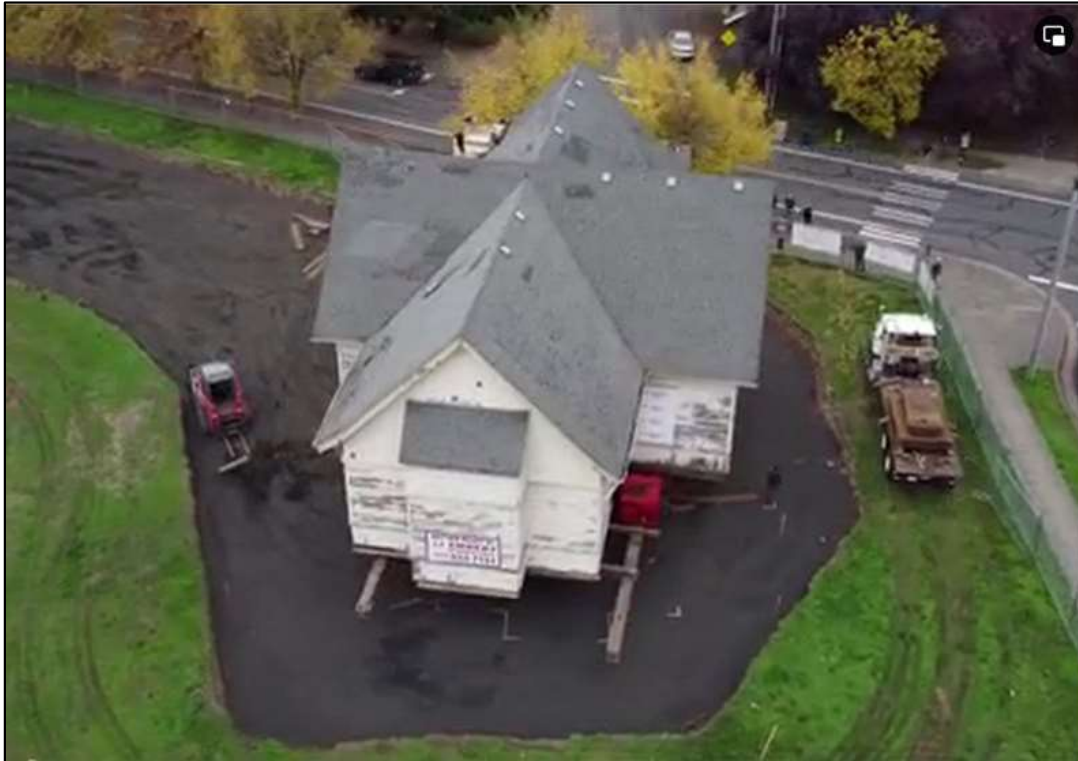
Figure 22: Image of Cumberland Presbyterian Church being rotated into place facing Santiam Road at new location.
