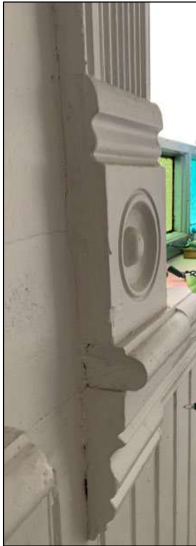
Photo 17 of 18: Additional 1892 moulding detail showing fluted casing, rosettes, bullnosed window stool, corner blocks, chair rail and wainscotting.
