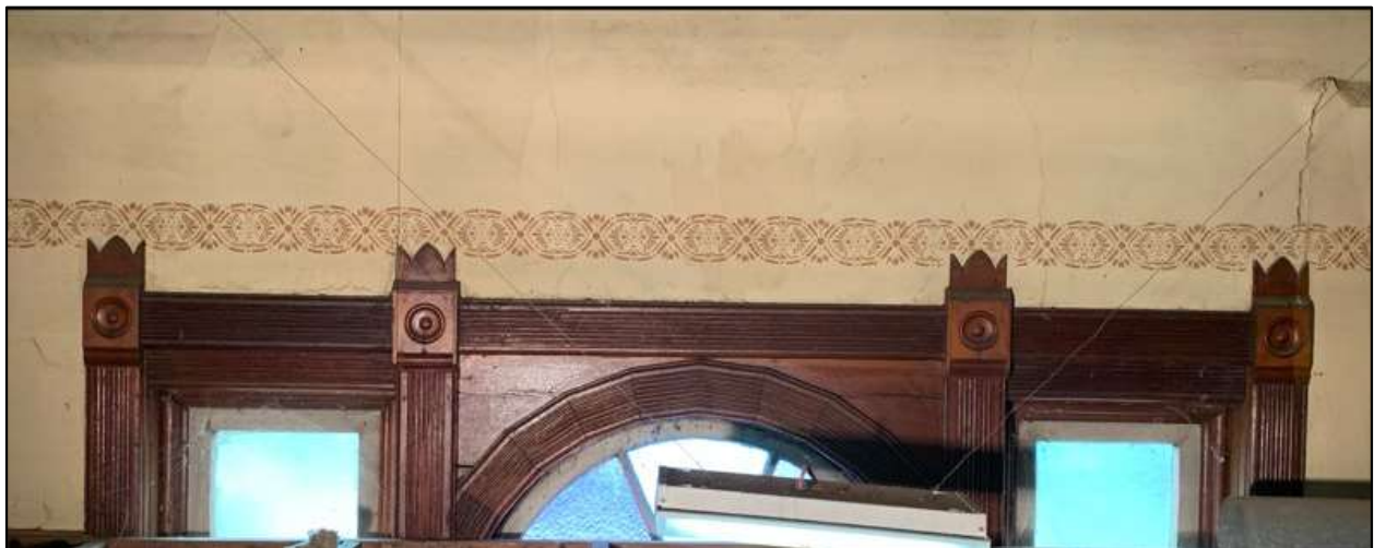
Photo 18 of 18: Interior 1892 moulding detail of ganged window in facade, camera facing north. Fluted casing topped by ornate wooden rosette style triple peaked head blocks. Copper colored wall stenciling
