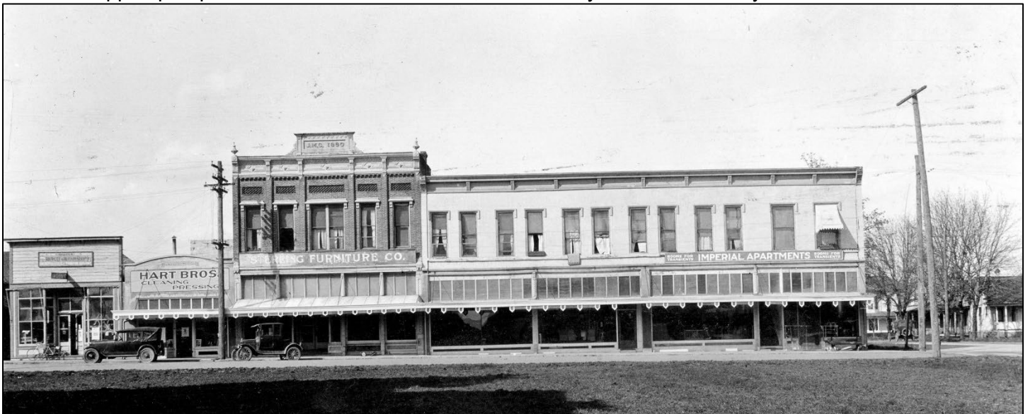
Fig. 18. Ca. 1919, SE Mill Street. Looking north from Courthouse Square with 166 SE Mill Street in the middle with the stepped parapet. Source: Dalton Collection, Polk County Historical Society.
