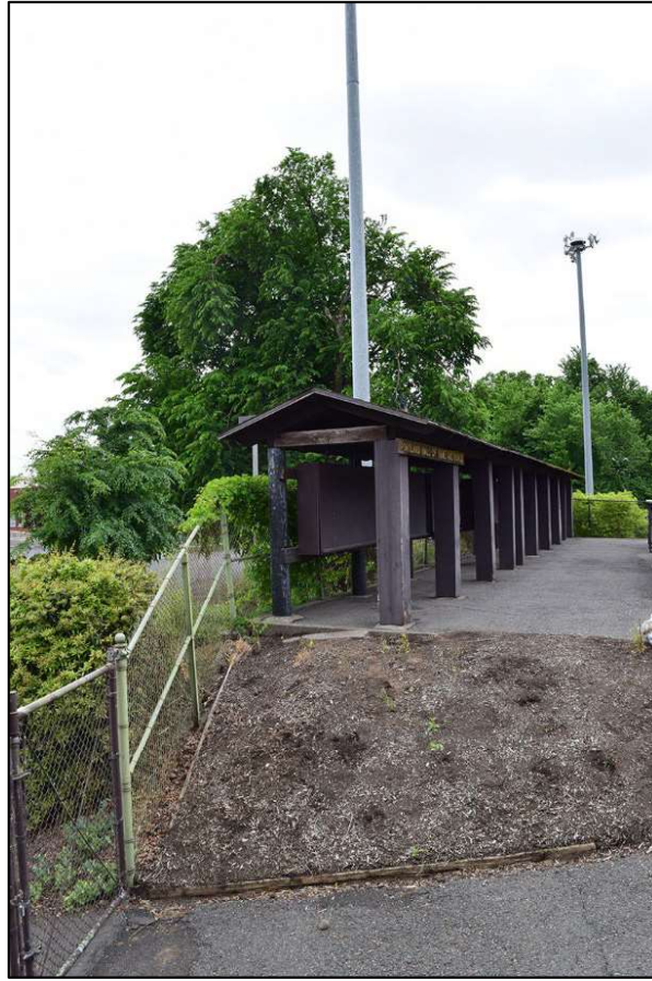
Photo 11 of 14: OR_Multnomah_NormandaleField_0011 Looking southwest from secondary stadium entry towards the “Hall of Fame”
