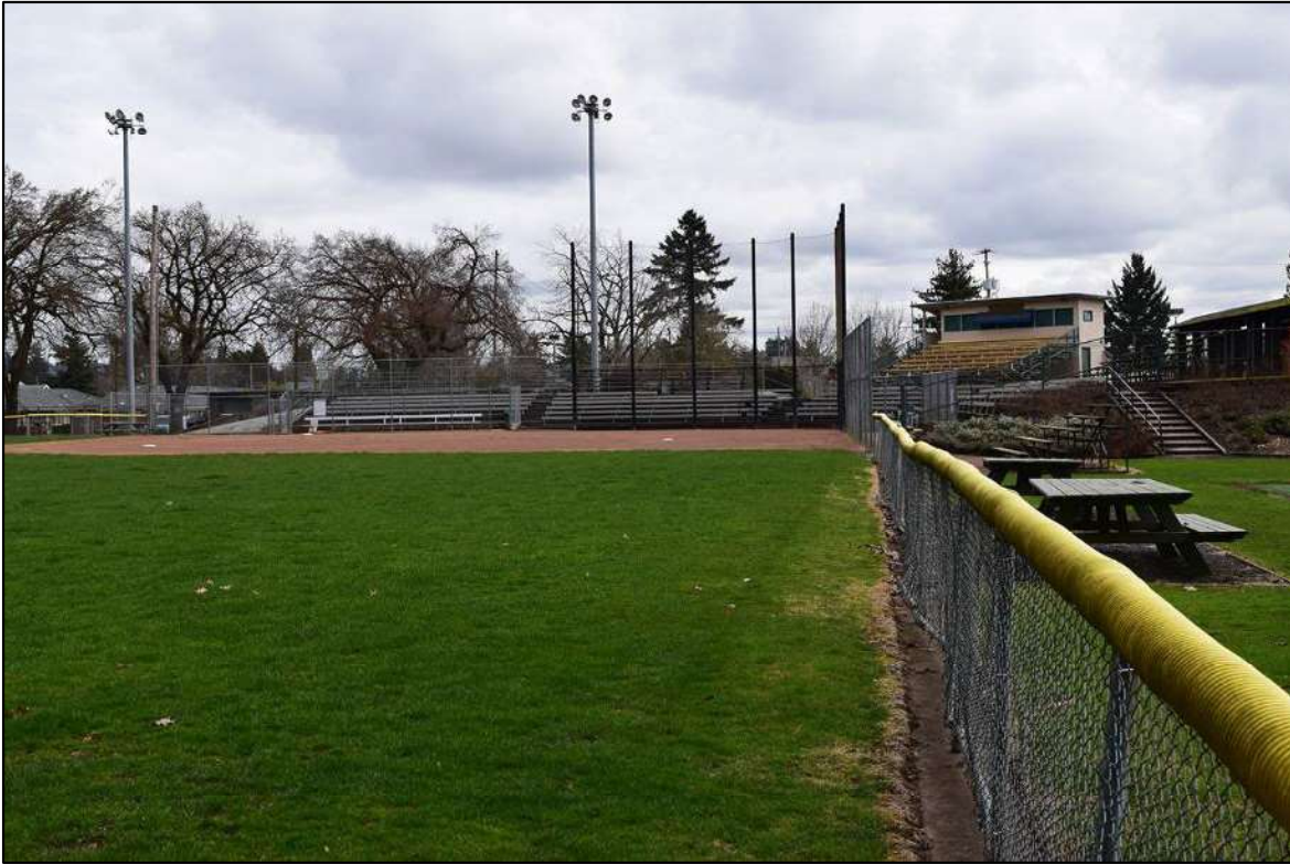
Photo 5 of 14: OR_Multnomah_NormandaleField_0005 Looking east across the outfield towards the infield
