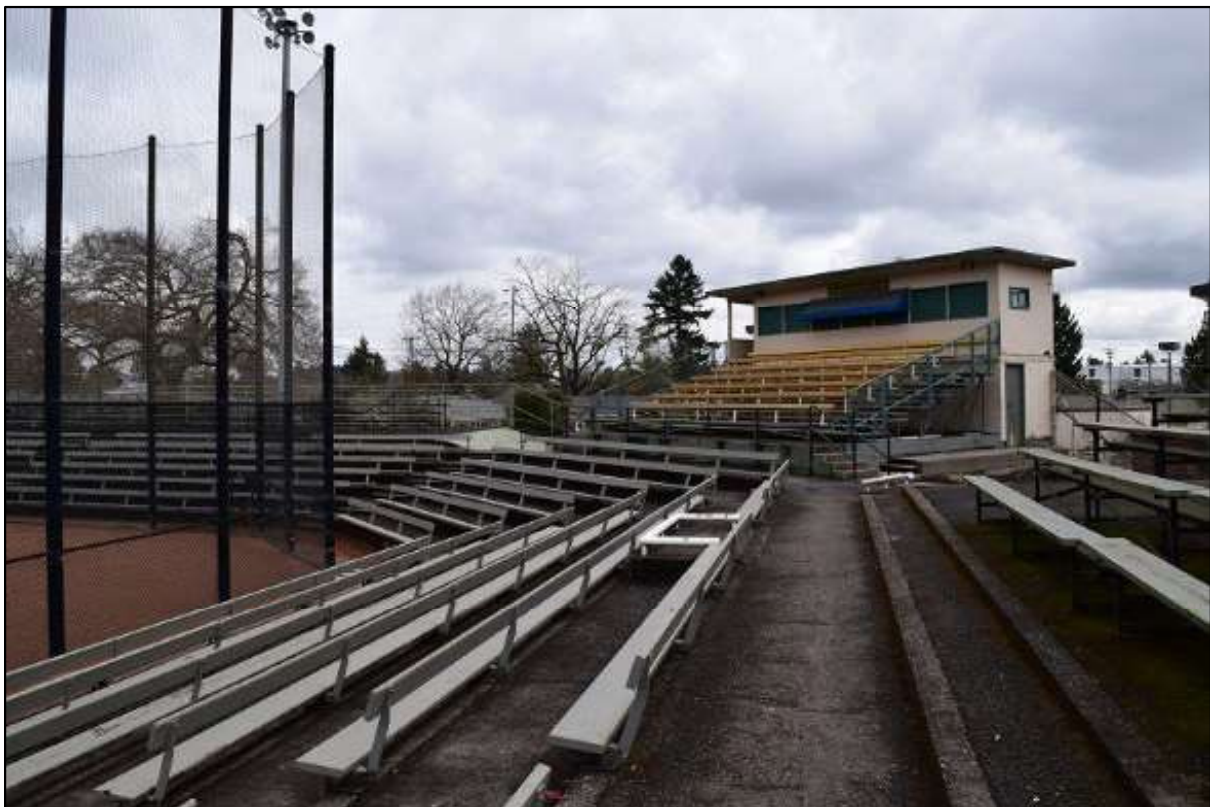
Photo 2 of 14: OR_Multnomah_NormandaleField_0002 Looking east from bleacher center walkway towards press box
