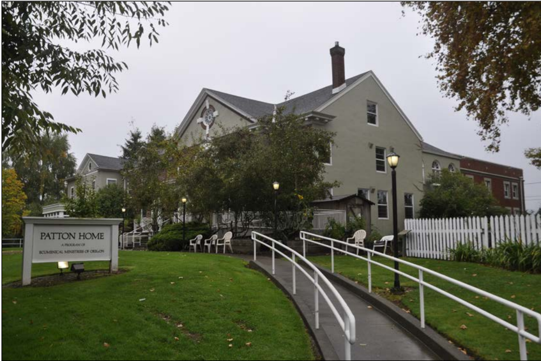
Photo 1 of 21: East and north elevations
