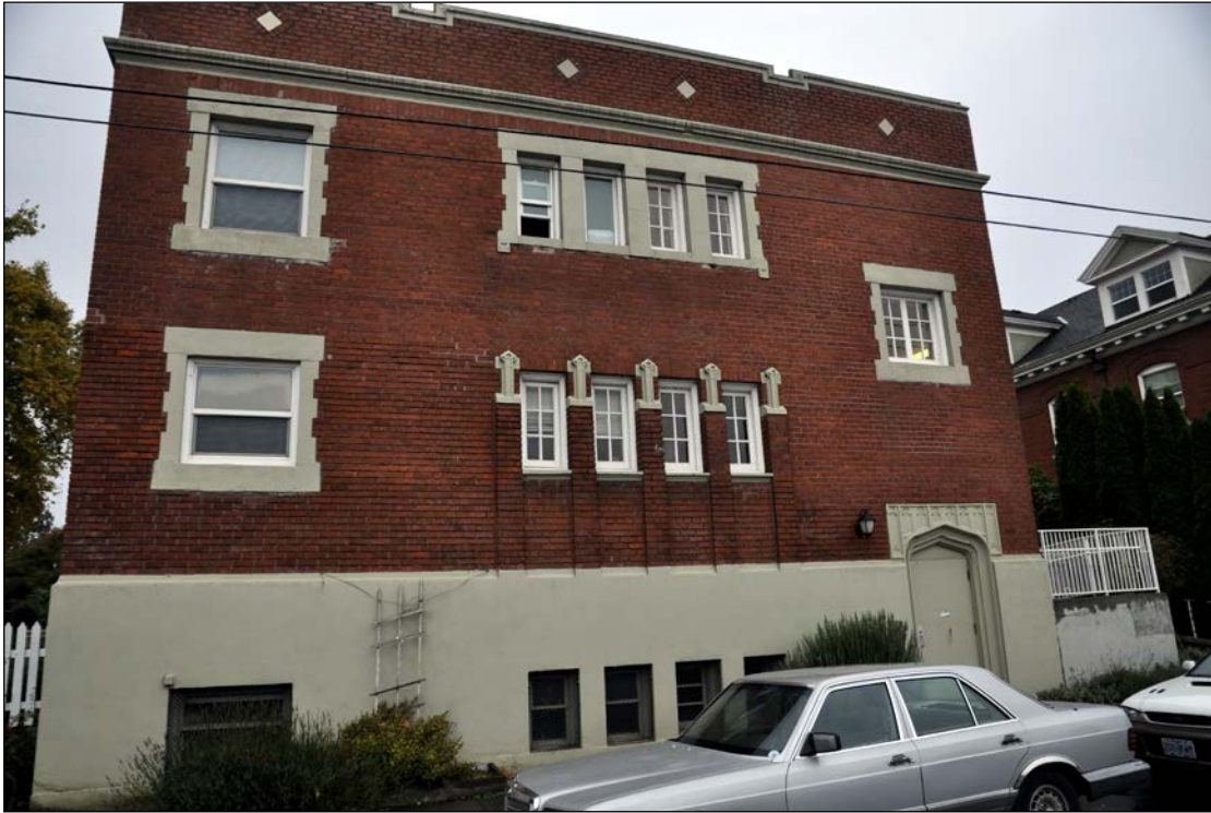
Photo 11 of 21: West elevation
