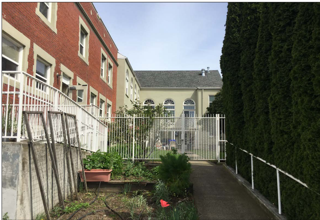
Photo 10 of 21: Courtyard looking east
