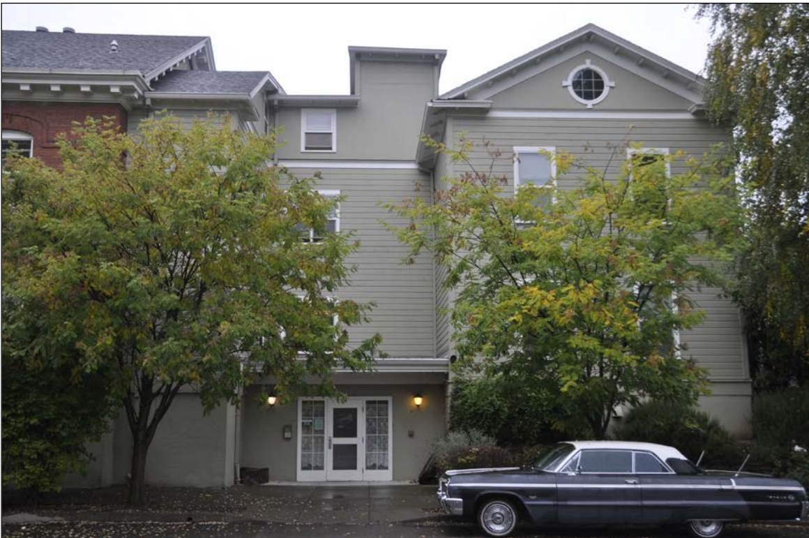
Photo 6 of 21: Wood frame portion of south elevation.
