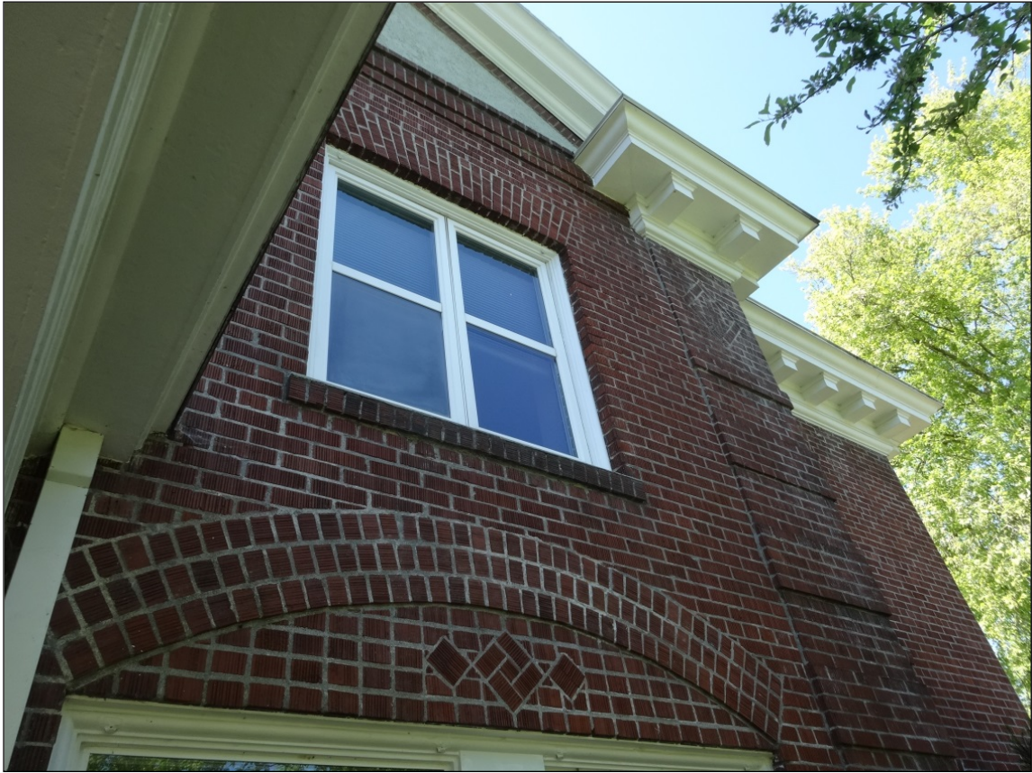
Photo 5 of 21: East elevation brick detailing and cornice.
