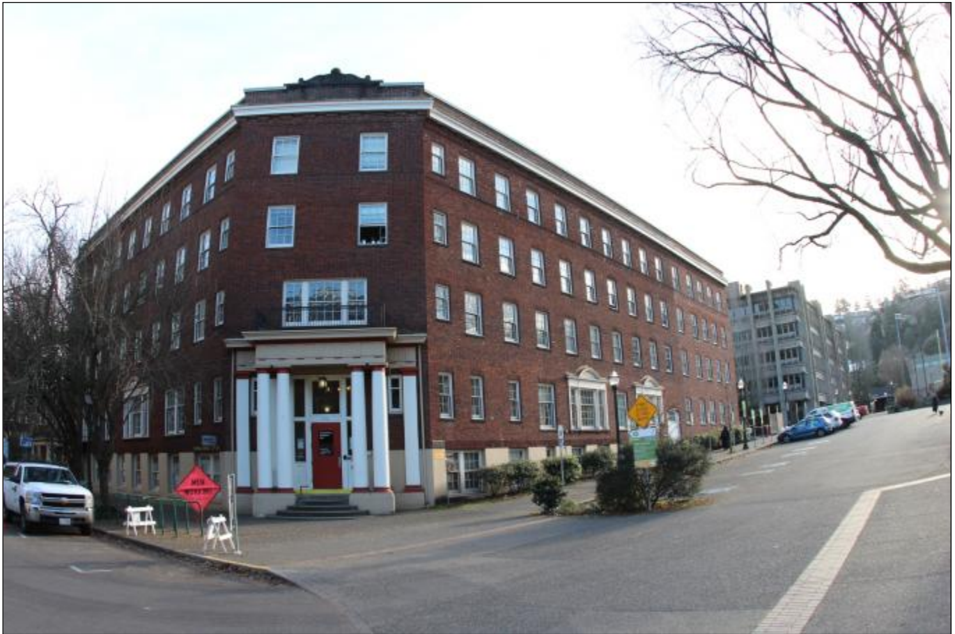
Figure 27: Martha Washington Hotel, 1802 SW 10 th Ave., Portland.
