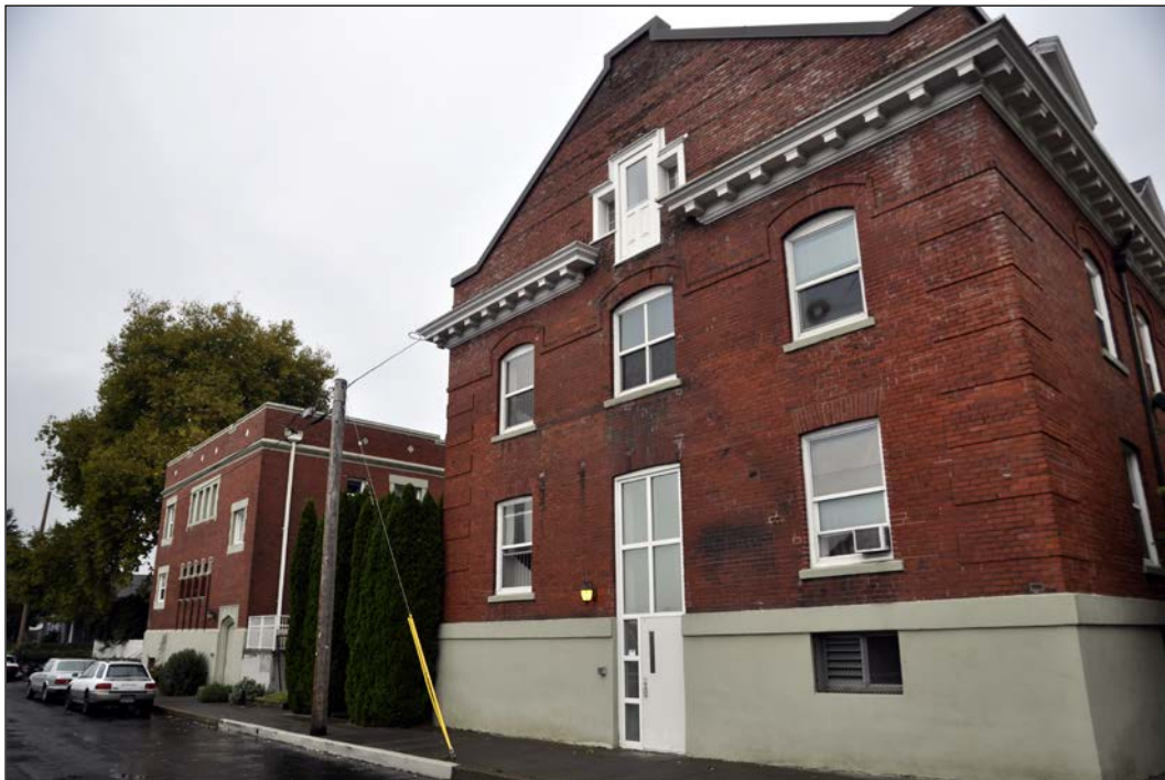
Photo 8 of 21: West elevation
