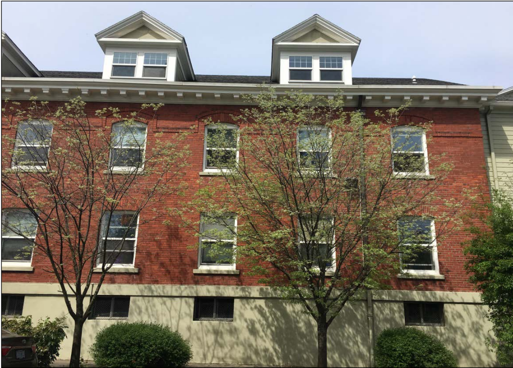
Photo 7 of 21: Masonry wing, south elevation.
