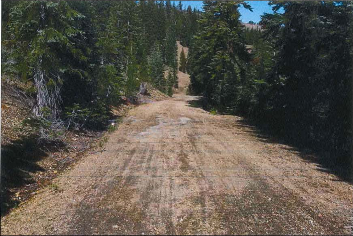
Photo 1 of 20: Typical section of Rim Road, Grayback Segment, looking east
