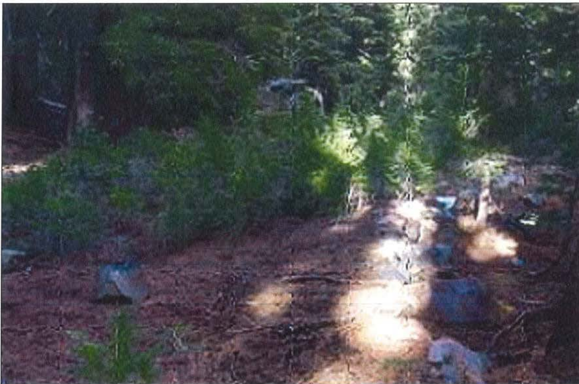
Photo 3 of 20: Abandoned section of Rim Road, showing base material, looking east
