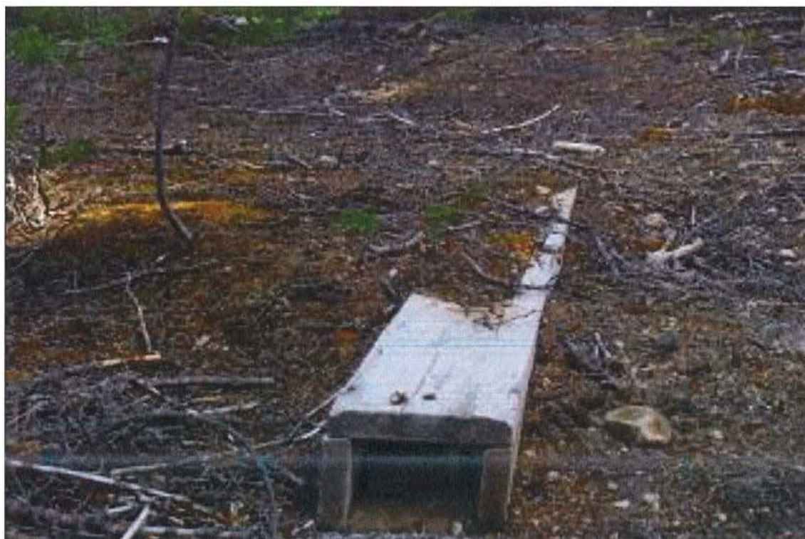
Photo 20 of 20: Log plank culvert on abandoned Rim Road, looking east
