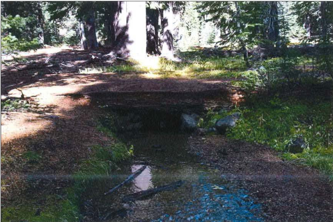
Photo 2 of 20: Cross drainage at Vidae Creek on Rim Road, looking north
