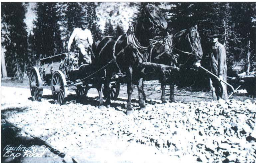
Figure 14: Spreading rock for experimental road surfacing in Munson Valley (Resource 3), 1913.
