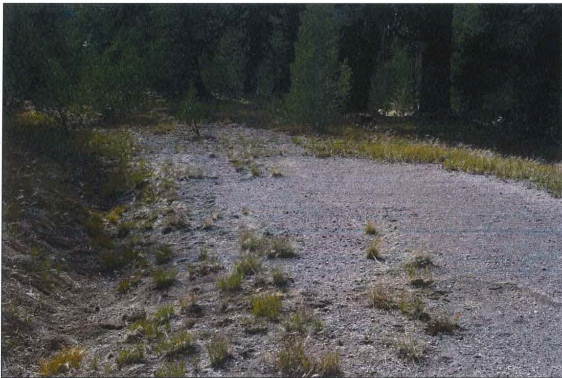
Photo 13 of 20: Typical section of Rim Road below Cloudcap showing ditch line on inside slope instead of culverts for cross drainage, looking north
