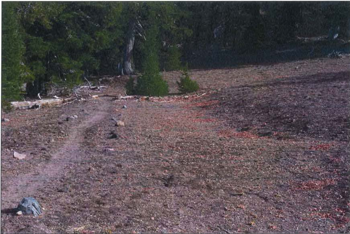
Photo 7 of 20: Rim Trail at left within a typical section of abandoned Rim Road, with small trees in the center of old roadway, looking east
