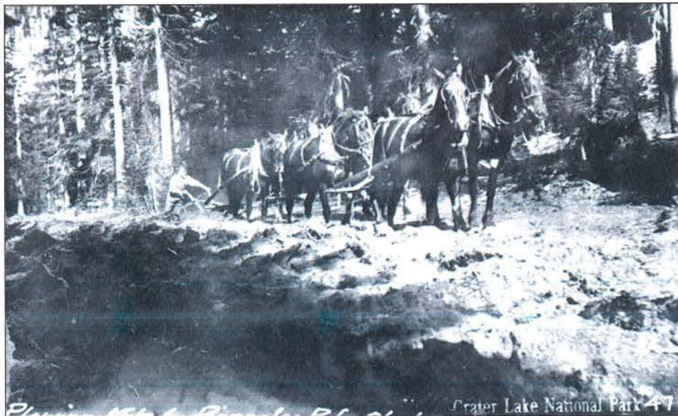
Figure 12: Rough grading with team of horses and plow, (just below Kerr Notch in Resource 18), 1913.
