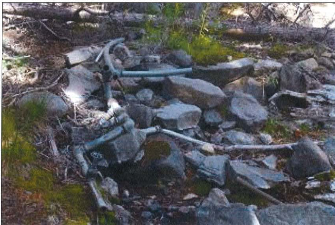
Photo 19 of 20: Abandoned water system next to overgrown section of Rim Road, looking south
