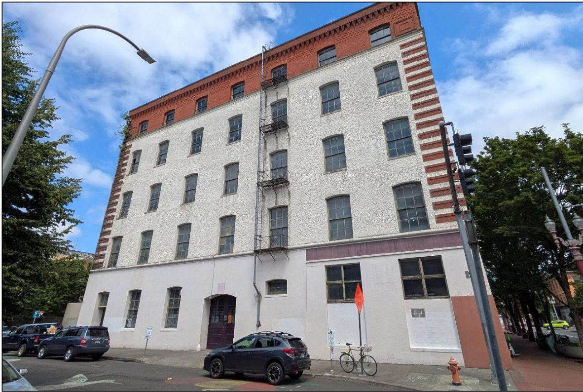
Photograph 3 of 15: OR_MultnomahCounty_OregonCasketCompanyBuilding_0003 South elevation; camera facing north.
