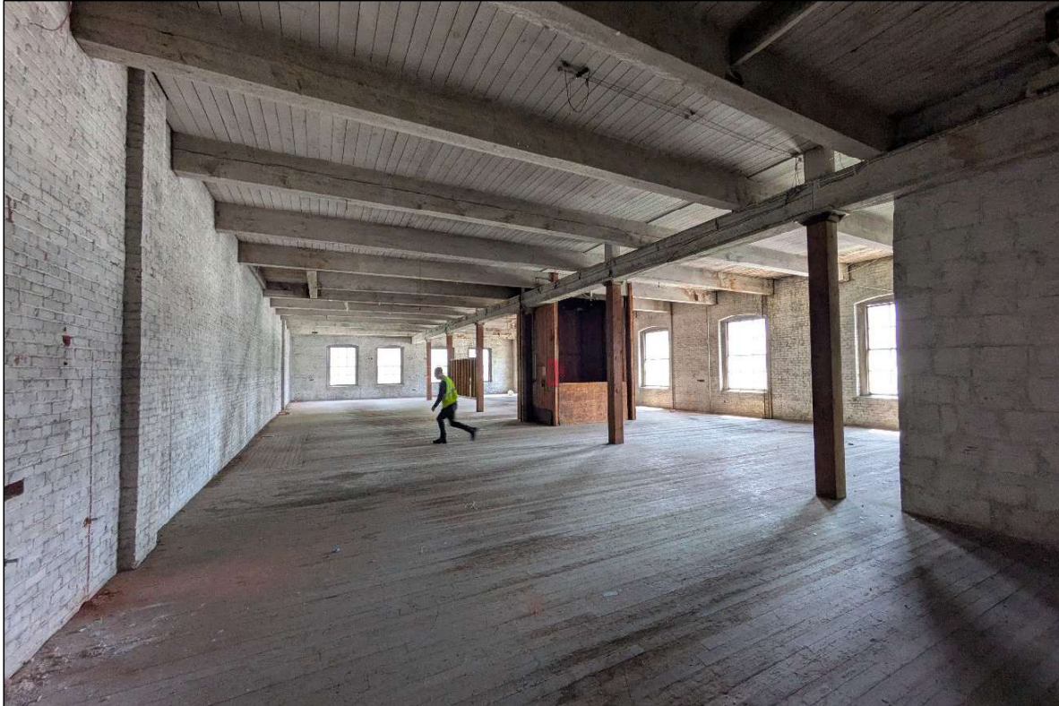
Photograph 12 of 15: OR_MultnomahCounty_OregonCasketCompanyBuilding_0012 Third floor showing elevator at middle and staircase enclosure at right; camera facing southeast. Ghost marks on the left wall and framing modifications at the ceiling indicated the location of an older staircase.
