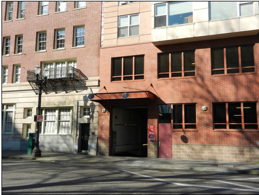
Photo 3 of 14: OR_MultnomahCounty_PortlandPoliceBlock(BoundaryDecrease)_0003 Entry at Southernmost Bay of East Elevation, Looking West
