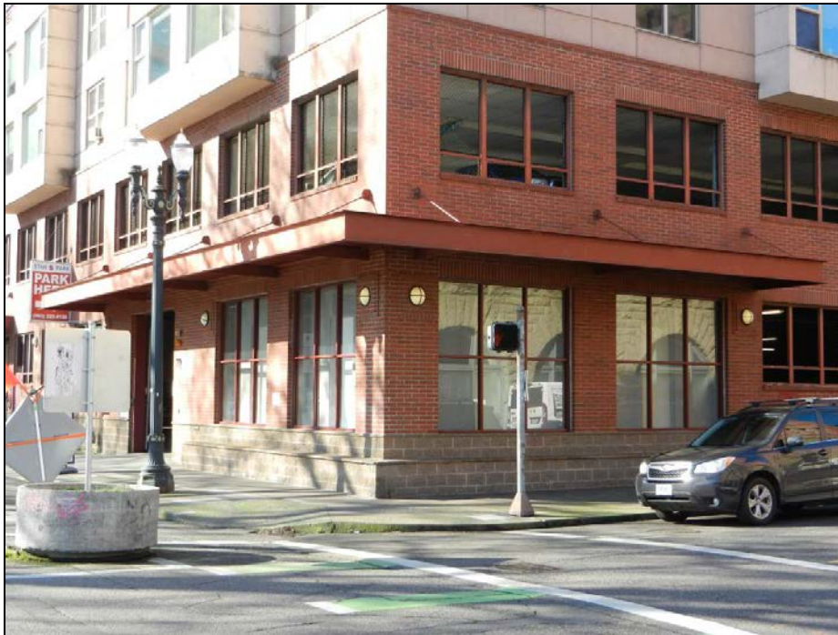
Photo 6 of 14: OR_MultnomahCounty_PortlandPoliceBlock(BoundaryDecrease)_0006 Enlarged Windows at Northeast Corner, Looking Southwest
