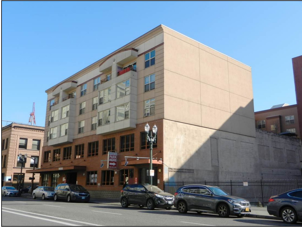
Photo 11 of 14: OR_MultnomahCounty_PortlandPoliceBlock(BoundaryDecrease)_0011 West and South Elevations, Looking Northeast
