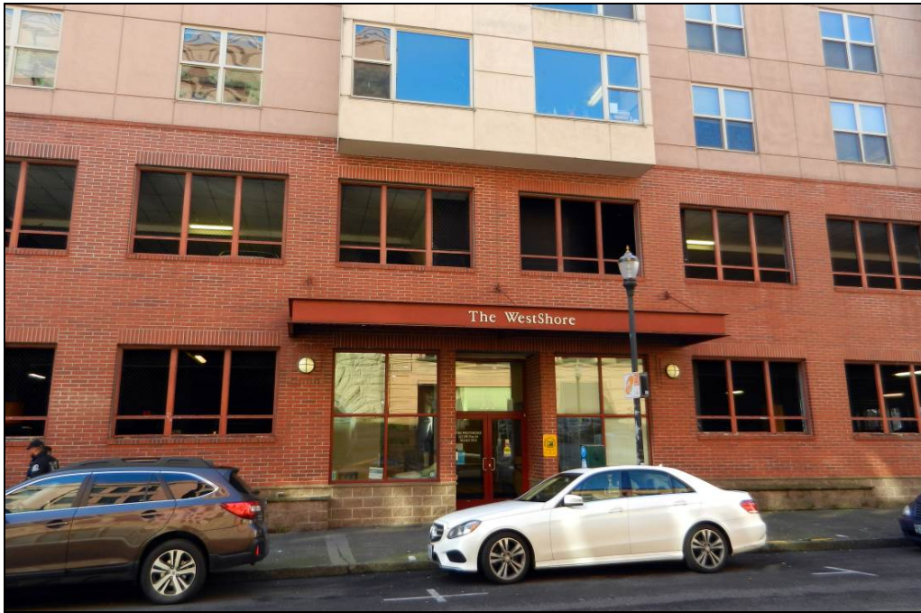
Photo 7 of 14: OR_MultnomahCounty_PortlandPoliceBlock(BoundaryDecrease)_0007 Entry at North Elevation, Looking South
