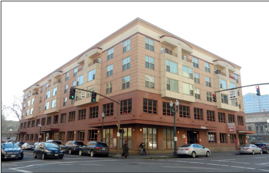
Photo 8 of 14: OR_MultnomahCounty_PortlandPoliceBlock(BoundaryDecrease)_0008 North and West Elevations, Looking Southeast
