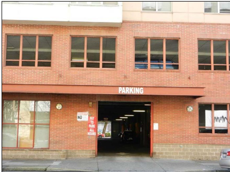
Photo 10 of 14: OR_MultnomahCounty_PortlandPoliceBlock(BoundaryDecrease)_0010 Non-original Entry, West Elevation, Looking East
