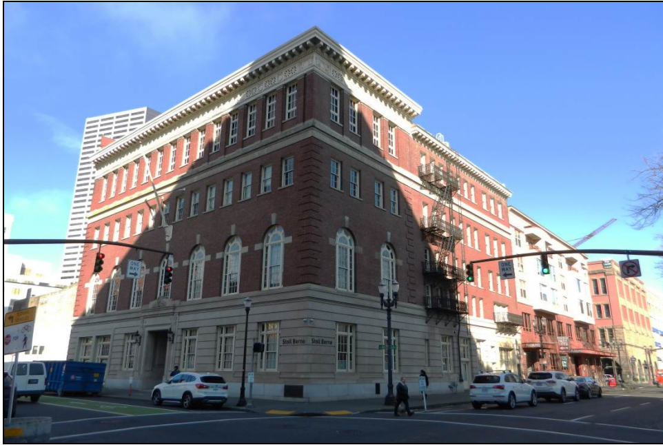
Photo 1 of 14: OR_MultnomahCounty_PortlandPoliceBlock(BoundaryDecrease)_0001 Portland Police Headquarters, South (Front) and East Elevations, Looking Northwest
