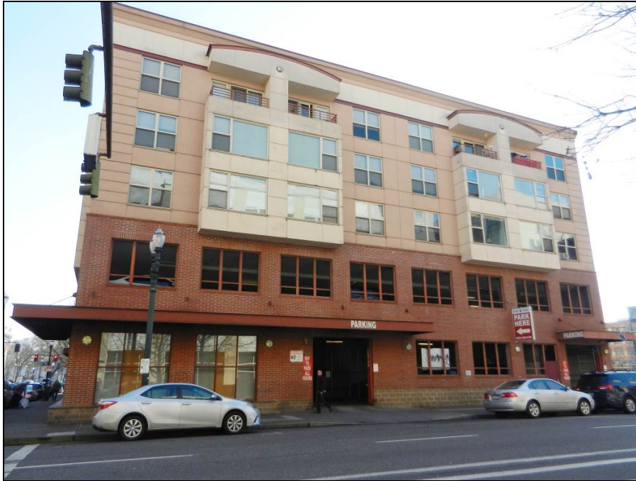
Photo 9 of 14: OR_MultnomahCounty_PortlandPoliceBlock(BoundaryDecrease)_0009 West Elevation, Looking East
