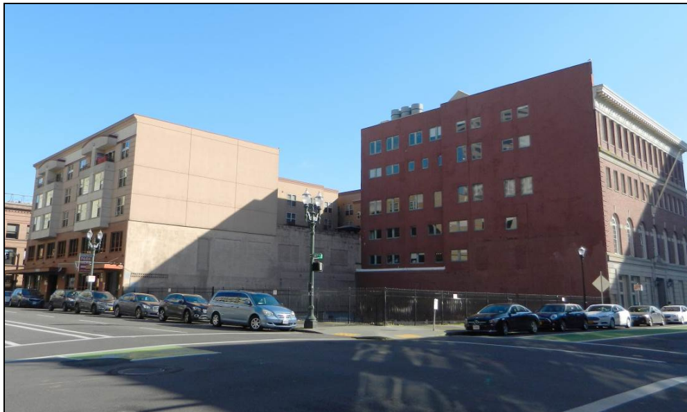
Photo 12 of 14: OR_MultnomahCounty_PortlandPoliceBlock(BoundaryDecrease)_0012 1955/1998 Addition (Left) and Portland Police Headquarters (Right), Looking Northeast
