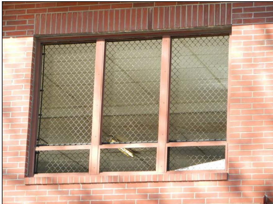
Photo 4 of 14: OR_MultnomahCounty_PortlandPoliceBlock(BoundaryDecrease)_0004 Detail of Second-story Window, East Elevation, Looking West
