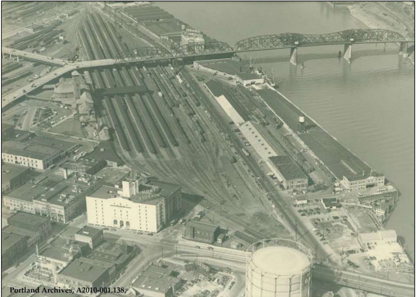
Figure 9. 1938 aerial photograph looking northwest at Union Station and the Broadway Bridge. Portland City Archives, A2010-001.138.
