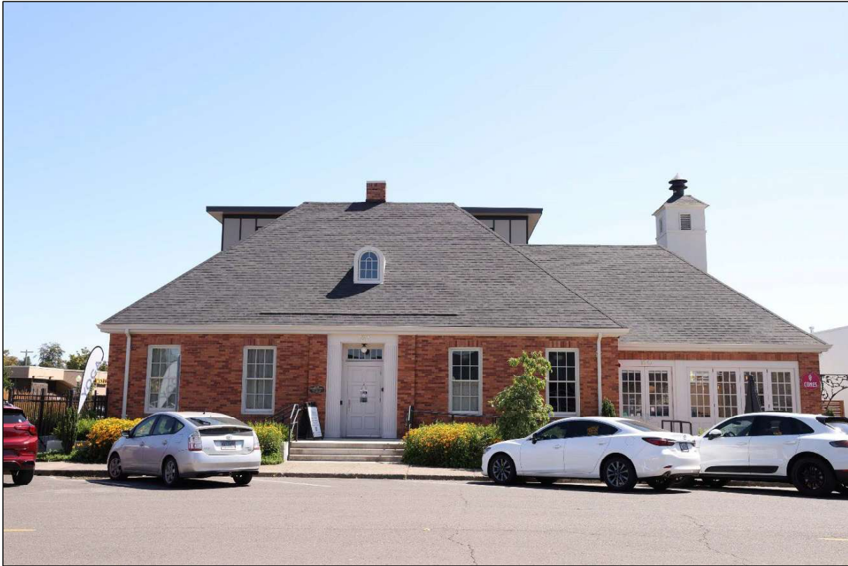
Photograph 1 of 16: OR_ClackamasCounty_CanbyCityHall_0001 Overview of Canby City Hall showing west (primary) façade, camera facing east-northeast.
