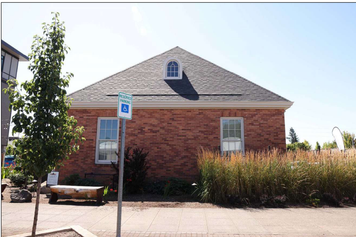
Photograph 4 of 16: OR_ClackamasCounty_CanbyCityHall_0004 North façade of main volume, camera facing south-southeast.
