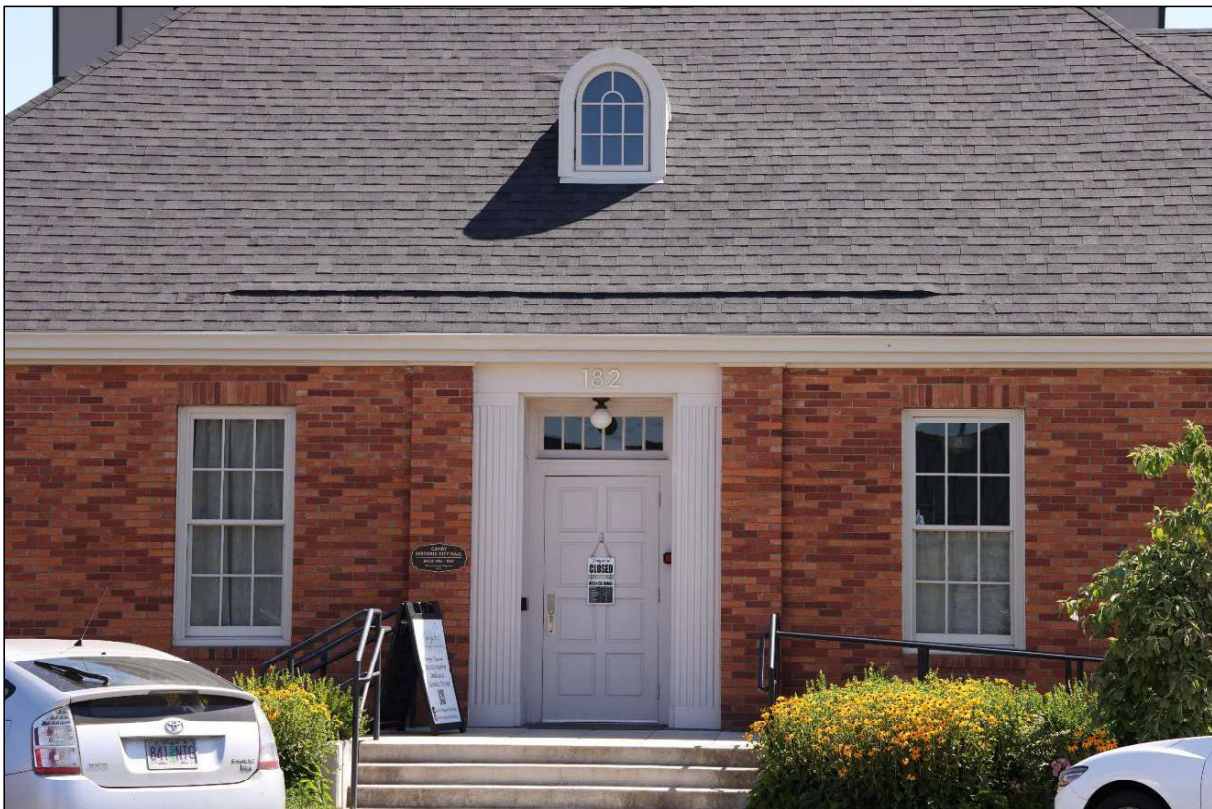
Photograph 2 of 16: OR_ClackamasCounty_CanbyCityHall_0002 Primary entrance centered in west façade of main volume, camera facing east-northeast.
