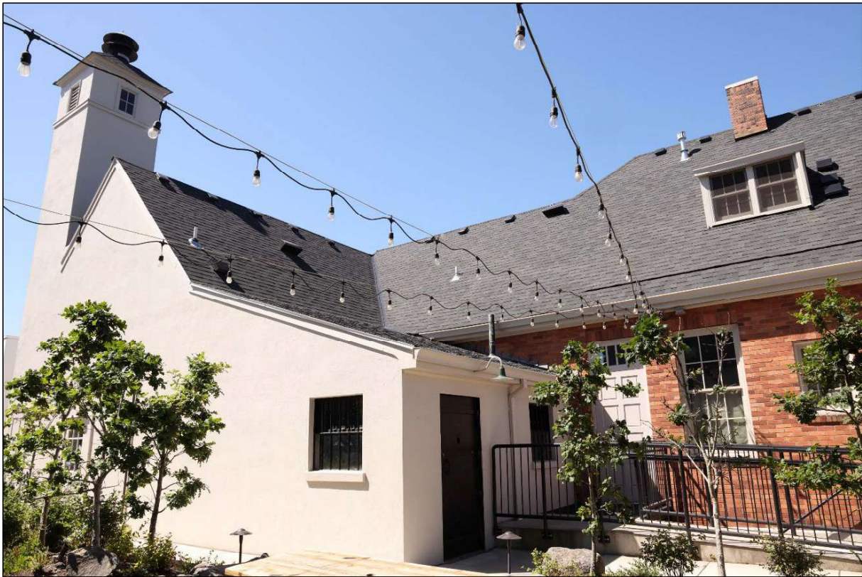
Photograph 7 of 16: OR_ClackamasCounty_CanbyCityHall_0007 Oblique view of east façade centered on the jail, camera facing south-southwest.
