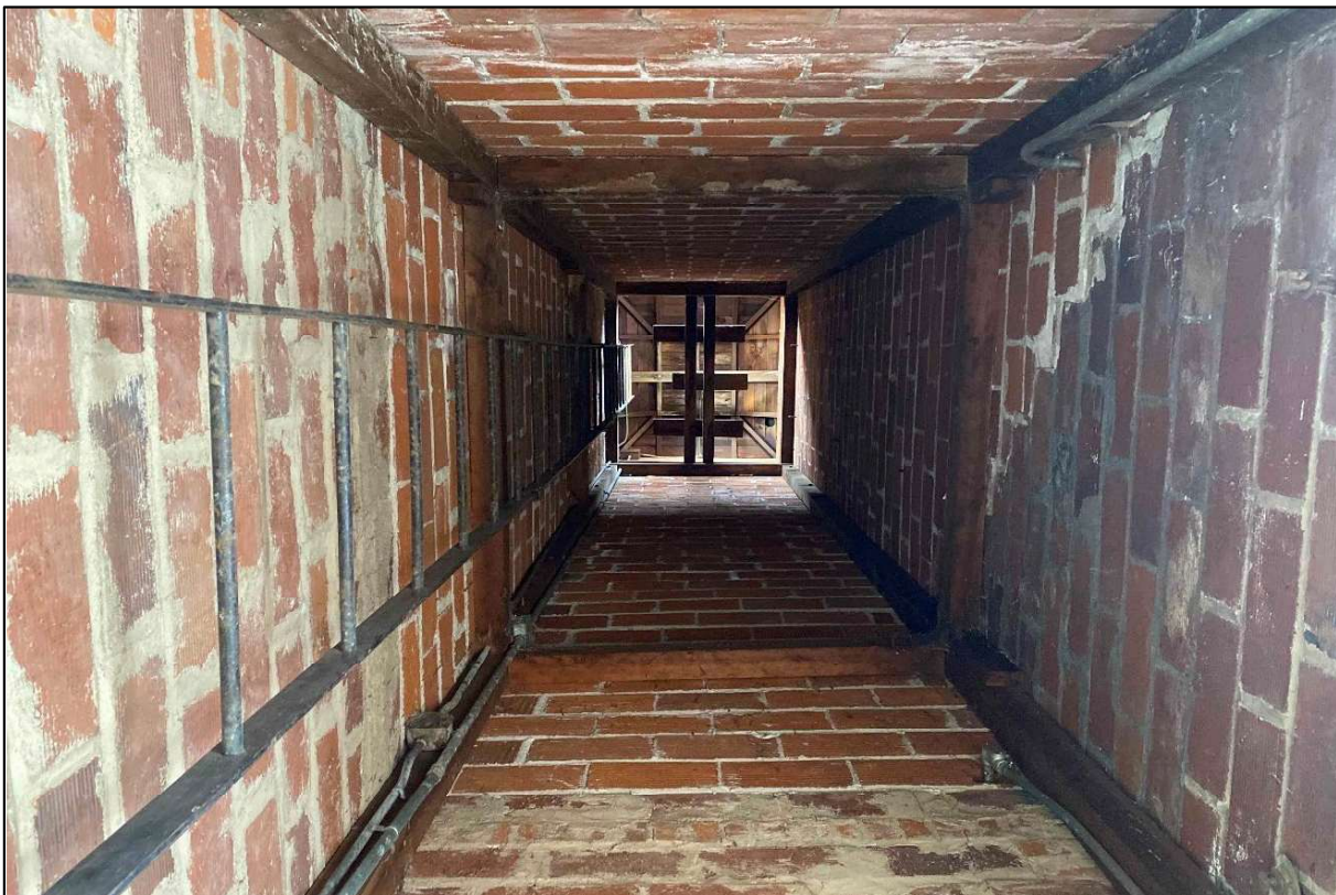
Photograph 14 of 16: OR_ClackamasCounty_CanbyCityHall_0014 Interior of hose tower, camera facing up.
