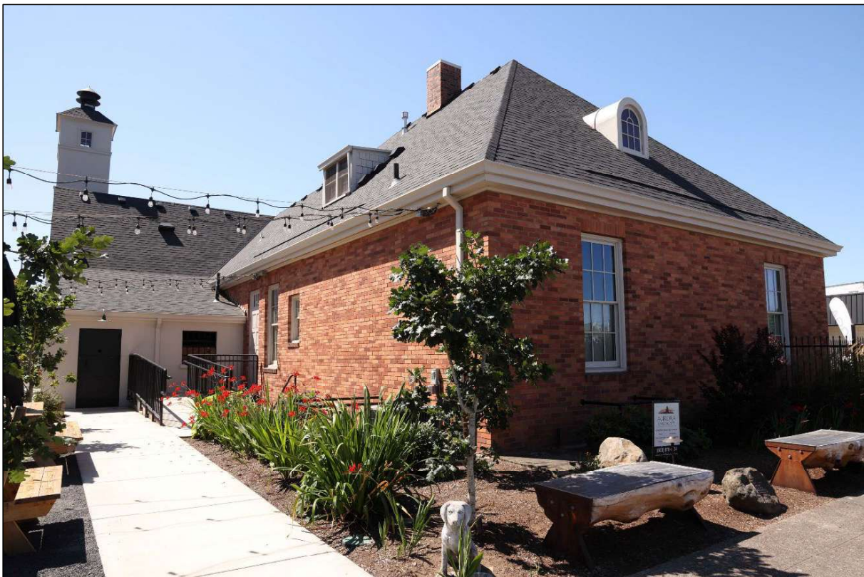
Photograph 6 of 16: OR_ClackamasCounty_CanbyCityHall_0006 Oblique view of east and north façades, camera facing south.
