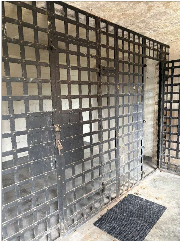
Photograph 15 of 16: OR_ClackamasCounty_CanbyCityHall_0015 Interior of jail showing partition and cell doors, camera facing south-southwest.
