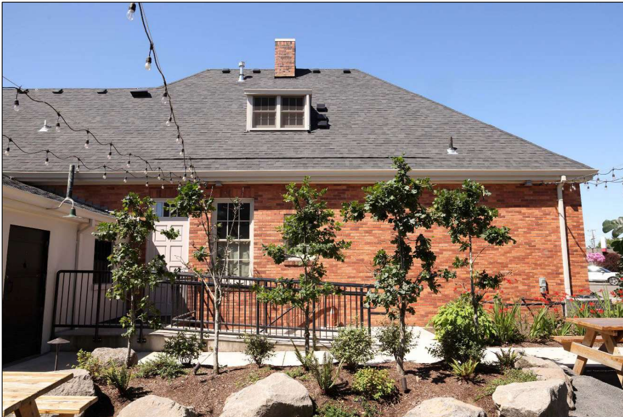
Photograph 5 of 16: OR_ClackamasCounty_CanbyCityHall_0005 East façade of main volume, camera facing west-southwest.
