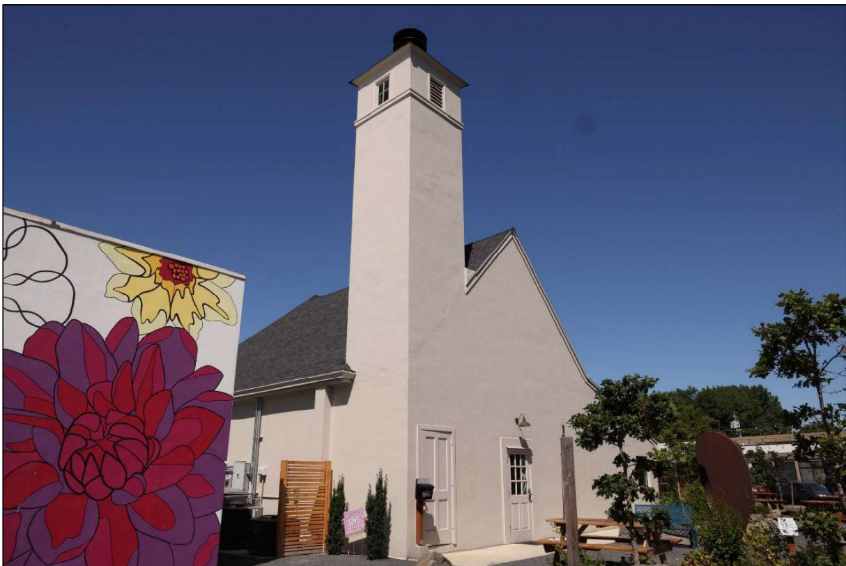
Photograph 8 of 16: OR_ClackamasCounty_CanbyCityHall_0008 Oblique view of firehouse showing south and east façades, camera facing north-northwest.
