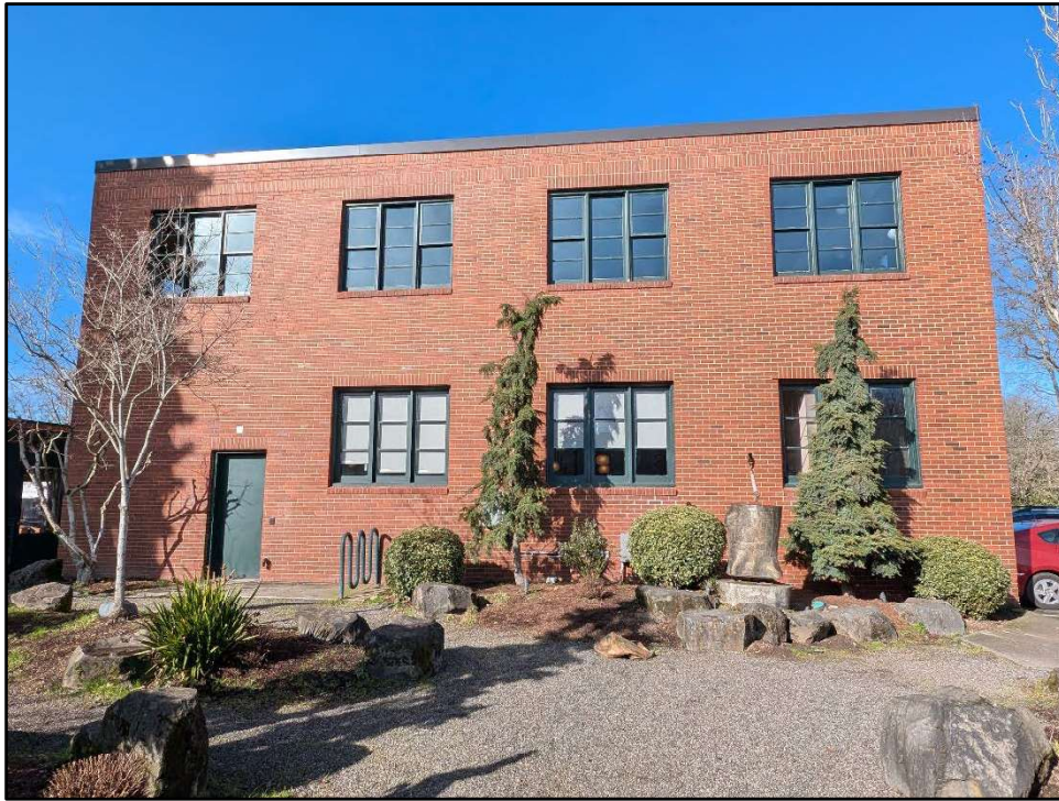
Photo 5 of 20: OR_ClackamasCounty_MilwaukieCityHall_0005 South Elevation, camera facing north
