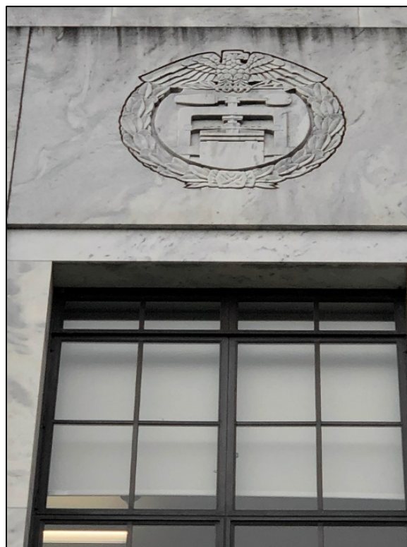
Photo 4 of 16 - OR_MarionCounty_StateLibrary_0004; seal at center top of east side of State Library building shows mission printing press, facing west
