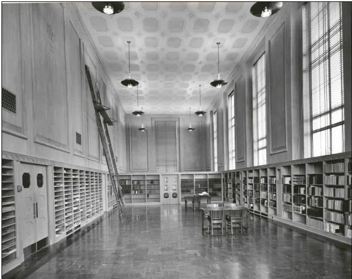
Figure 19 – Construction of State Library, reference room, February 19, 1939, shows ladder for installation of stenciled printers’ marks and cast bronze clock on panels, south side of reference room. Windows are on north side; government documents room is at west end of room behind doors with octagonal bronze grills. Three carved wood panels between shelving units on north side illustrate printing press, meadow lark, and Oregon grape.
