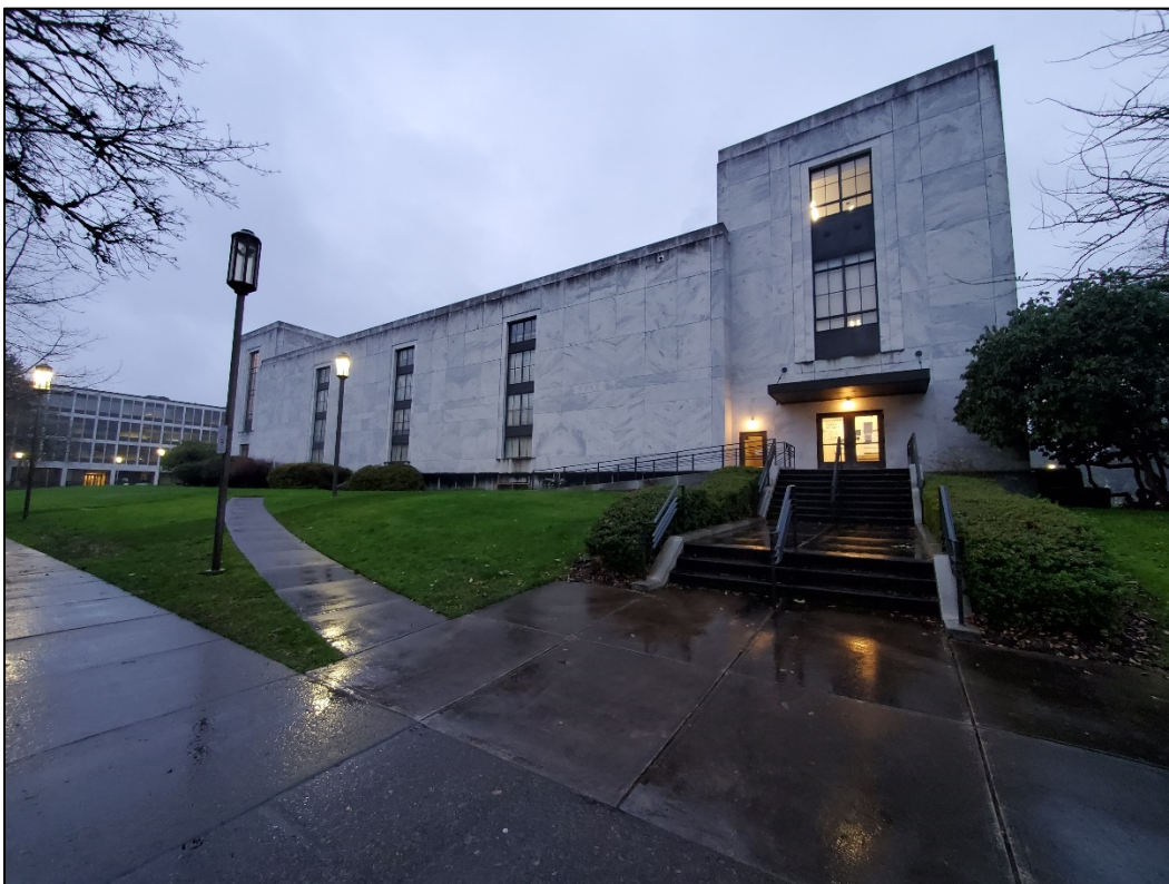
Photo 8 of 16 - OR_MarionCounty_StateLibrary_0008; west side of building showing altered door and canopy with public entrance from Winter Street, facing east
