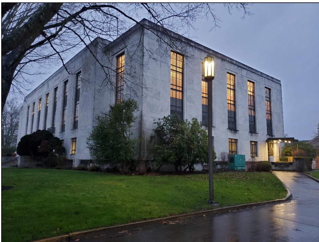
Photo 2 of 16 - OR_MarionCounty_StateLibrary_0002; State Library northeast corner of building, facing southwest
