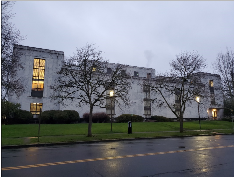
Photo 3 of 16 - OR_MarionCounty_StateLibrary_0003; state library southwest corner of building, facing northeast
