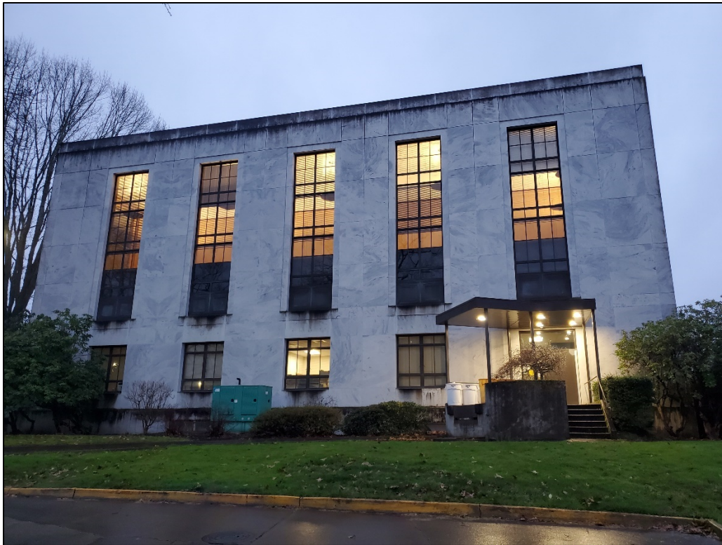
Photo 7 of 16 - OR_MarionCounty_StateLibrary_0007; State Library north side, loading dock on west corner result of alteration, landscaping includes several trees identified on the State Capitol State Park walking tour: Dove Tree ( Davidia involucrata ) and Northern Red Oak ( Quercus rubra ), facing south
