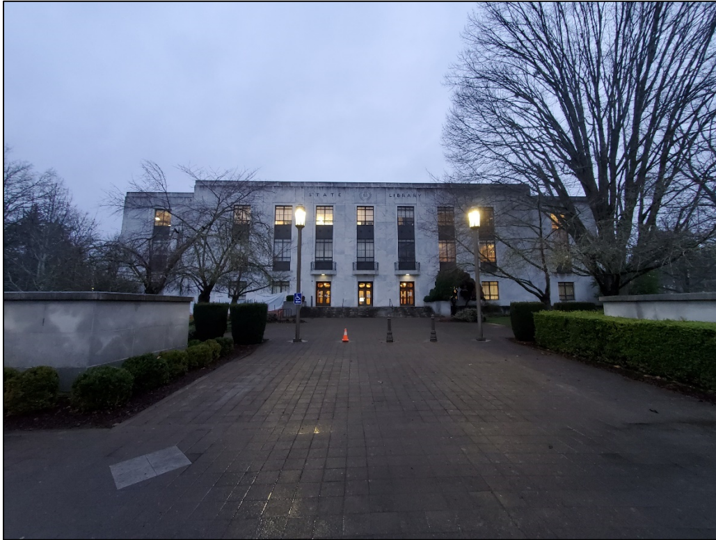
Photo 1 of 16 – OR_MarionCounty_StateLibrary_0001; State Library and setting, facing west
