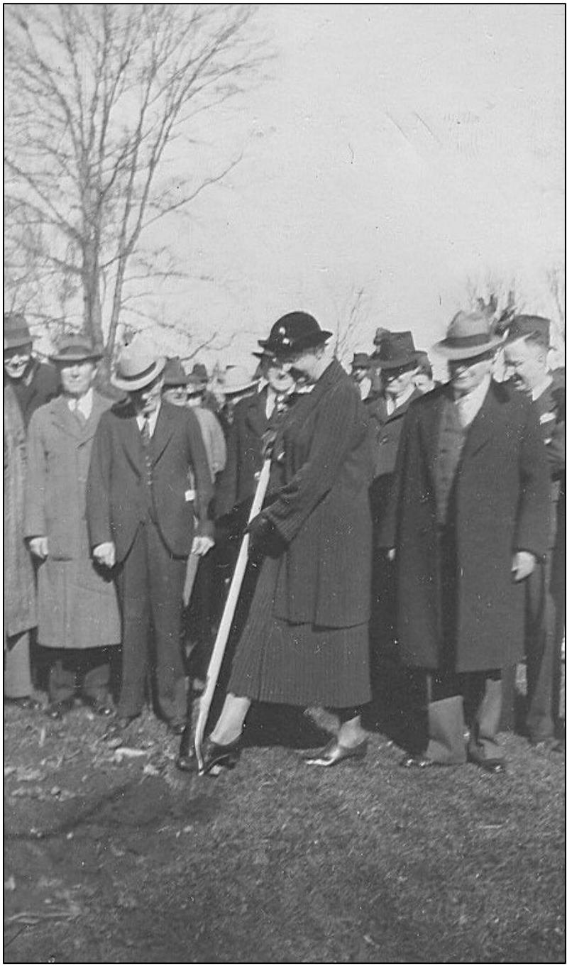
Figure 12 – Groundbreaking photo shows librarian Harriet Long breaking ground for new State Library on February 24, 1938. Governor Charles Martin looking on. Photo that appeared in Oregonian on February 25 showed Governor Martin with spade.
