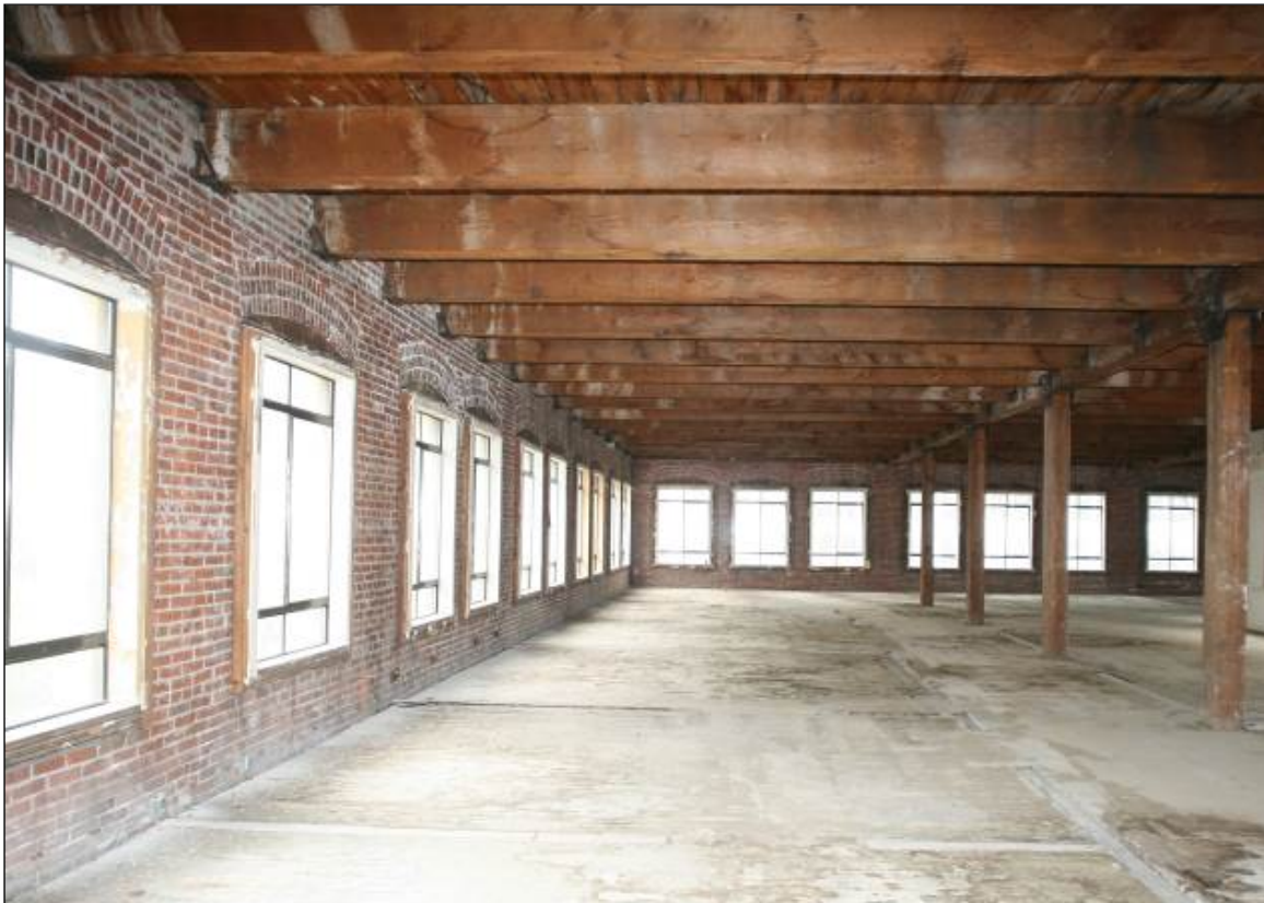
Photo 14 of 14: Interior view, fourth floor, looking west, typical.
