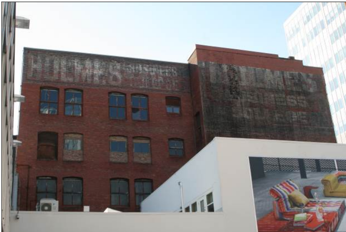
Photo 8 of 14: Exterior view, west elevation, looking east
