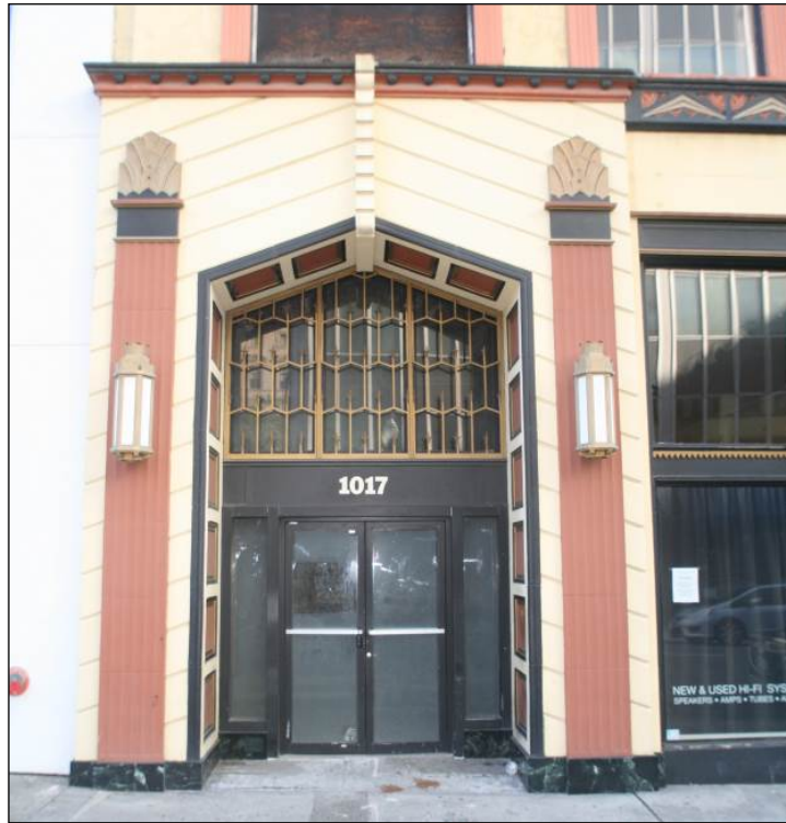
Photo 3 of 14: Exterior view, south elevation, entry at west, looking north.
