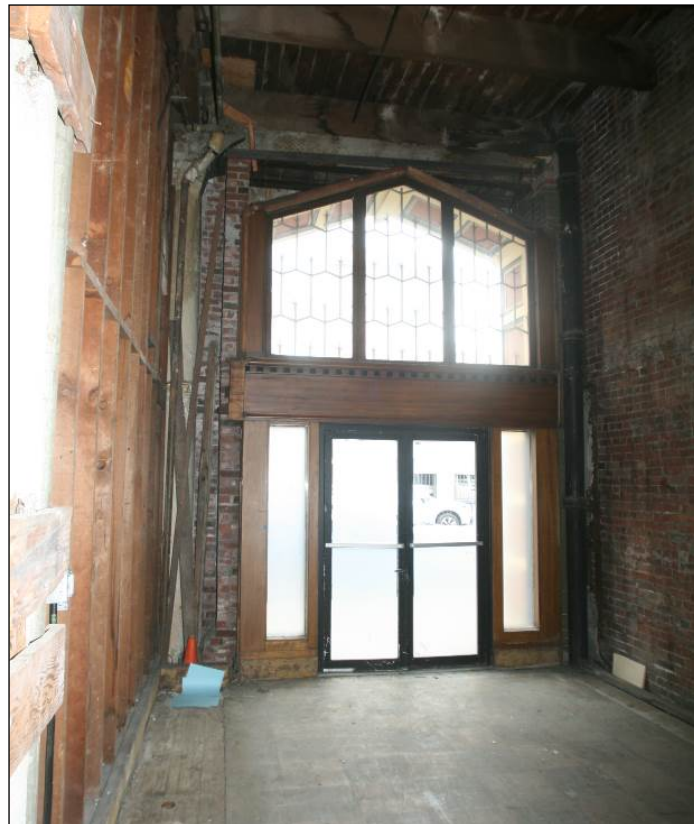
Photo 10 of 14: Interior view, first floor, lobby, looking south.
