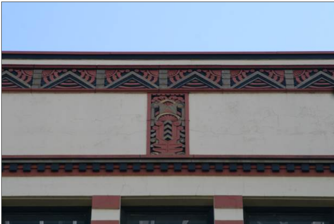
Photo 6 of 14: Exterior Detail, south elevation, looking north, decorative Zig-Zag cornice (typical)
