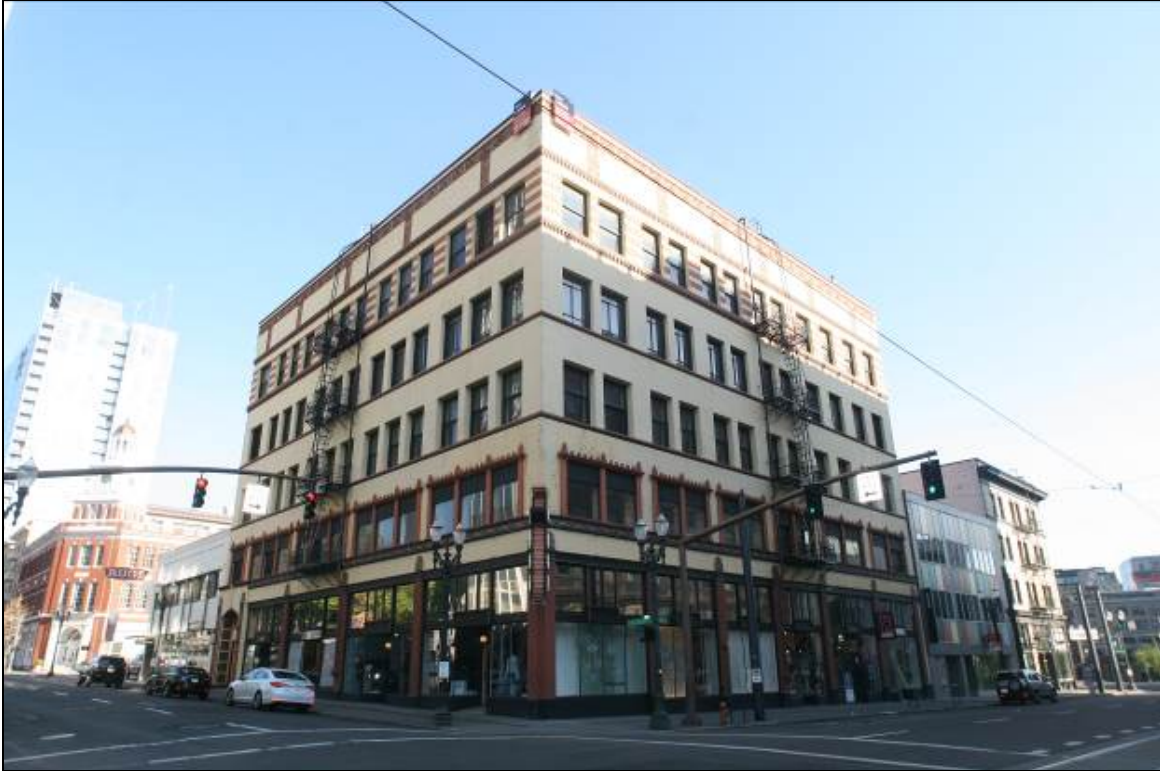
Photo 1 of 14: Exterior view, south and east elevations, looking northwest
