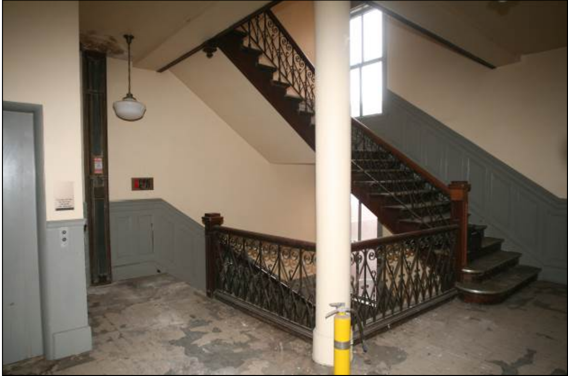
Photo 13 of 14: Interior view, second floor, elevator/stair lobby, looking northwest
