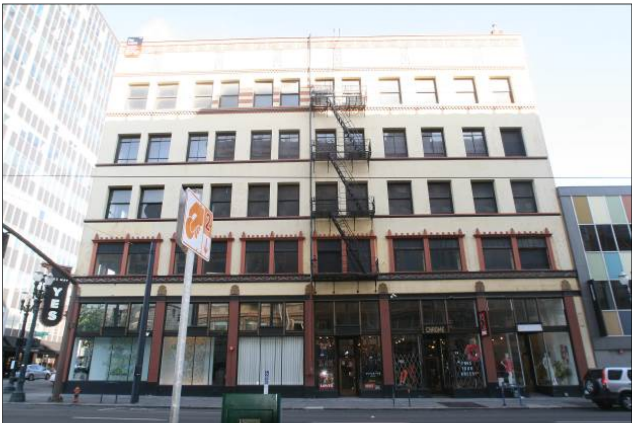
Photo 4 of 14: Exterior view, east elevation, looking west
