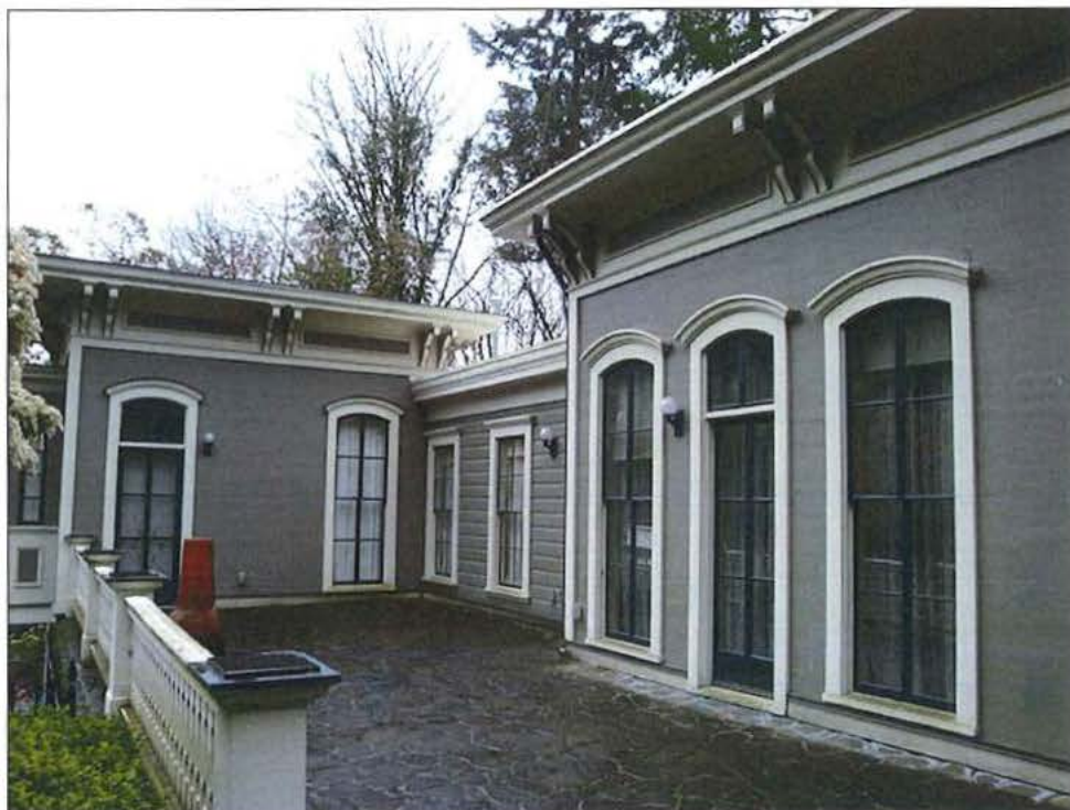
Photo 6 of 17: View of north side with original circa-1865 house (right), circa-1885 addition (center), and 1965-1966 addition (left), view looking east.
