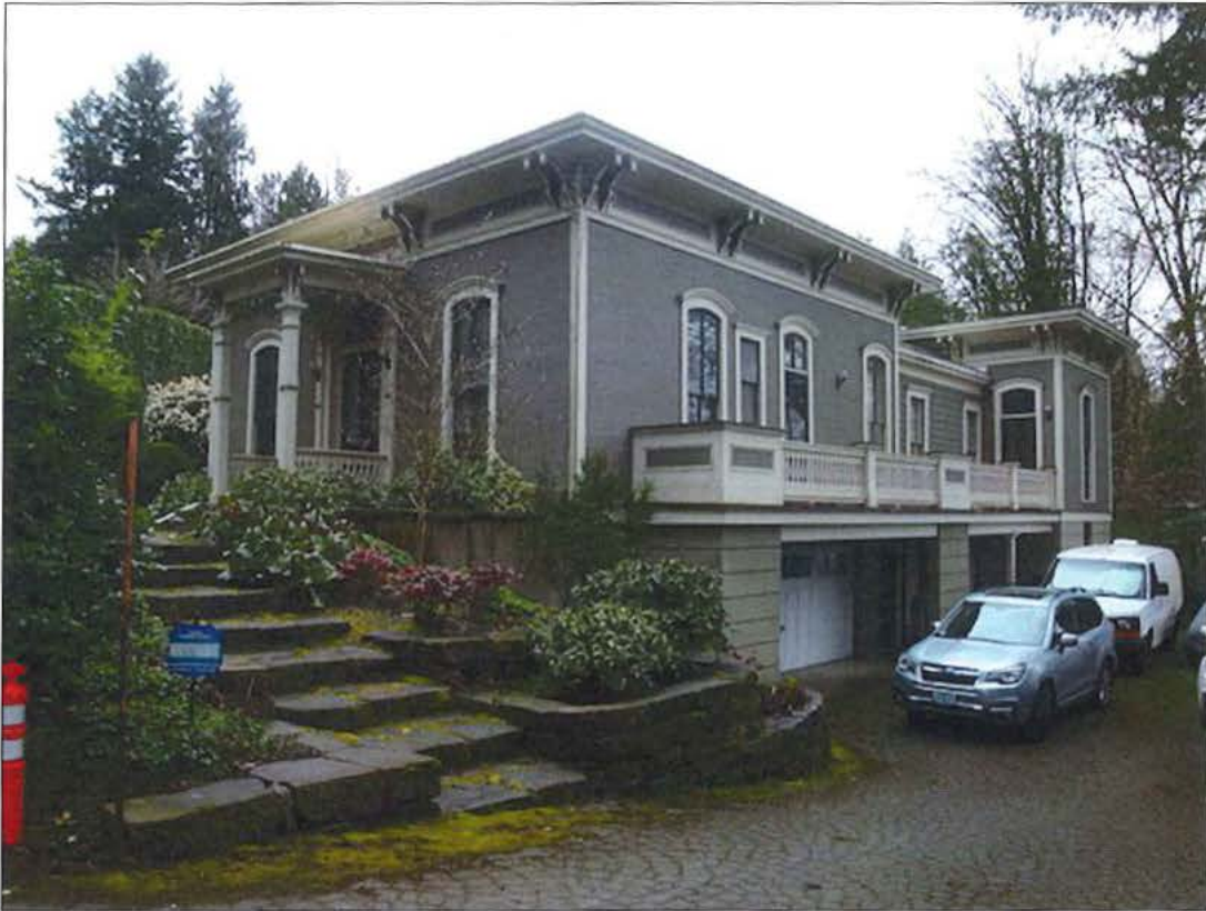
Photo 1 of 17: View of southwest corner, looking northeast from S.W. Cheltenham Court.
