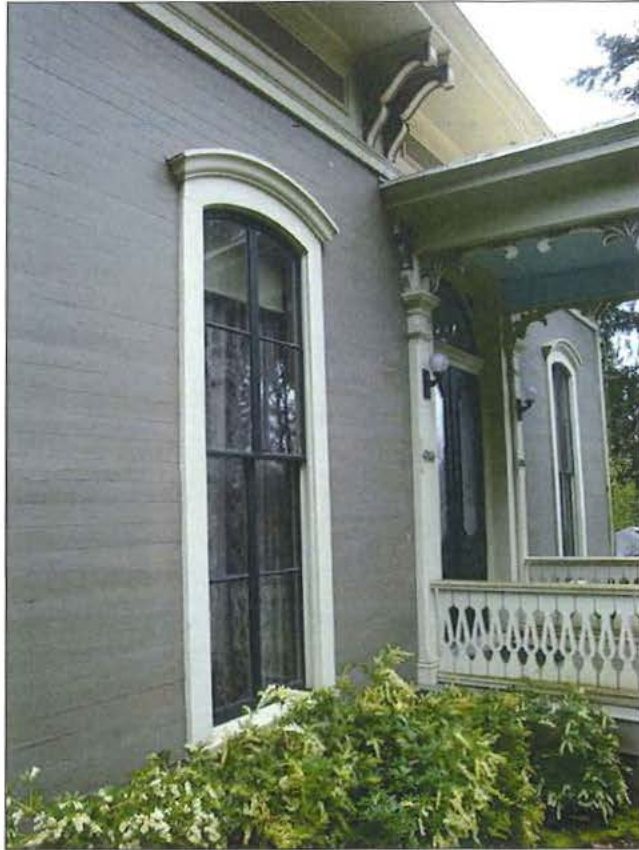
Photo 5 of 17: Detail of front (west) façade showing siding, window, porch, and eave details, looking southeast.
