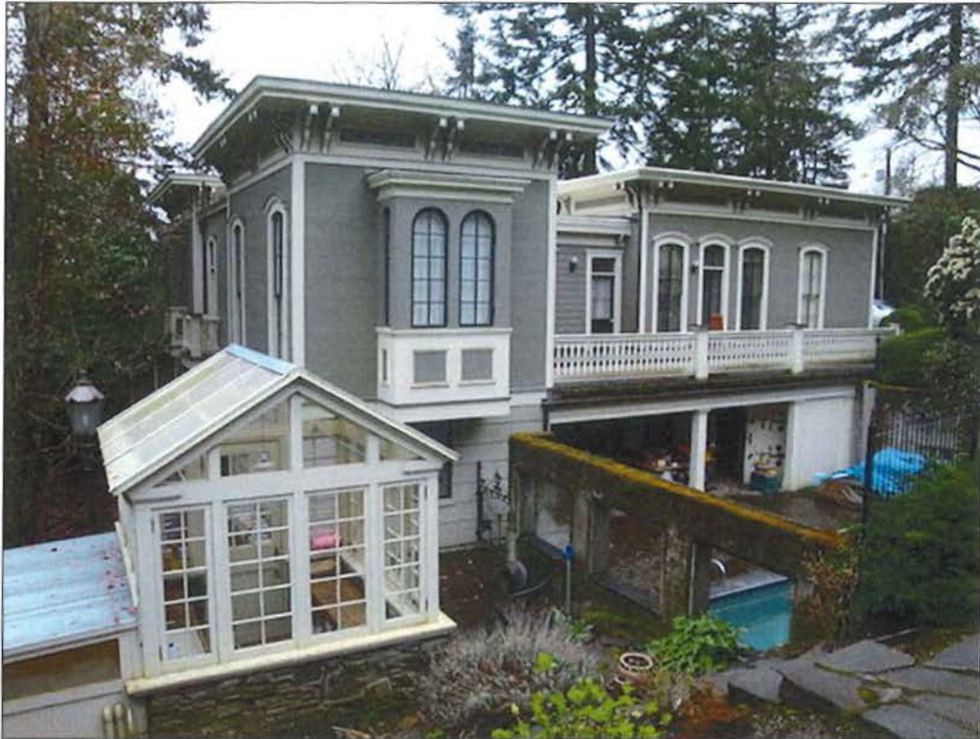
Photo 3 of 17: North elevation view, with greenhouse, remnant foundation wall, and section of salvaged iron fencing, view looking south/southwest.
