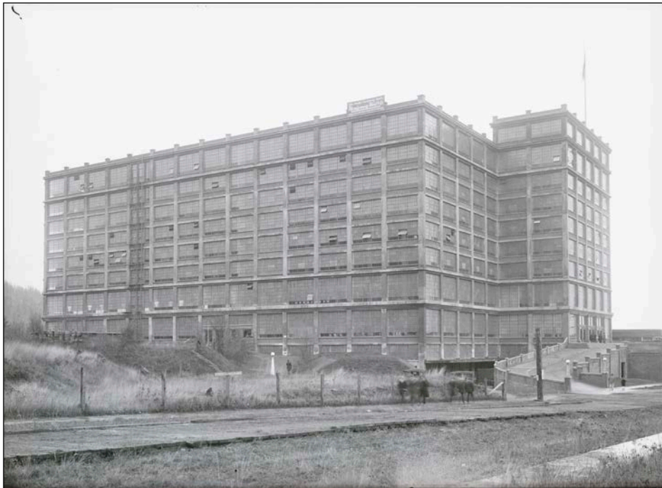
Figure 10a. South and East Elevations, Looking Northwest, September 1920
