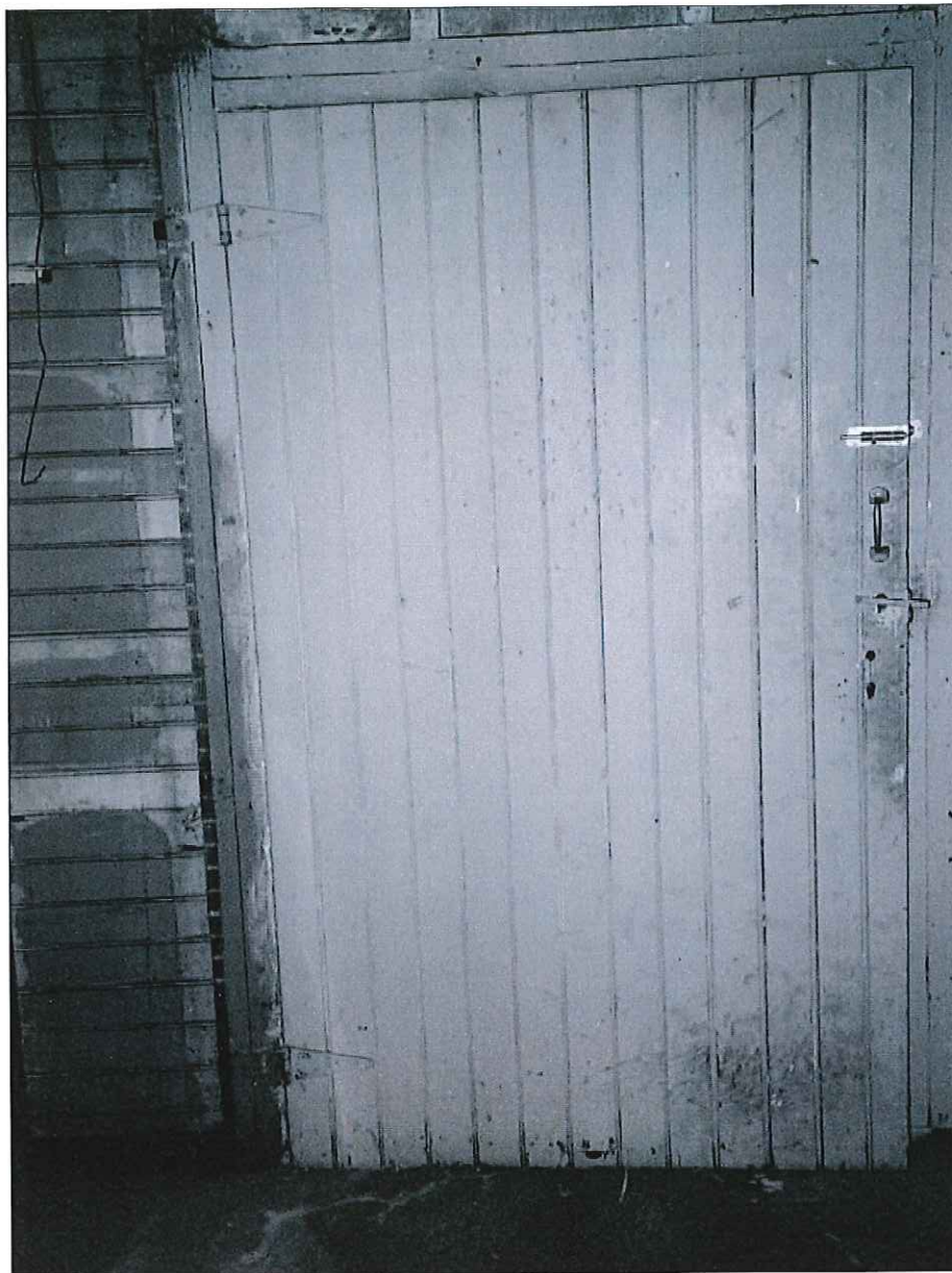
Photo 11 of 15: Basement, 1929 door to garage
