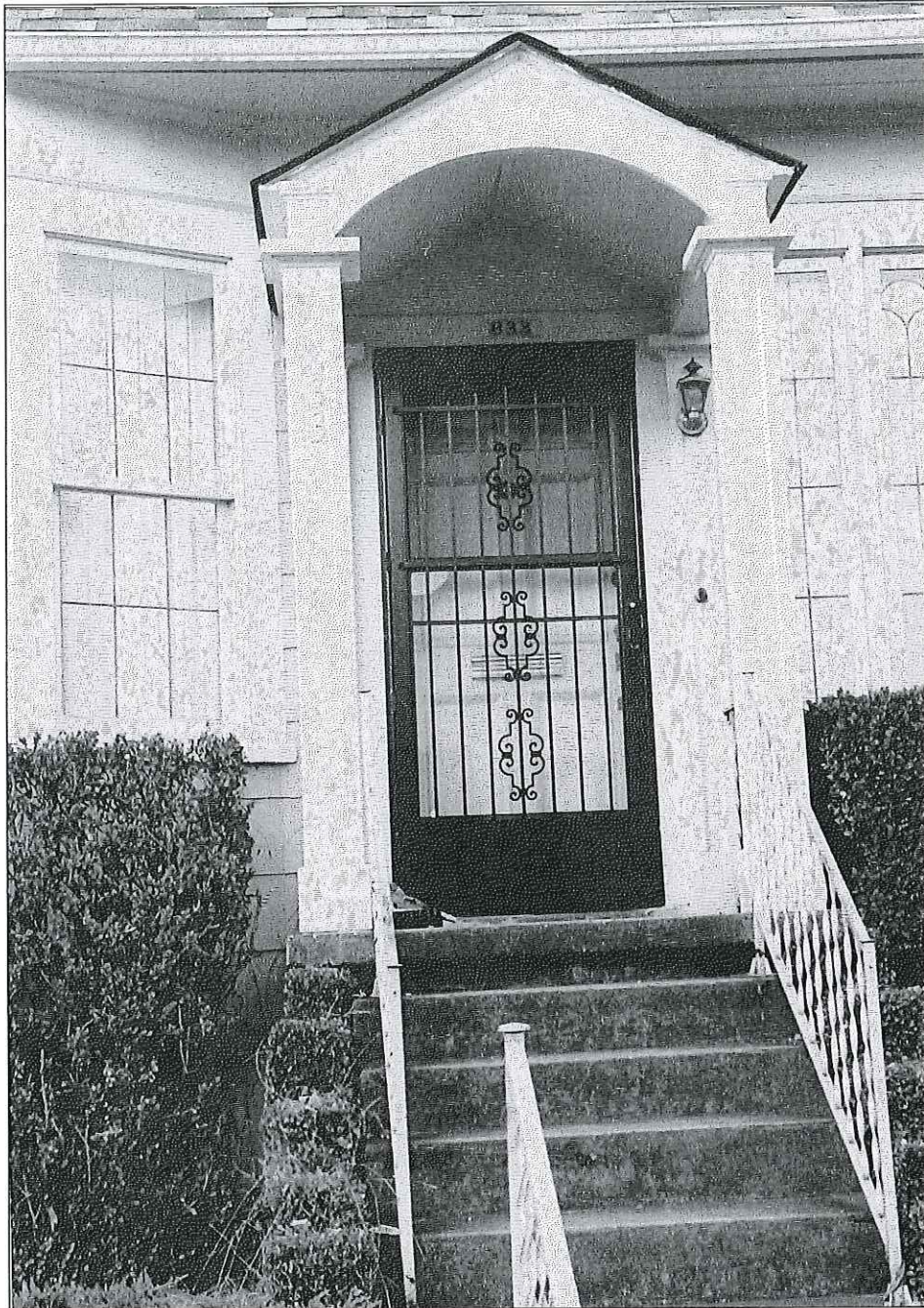
Photo 2 of 15: Main (south) entry façade
