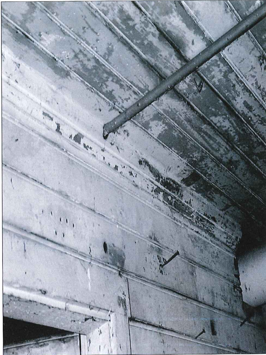
Photo 12 of 15: Basement – garage wall, ceiling
