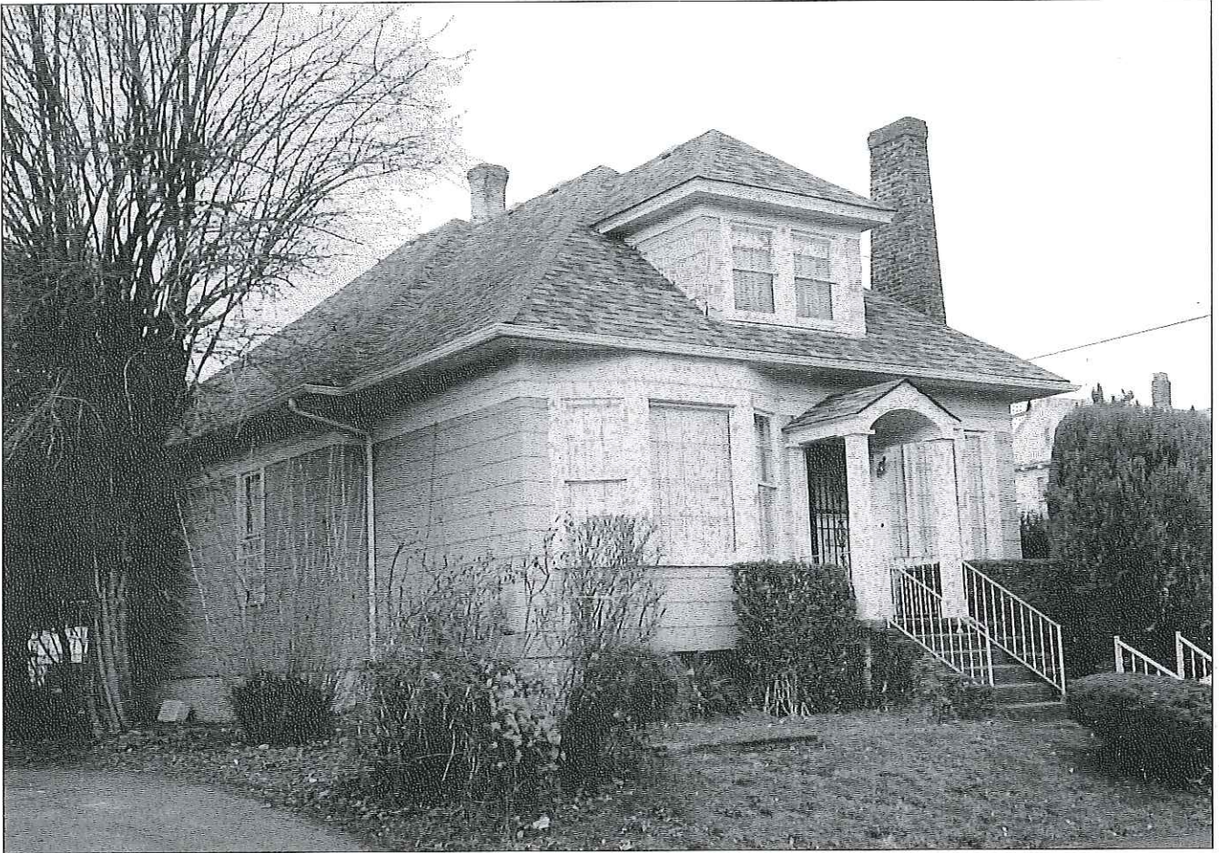
Photo 1 of 15: Main (south) façade and portion of west façade
