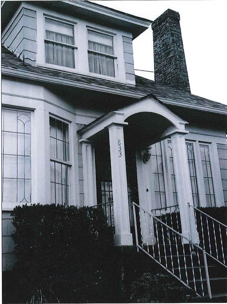
Photo 5 of 15: Main (south) elevation – entry porch and windows
