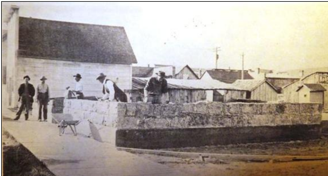
Figure 4: Historic Photo, Wallowa County Chieftain Building under construction, Autumn 1915, Chieftain Files, Enterprise, OR.
