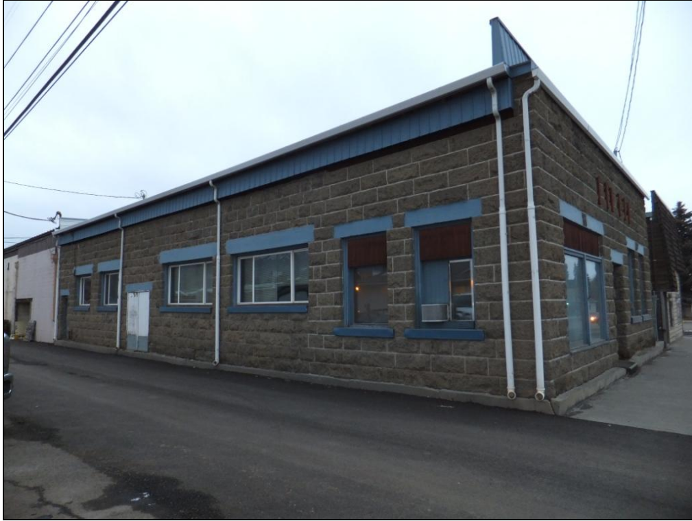
Photo 3 of 11: OR_WallowaCounty_WallowaCoChieftainBuilding_0003 South facade, left, and east façade, right, looking northwest
