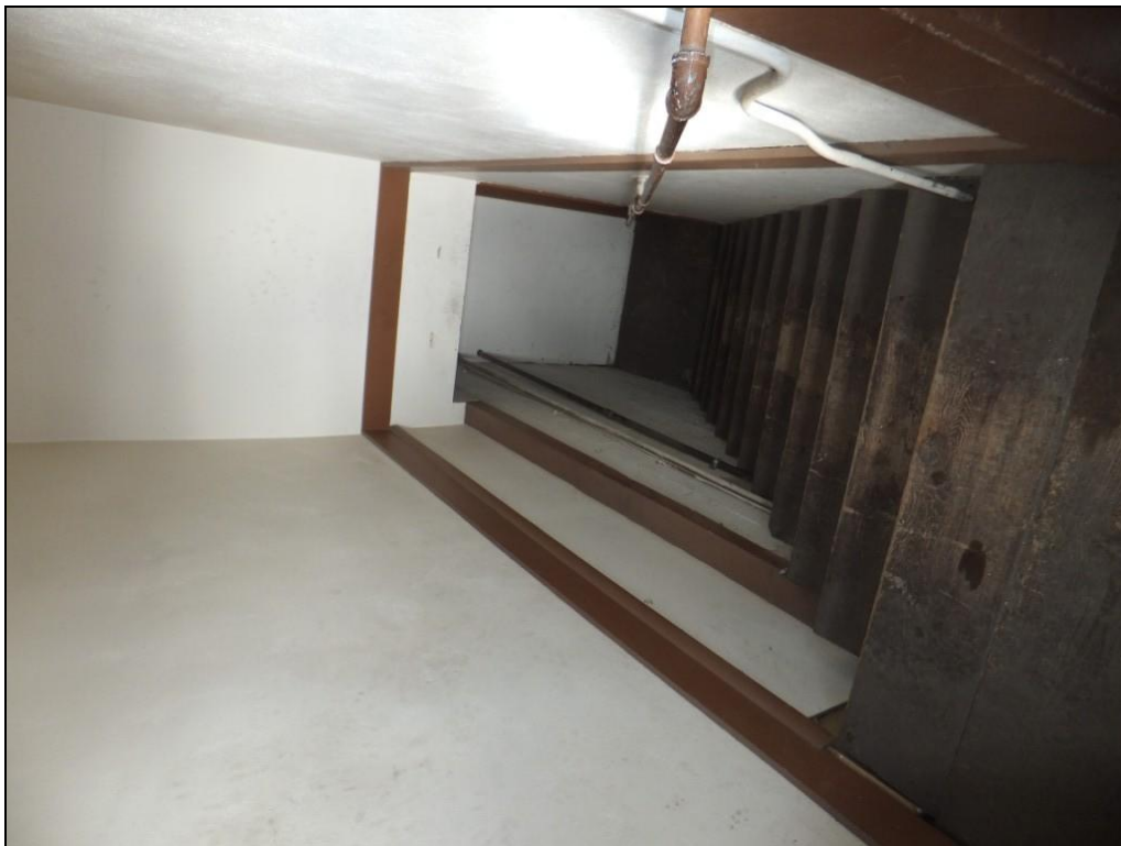
Photo 10 of 11: OR_WallowaCounty_WallowaCoChieftainBuilding_0010 Upstairs landing and stairs to the basement, looking north
