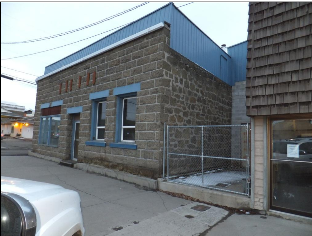
Photo 2 of 11: OR_WallowaCounty_WallowaCoChieftainBuilding_0002 North facade, right, and east facade, left, looking southwest
