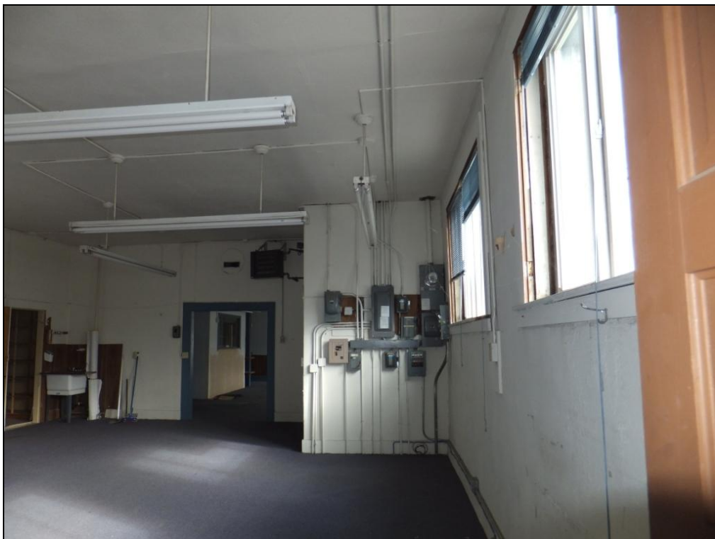
Photo 8 of 11: OR_WallowaCounty_WallowaCoChieftainBuilding_0008 Job Room, looking east from west stairs
