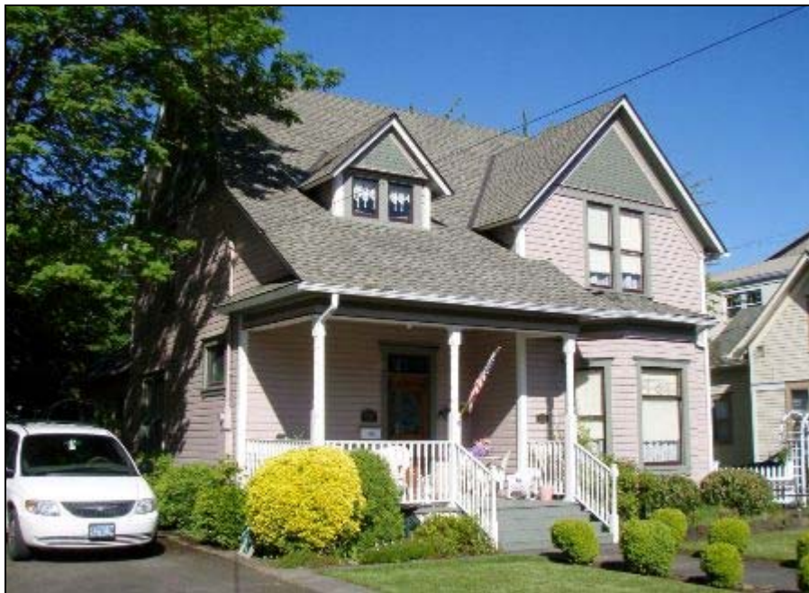
Photo 2 of 16: OR_MarionCounty_JuneDrakeHouse_0002 North, west half (left) and west (right) elevations, view to the east.
