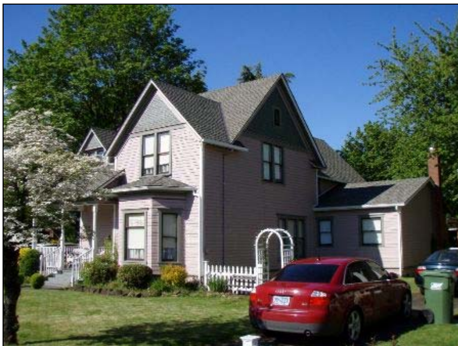
Photo 3 of 16: OR_MarionCounty_JuneDrakeHouse_0003 West (left) and south (right) elevations. View to the north.
