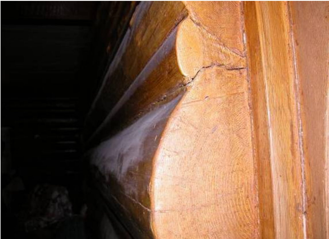
Photograph 8 of 12 Main House-Interior detail of quarter-round chinking in dining room
