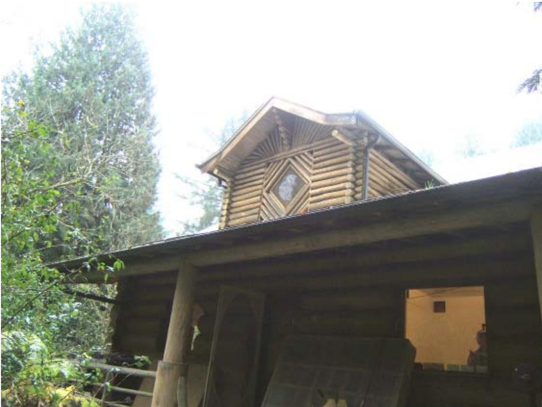
Photograph 4 of 12 Main House-North elevation
