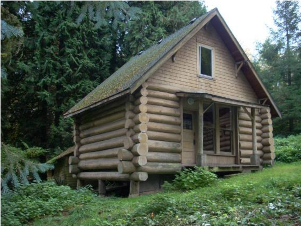
Photograph 11 of 12 Guesthouse-North and east elevations
