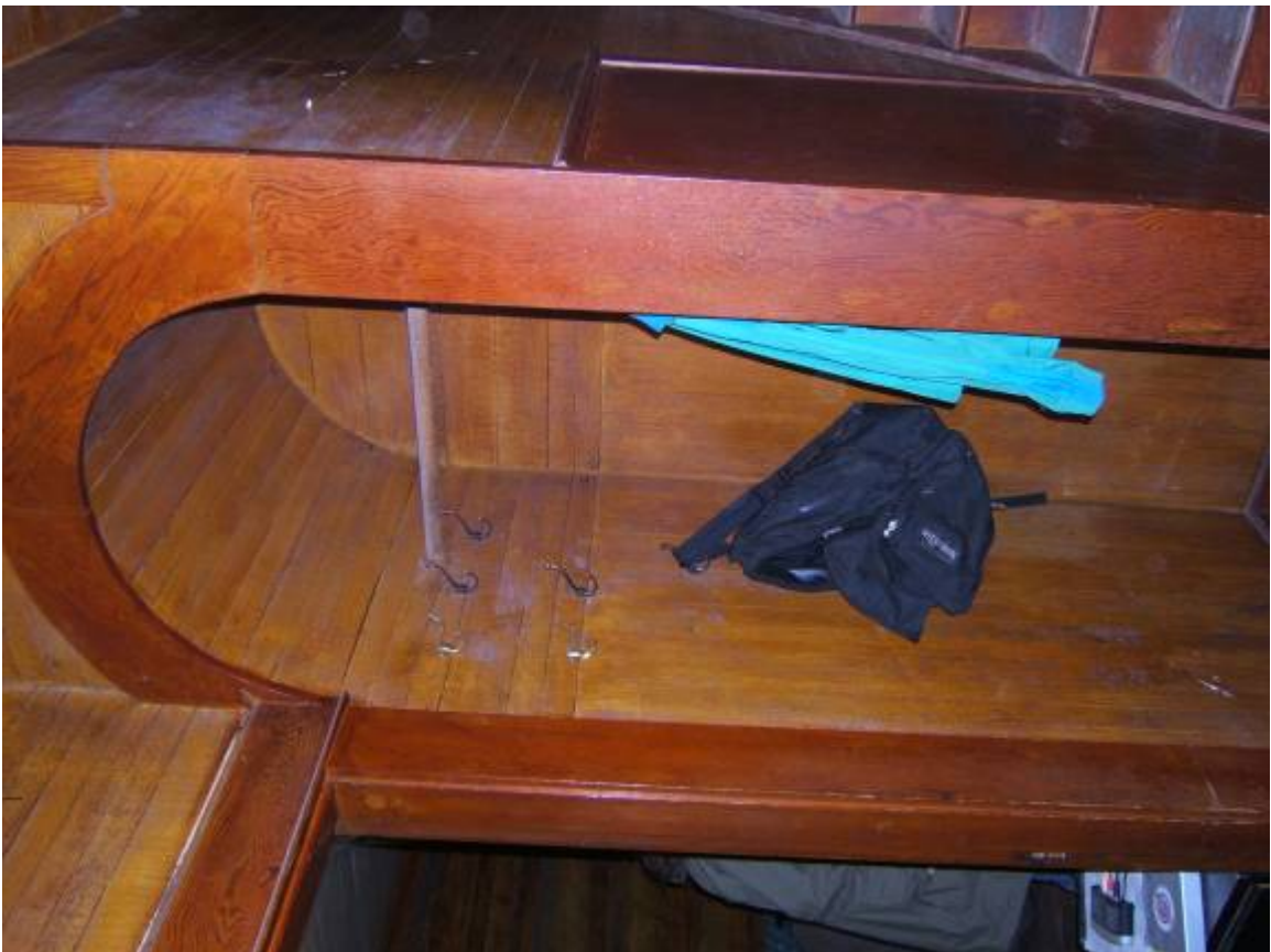
Photograph 6 of 12 Main House-Interior view of barrel vaulted closet near main entryway
