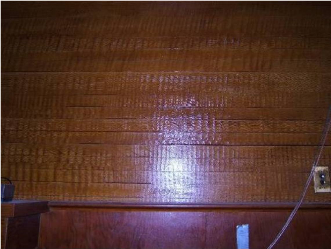
Photograph 9 of 12 Main House-Interior view of faux-grained woodwork in dining room
