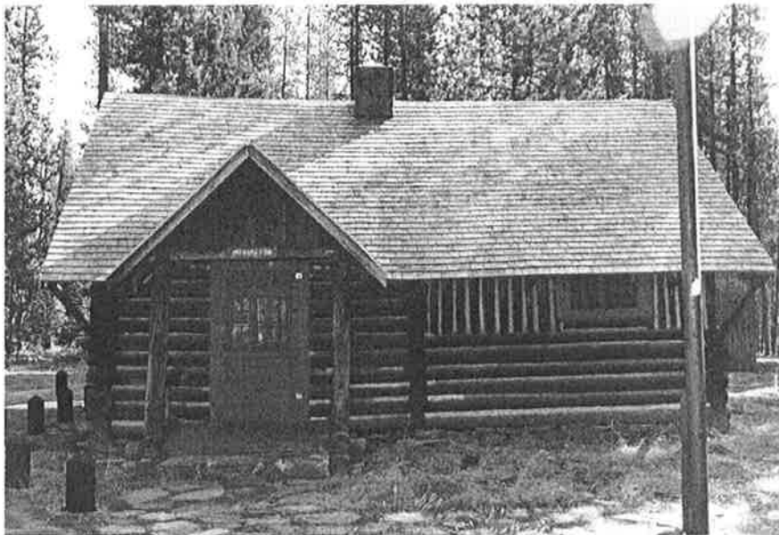
2 of 20: Exterior view, west (front) facade. View to east.
