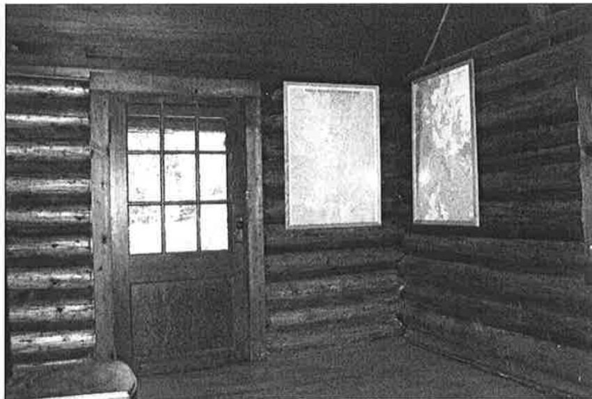
10 of 20: Interior view, guard station, front room. View to west.
