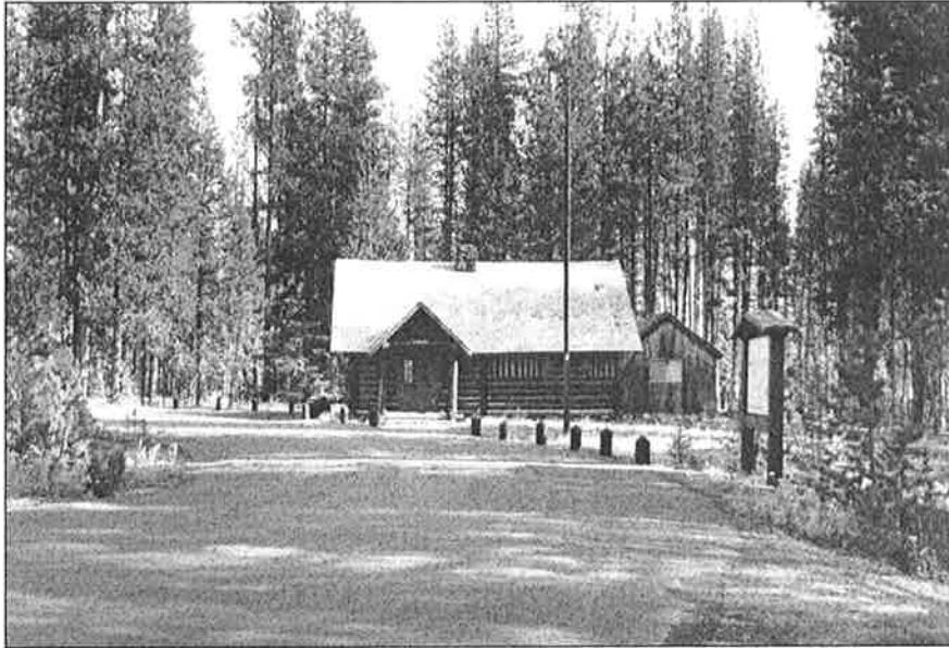
1 of 20: Exterior view, Elk Lake Guard Station site and setting. View to east.
