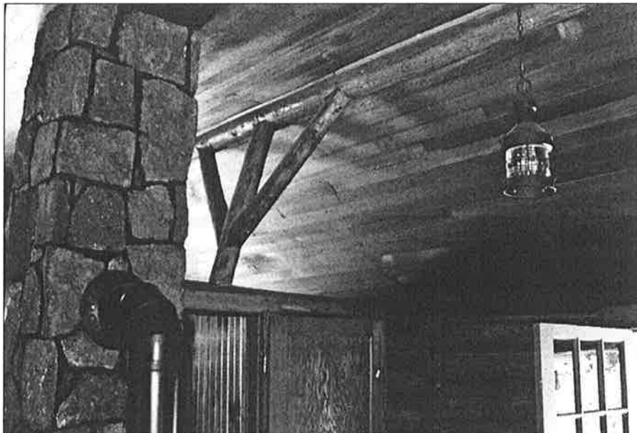
16 of 20: Exterior view, guard station, east roof purlin and bracing.
