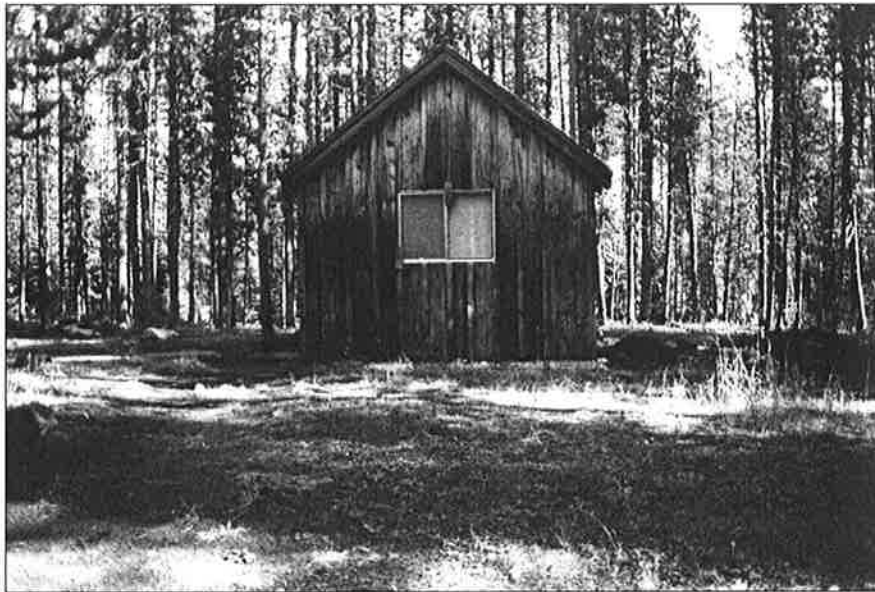
9 of 20: Exterior view, west facade, utility building. View to east.
