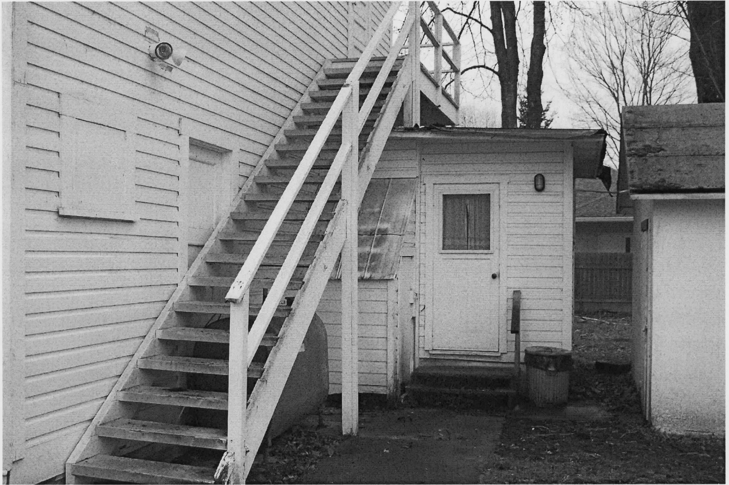
Photo 6 of 12: North elevation showing kitchen addition and detached storage shed, facing west.
