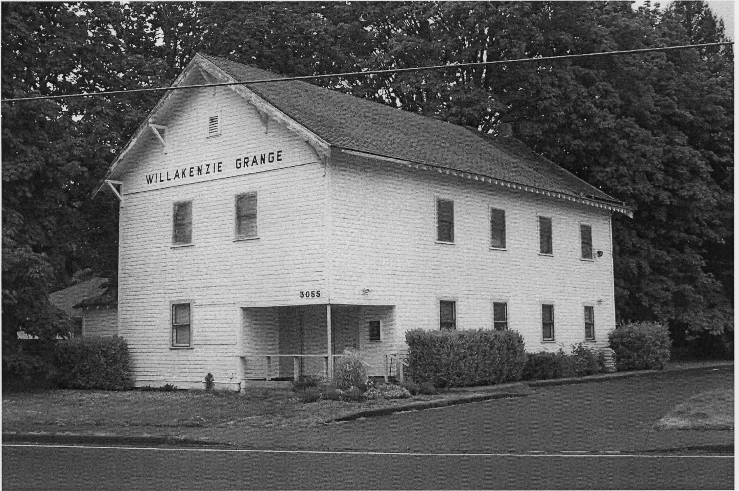
Photo 2 of 12: South and east elevations, facing northwest.
