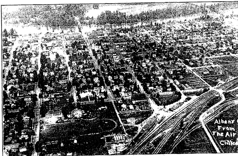
54) Looking north. Remains of demolition of old Albany College shown just above Central field. race track in lower left. Photo taken before construction of Pacific Boulevard. c. 1927
