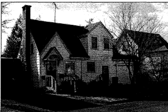
Photo 4: 616 11th Ave. SW, facing South
