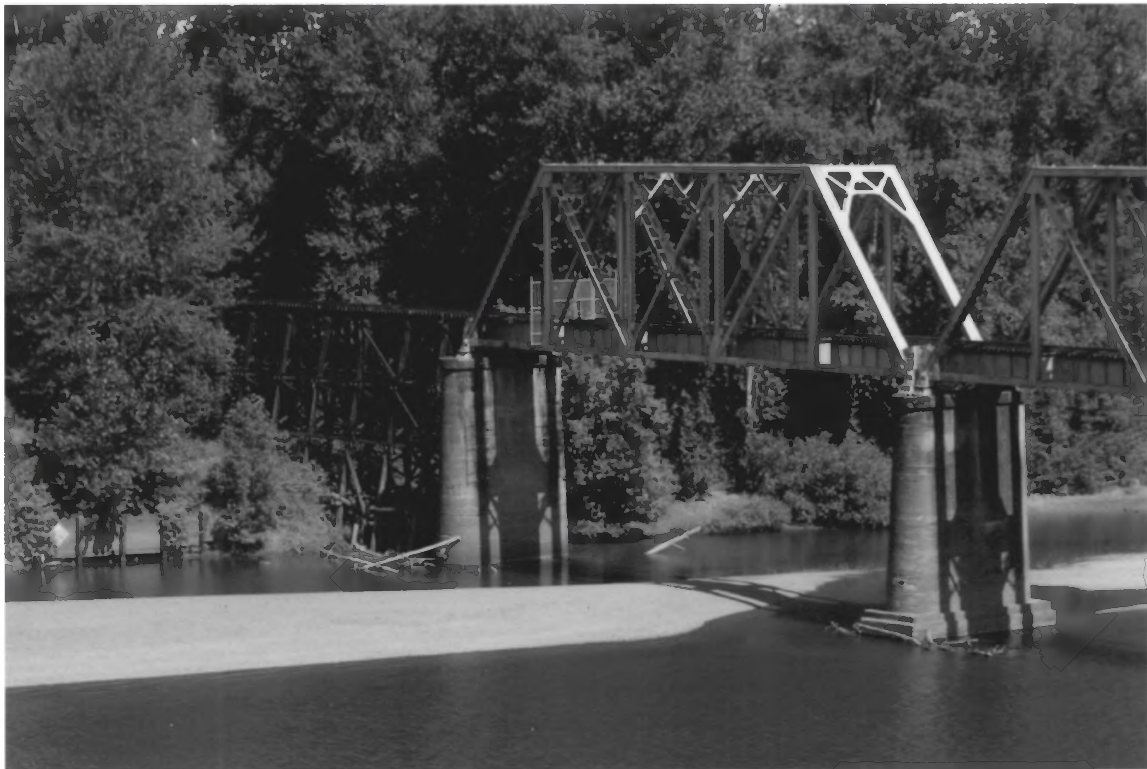
Picture 5. Bridge connection to trestle, looking northwest.
