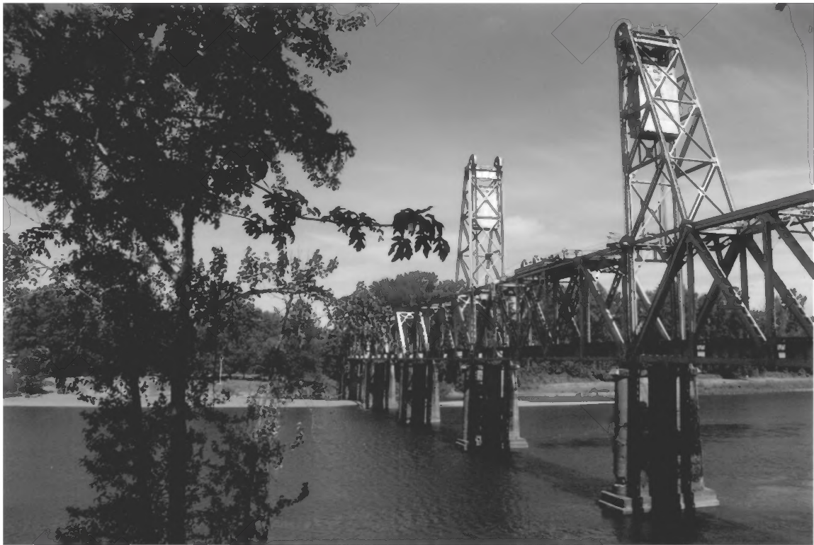
Picture 2. Bridge from east bank, looking northwest.
