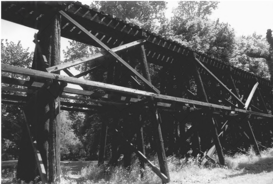
Picture 7. Typical transverse view of trestle, looking northwest.
