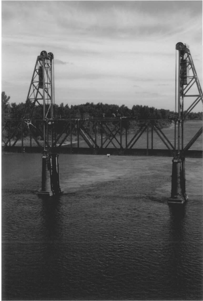
Picture 10. Lift span from Marion Street Bridge, looking north.
