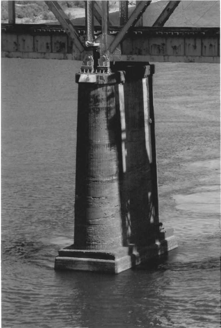
Picture 16. Pier 4, looking north.
