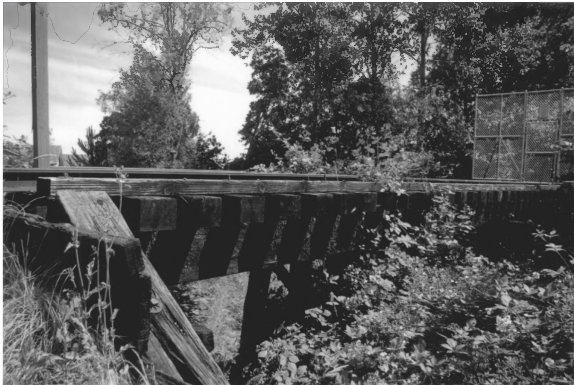
Picture 9. West end of trestle at embankment, looking northwest.
