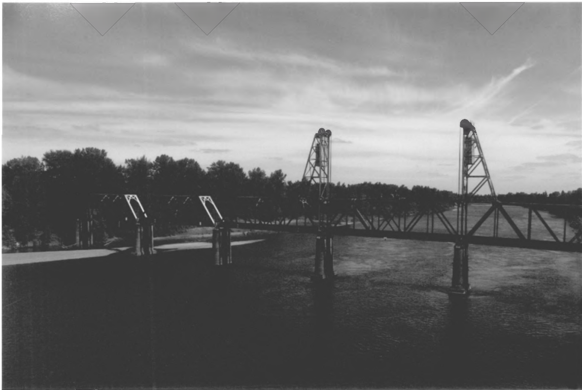
Picture 3. Bridge from Marion Street Bridge (Hwy 22), looking north.
