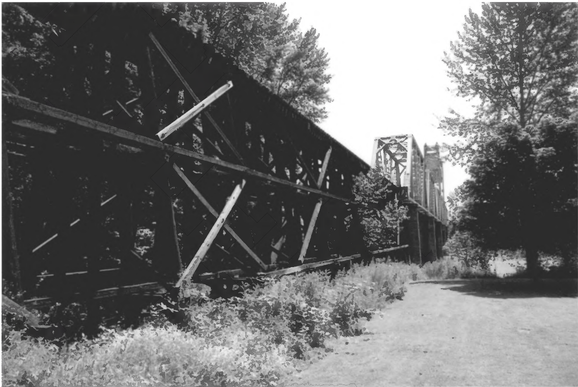
Picture 6. Trestle from park roadway, looking east.
