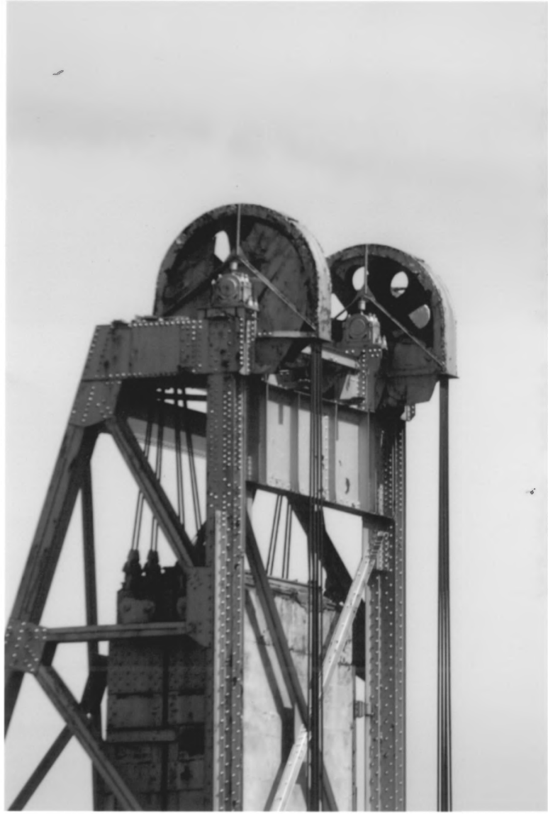
Picture 12. Western lift tower, looking north.
