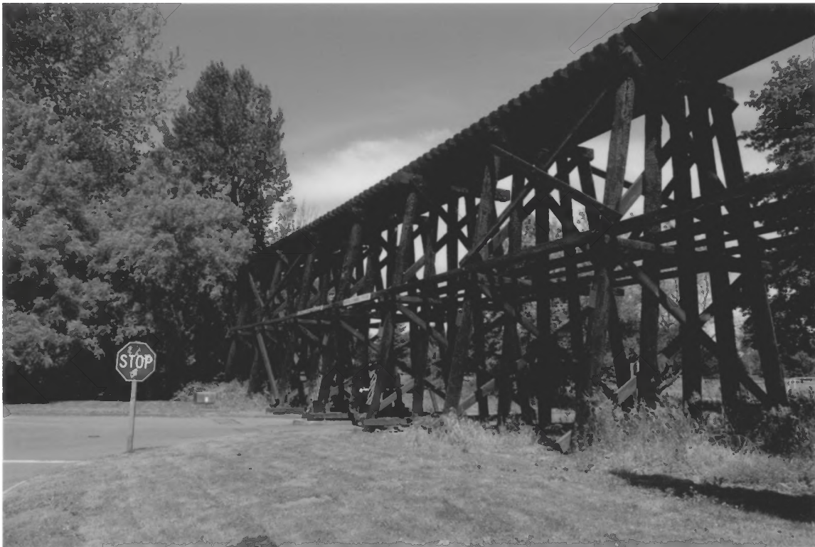
Picture 8. Trestle from park roadway, looking west.
