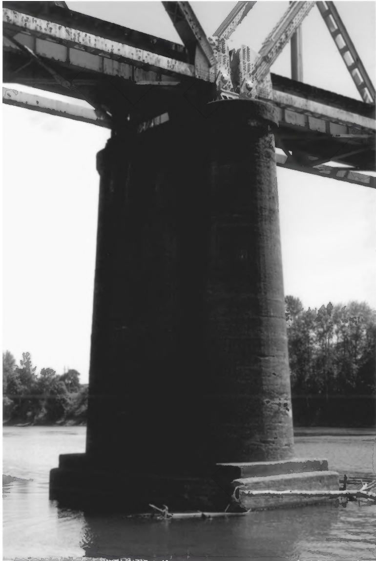
Picture 15. Pier2, looking northeast.
