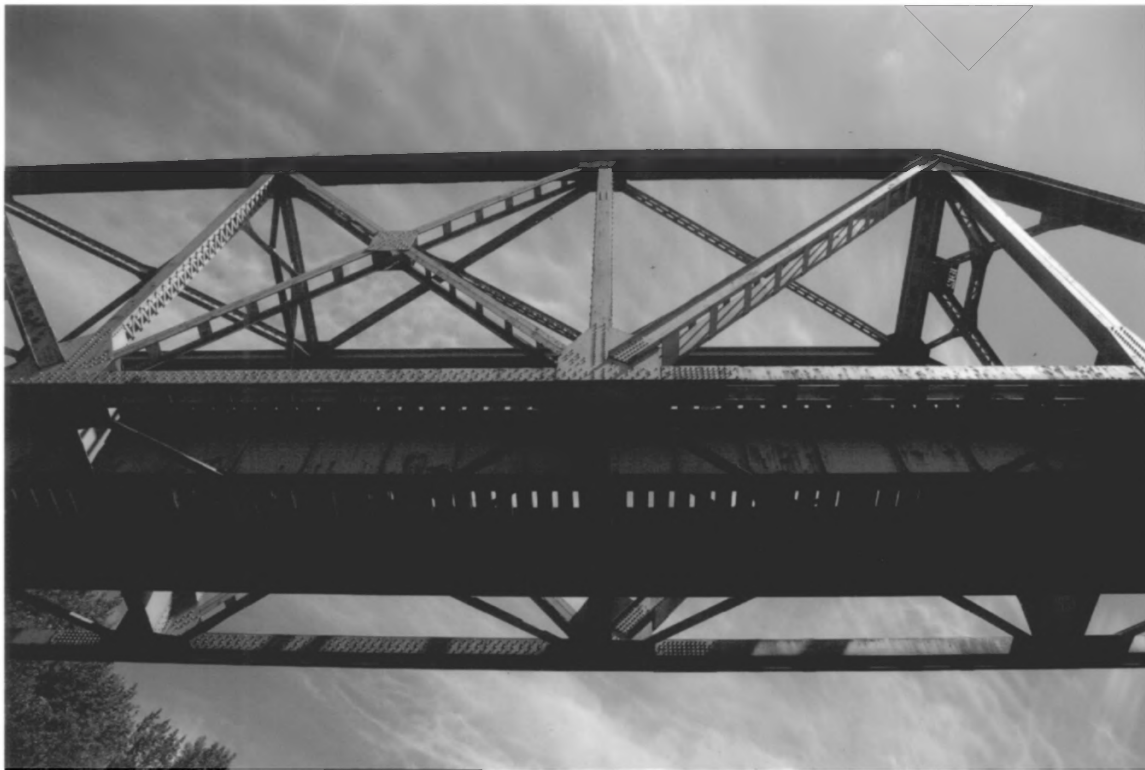
Picture 17. Truss detail, from below.
