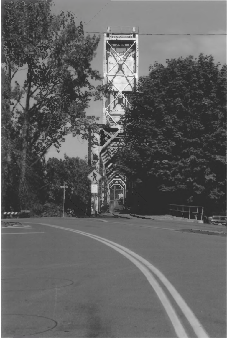
Picture 1. Bridge from centerline of Union Street NE, looking west-northwest.
