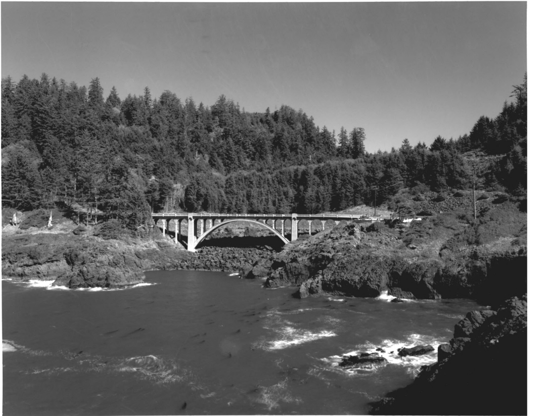
ROCKY CREEK BRIDGE, OTTER ROCK, OREGON
