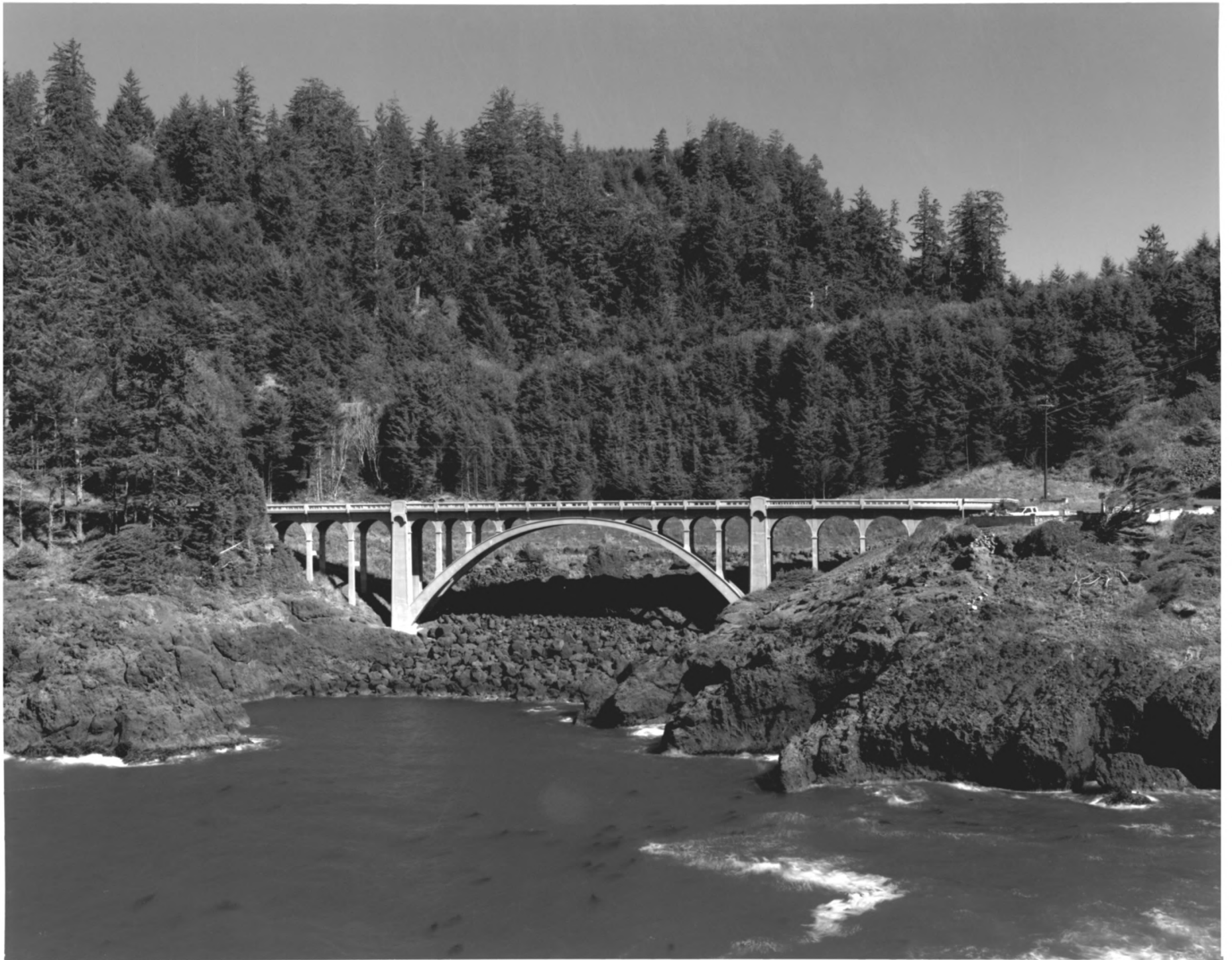
ROCKY CREEK BRIDGE, OTTER ROCK, OREGON #3
