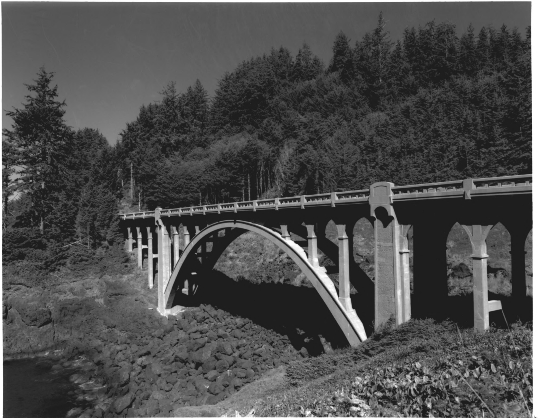
ROCKY CREEK BRIDGE, OTTER ROCK, OREGON #5
