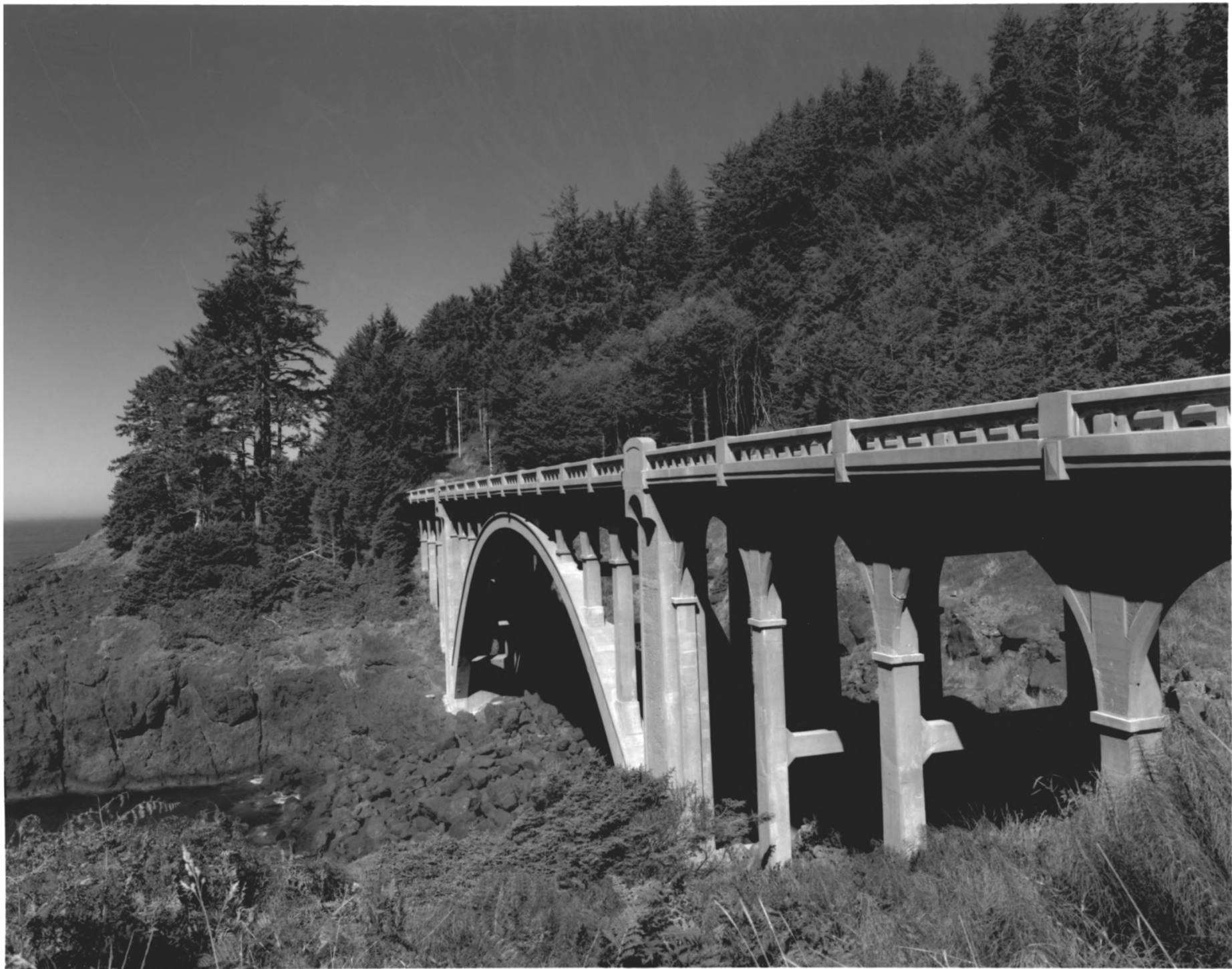
ROCKY CREEK BRIDGE, OTTER ROCK, OREGON # 2
