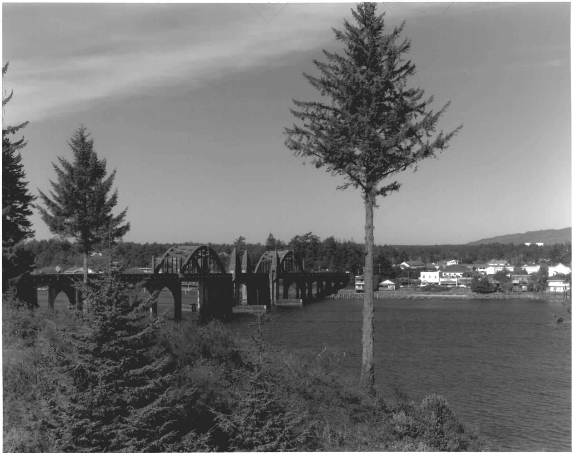
SIOUSLAW RIVER BRIDGE, FLORENCE, OREGON
