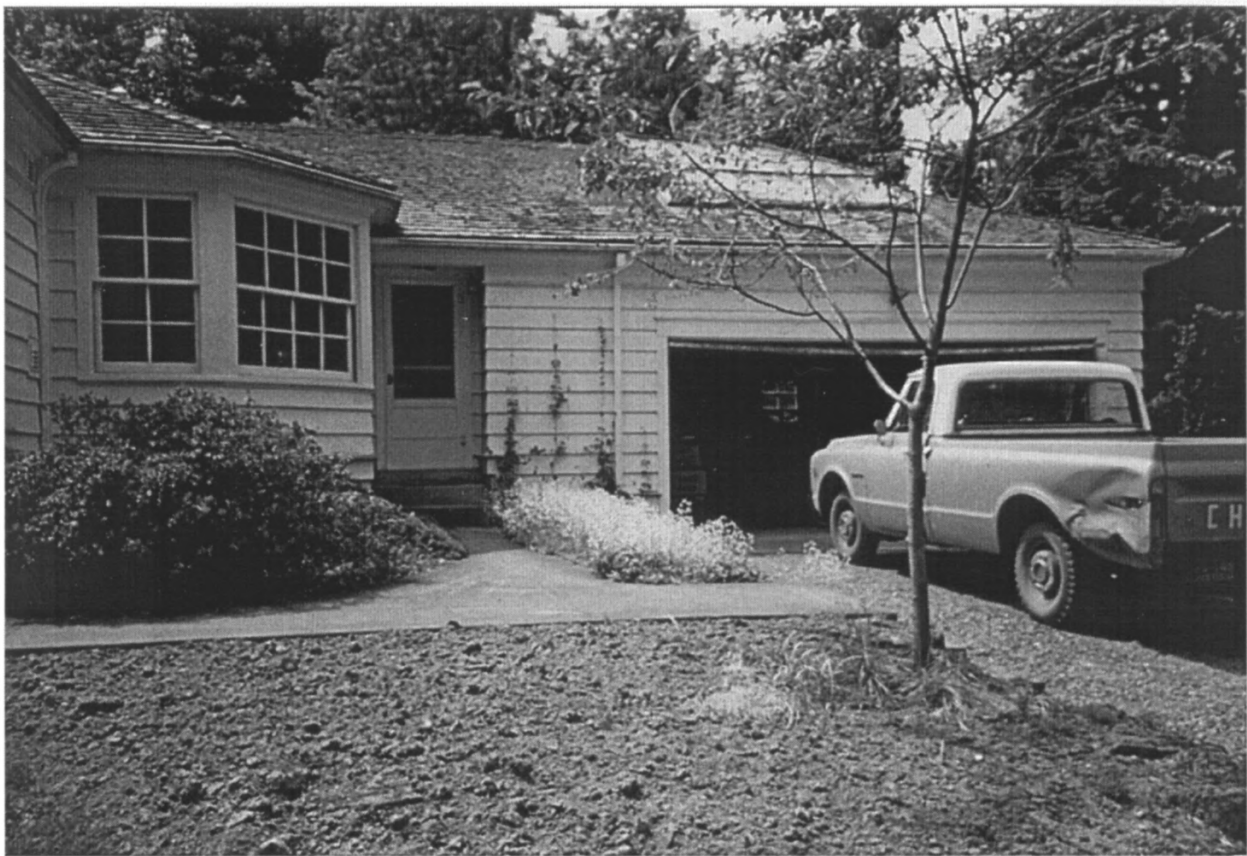
Garage, (demolished), note conservatory built into roof at right, 1982.
