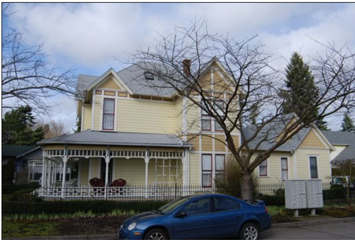
Photo 3 of 14: Southeast elevation of house. View to the northwest.
