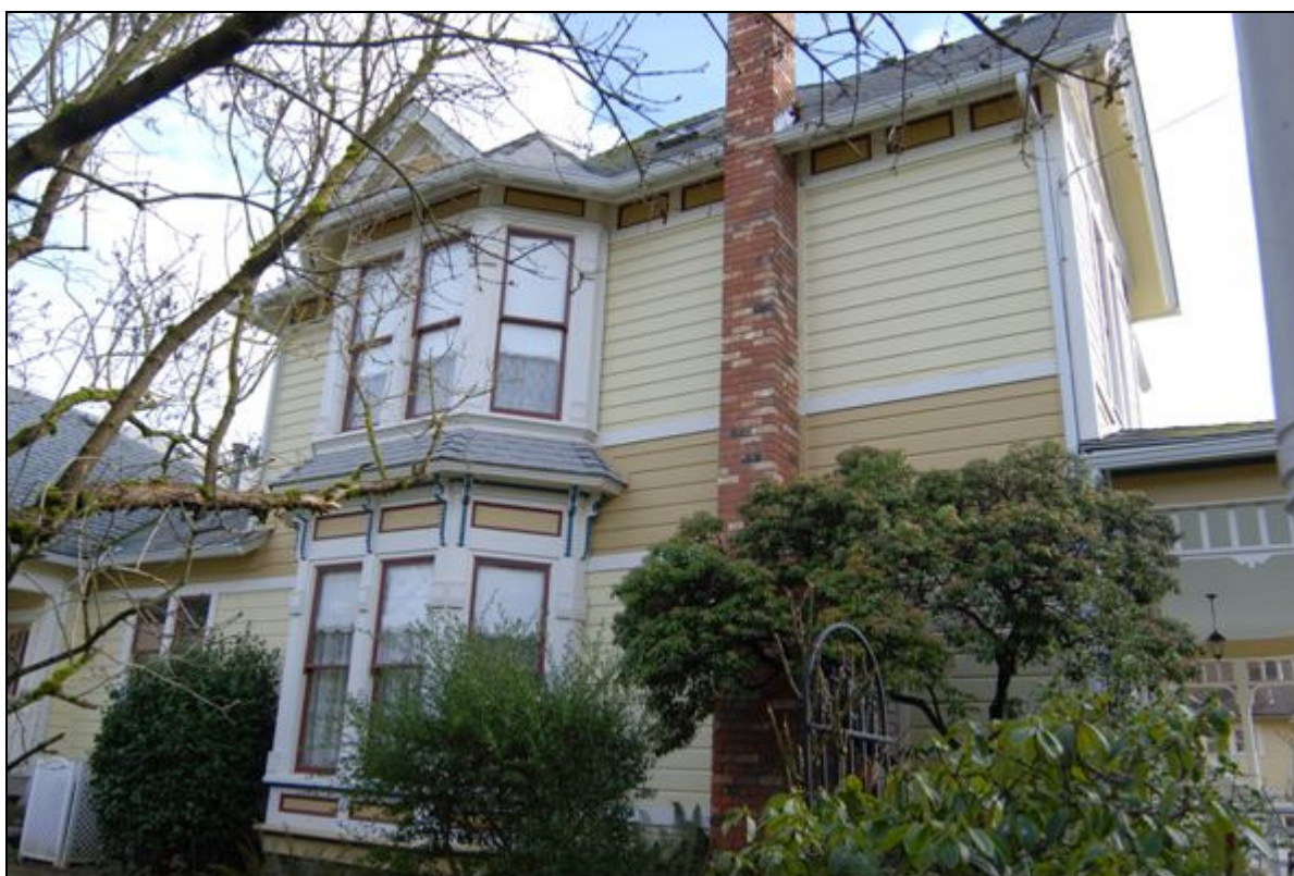
Photo 4 of 14: Northwest elevation of house, view to the east.
