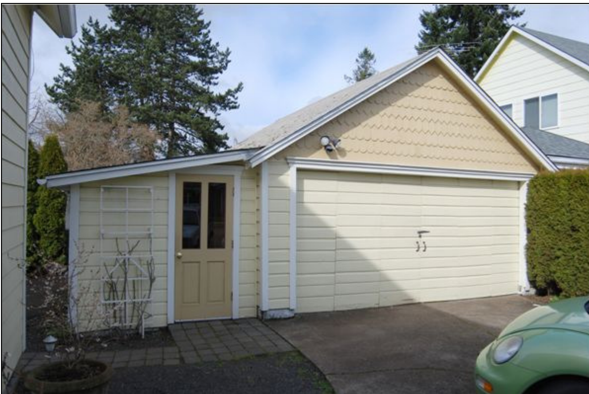
Photo 6 of 14: Southeast elevation of garage, view to the northwest.
