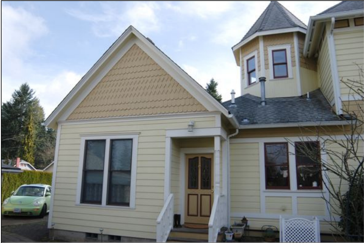
Photo 5 of 14: Northwest elevation of house, rear entry hall door, view to the southeast.
