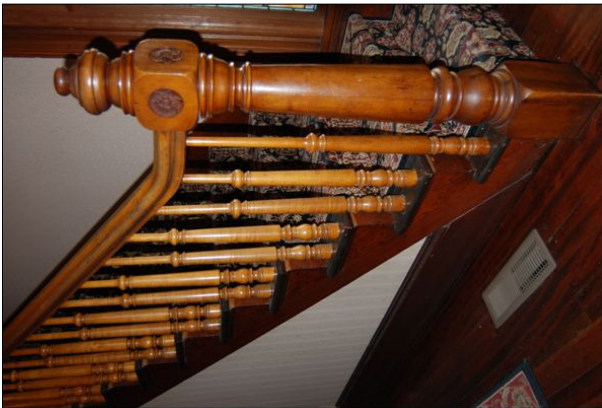
Photo 11 of 14: Balustrade detail view to the east
