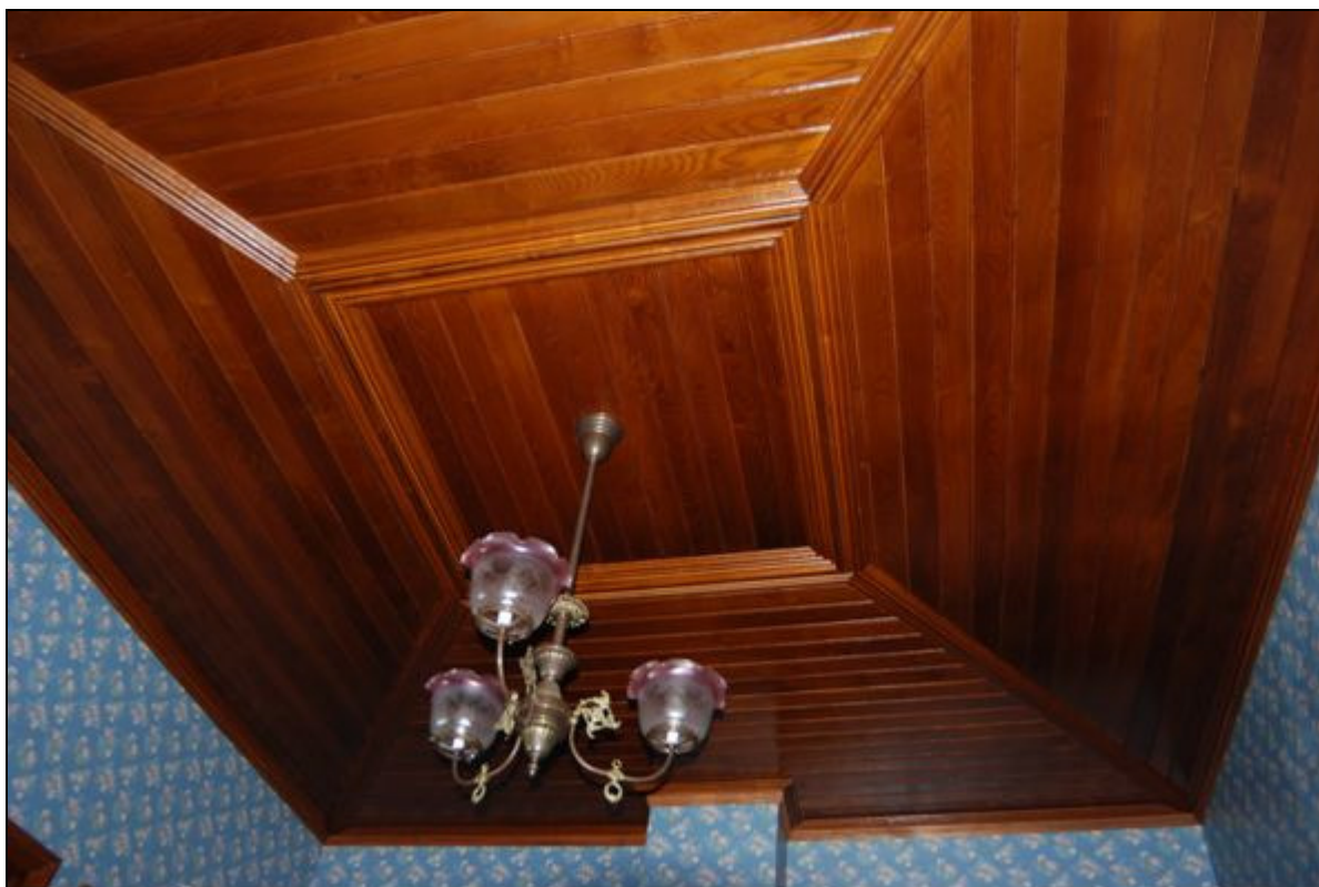
Photo 12 of 14: Wood ceiling detail.
