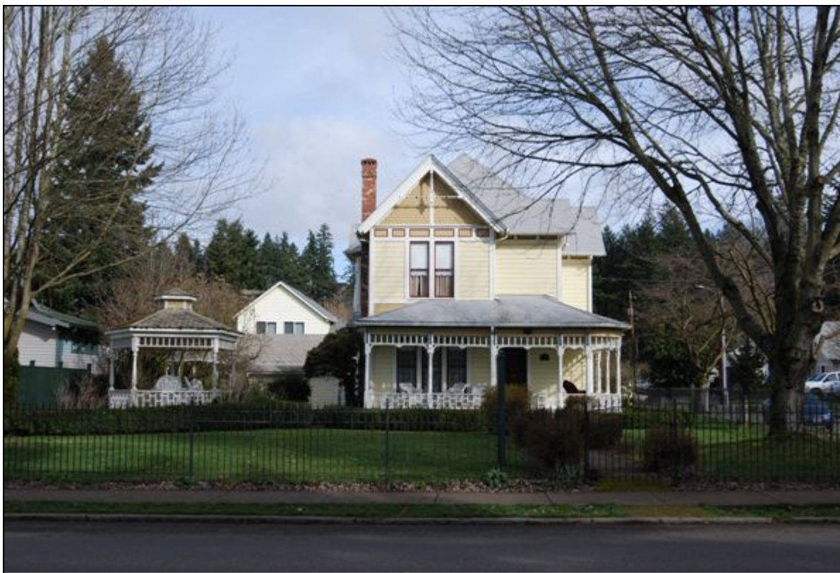
Photo 1 of 14: Southwest elevation of house, gazebo and garage visible. View to the northeast.
