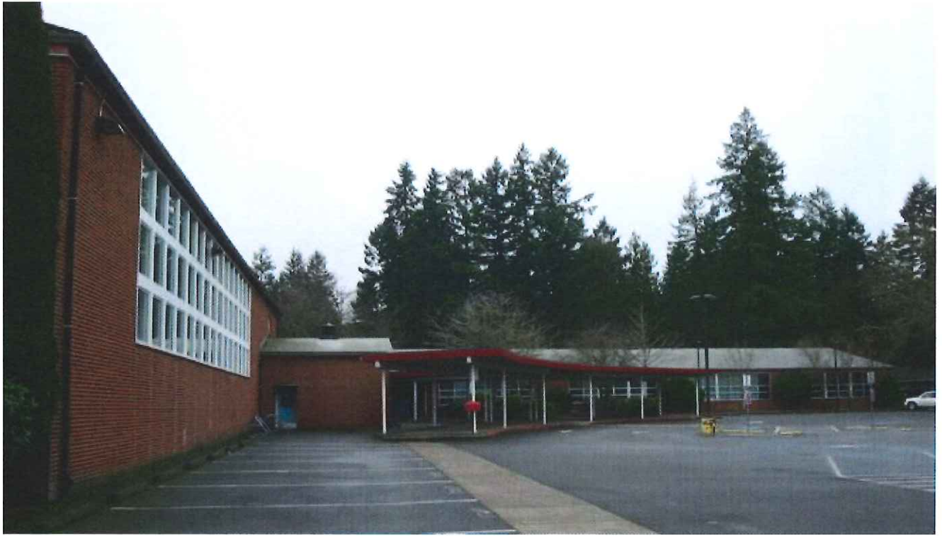
View: Looking west at 1954 north end addition; gymnasium/auditorium at left.
