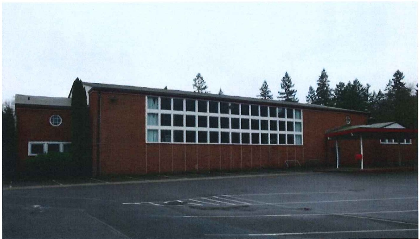
View: North side of gymnasium/auditorium, looking south.
