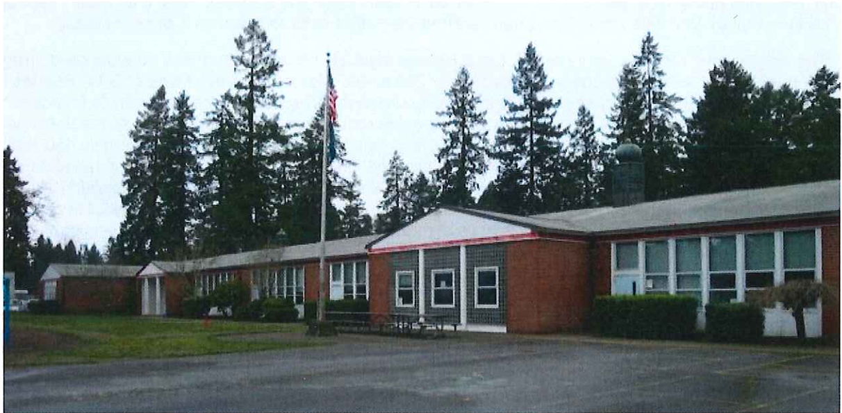
View of front (east) elevation.
