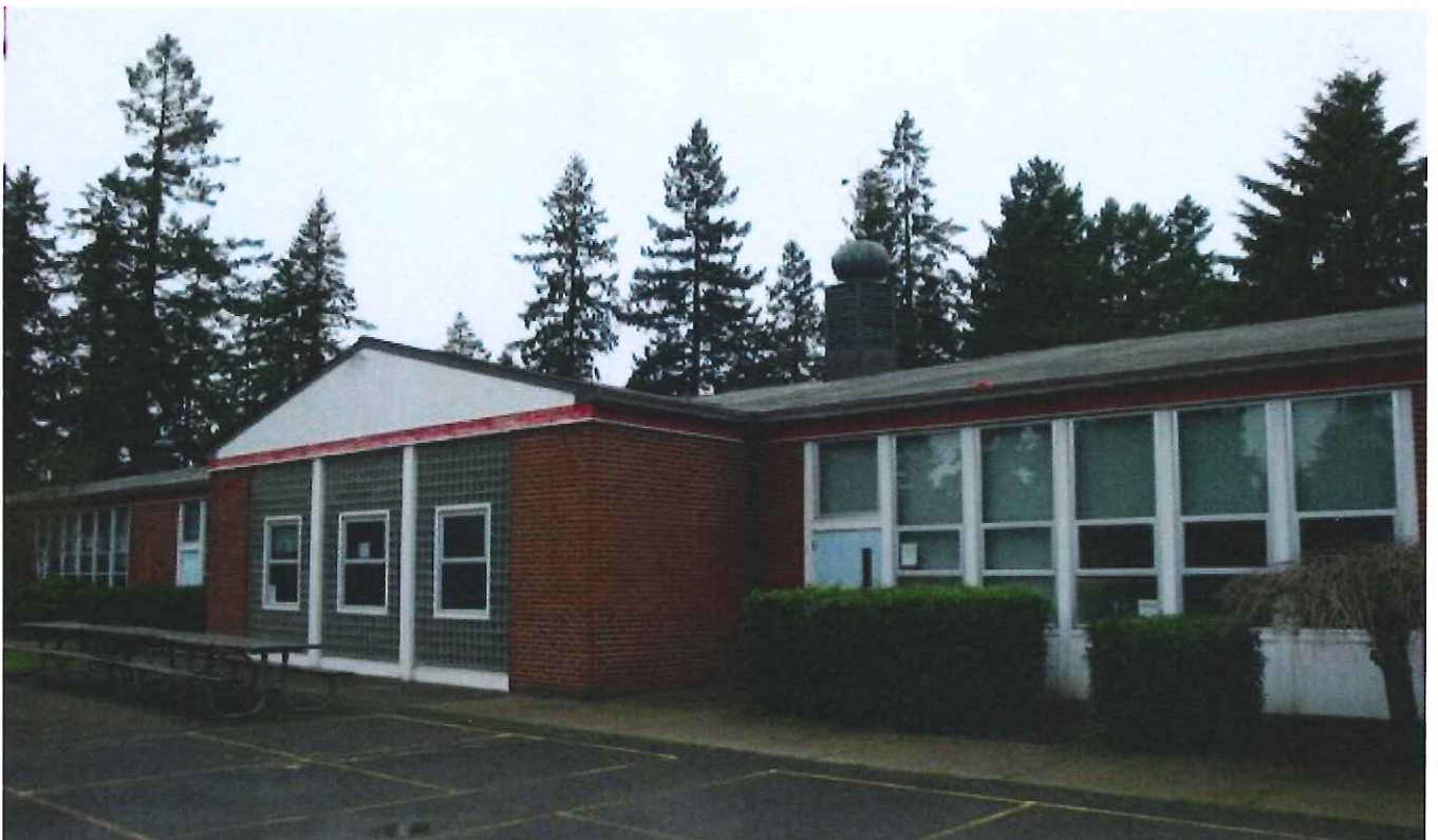
View: East elevation detail, view looking northwest.
