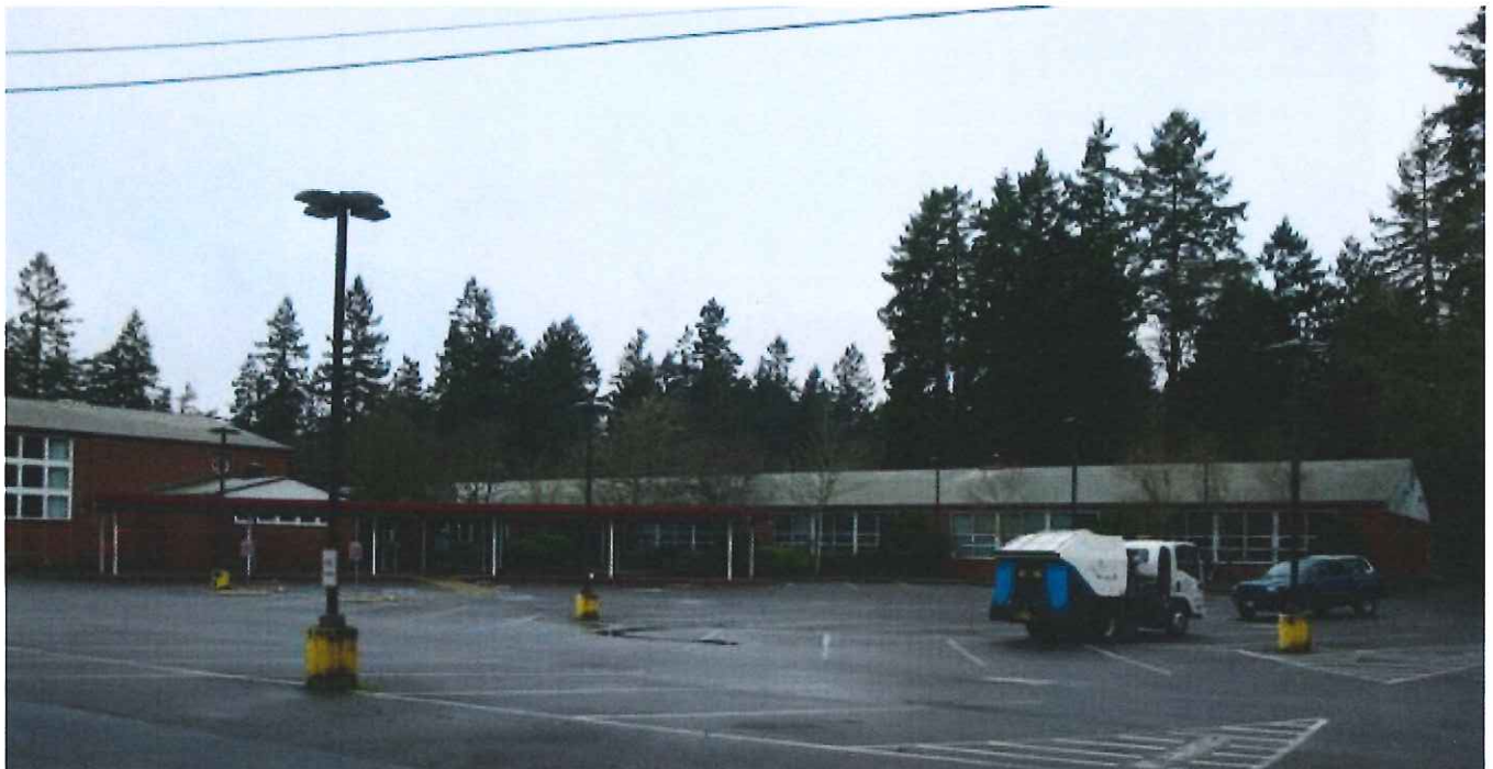
View: 1954 addition to north end of school complex, looking west.
