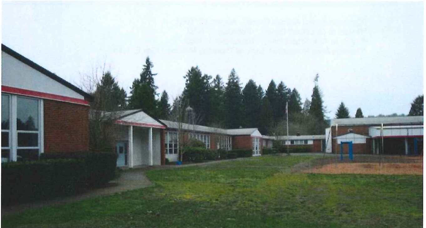
View: East elevation with classrooms along left and gymnasium/auditorium to right, looking north.
