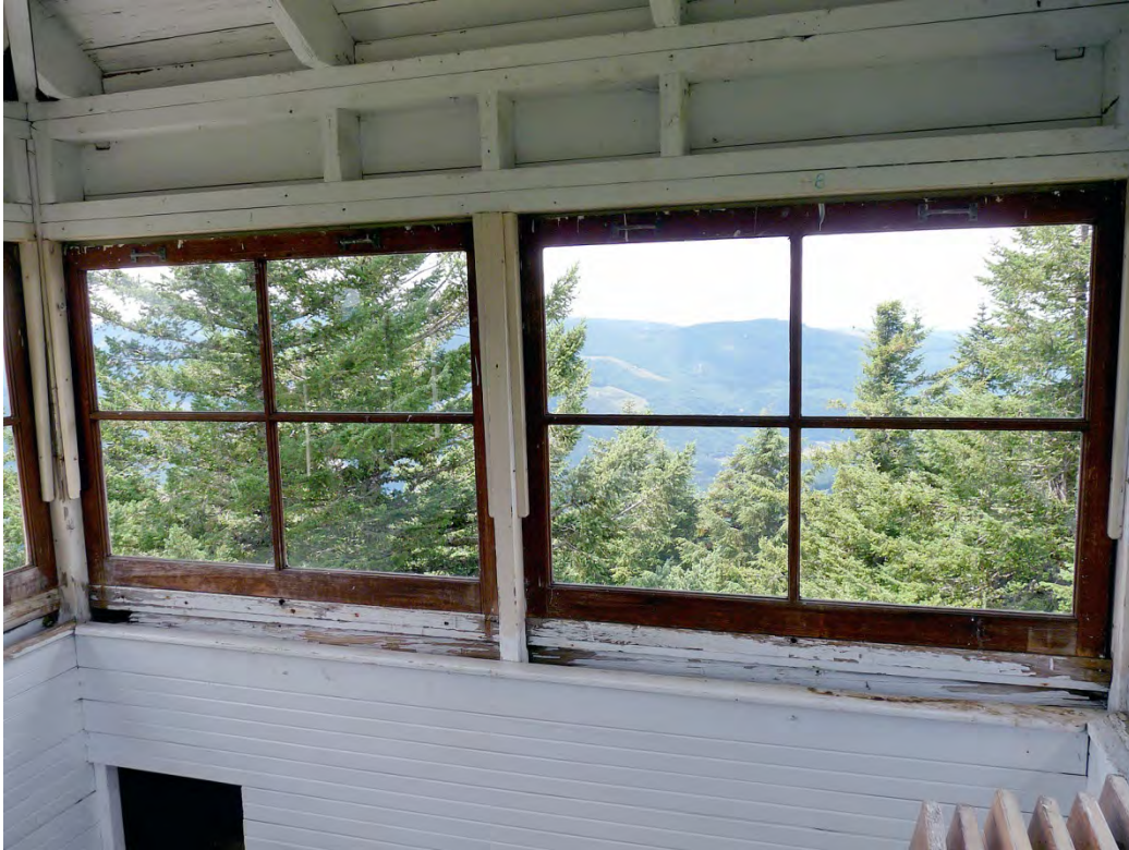
Figure 10. View of the windows in the cupola and the slot in the wall under the sill where the windows are lowered and stored when opened.
