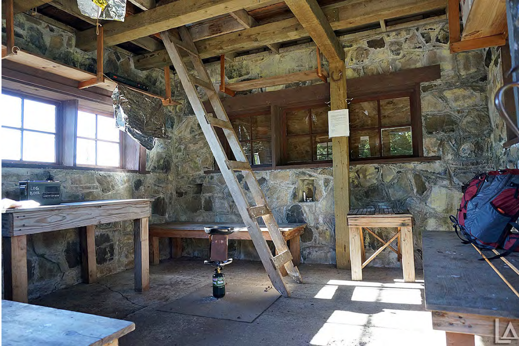
Figure 8. View from the entry door of the inside of the lower story of Pechuck Lookout.
