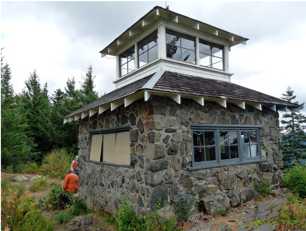
Figure 9. View to the southeast of the back of Pechuck Lookout showing the shutters on the windows on the north wall.
