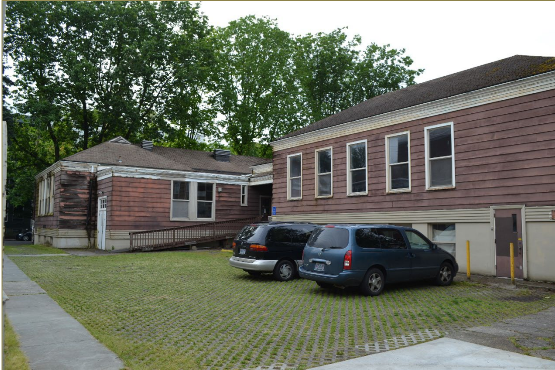
Photo 20. The north (rear) elevation of the St. Francis School and adjacent parking area, viewed towards the southeast.
