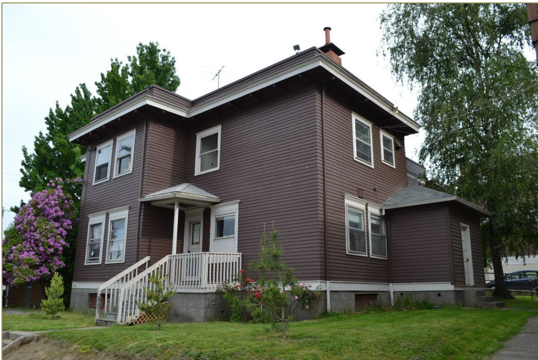
Photo 18. The south and east elevations for the Rectory, viewed towards the northwest.
