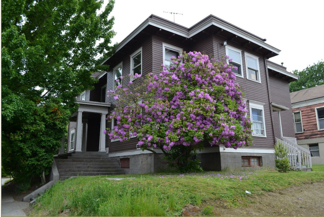
Photo 17. The west façade and south elevation of the Rectory, viewed towards the northeast.
