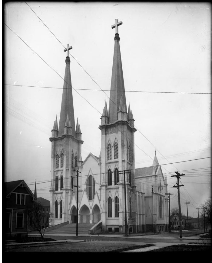
Photo 6. East (primary) and north elevations of the church, likely captured during construction in 1910. The view is facing southwest. Oregon Historical Society Research Library, Photo File #1768-1779, Folder 1770.
