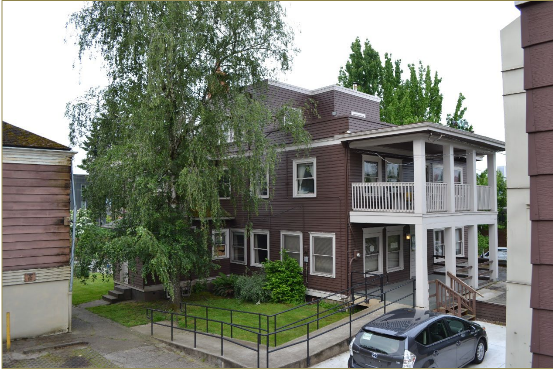
Photo 15. The west (rear) and north elevations of the Rectory, facing southwest.
