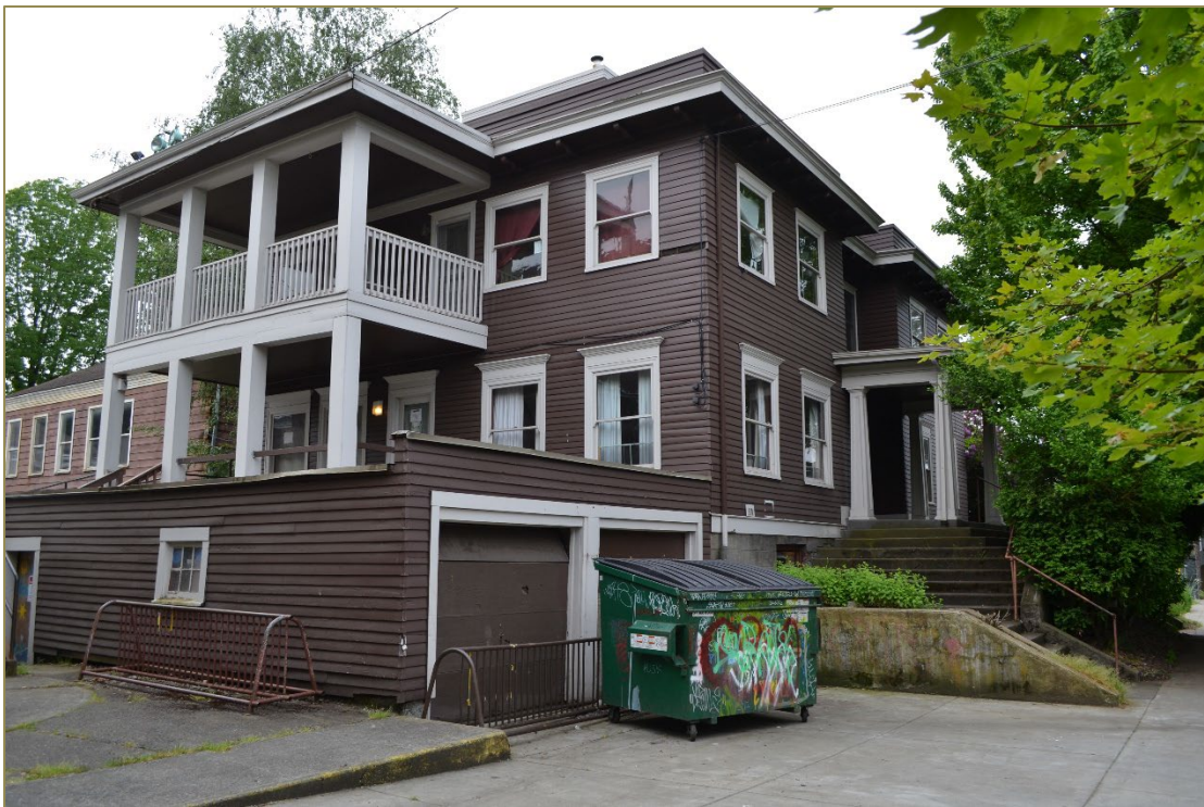
Photo 16. The north elevation and west façade of the Rectory, viewed towards the southeast.
