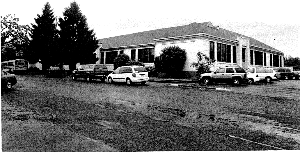
View: Clackamas Elementary School. The 1939 portion is visible at center, the 1947 north wing is at right. The view is to the southwest.
