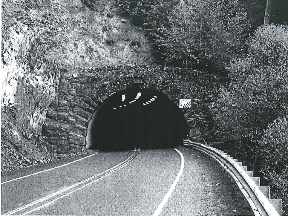
Salt Creek Tunnel, west portal.
