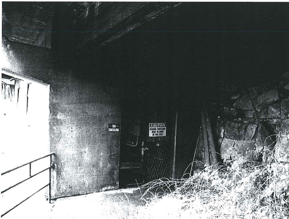
Powerhouse, view from southeast.
