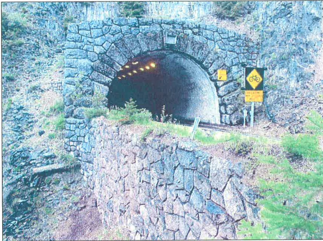
Figure 3: East side rock portal face and retaining wall
