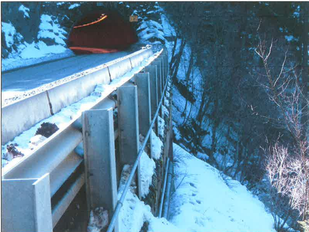
Figure 6: West side viaduct with "W" bridge rail (added in 1995)
