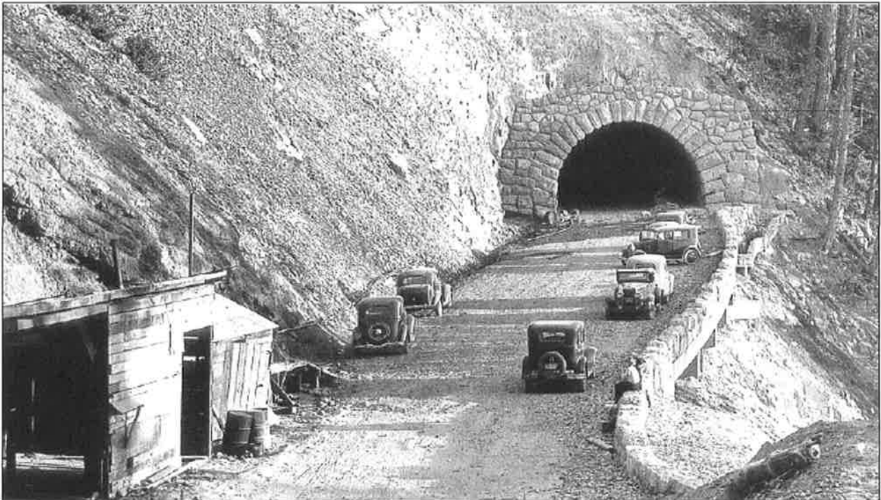
Figure 2b: East side Salt Creek Tunnel during construction 1938
