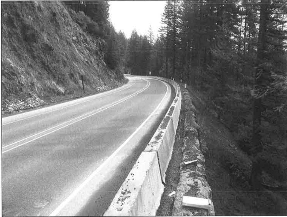
Figure 11: Masonry bridge rail, through the build up of volcanic rock during the snowy season, is nearly buried, aside from being masked to traveling public by requisite bridge rail for safety
