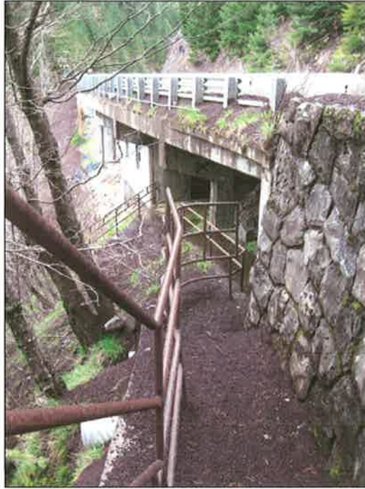
Figure 5: Modified tube pedestrian rail at west side viaduct
