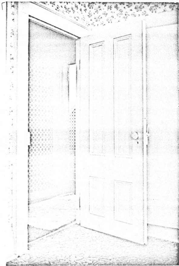
4-panel door, upstairs bedroom.
