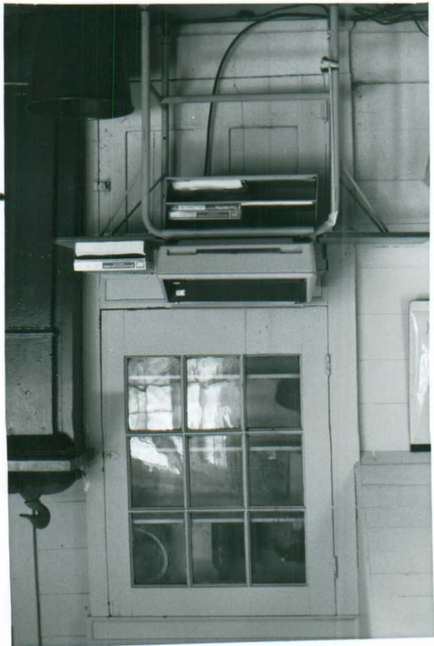
Fiechter (gann) House: Built-in cupboard, South Parlor
